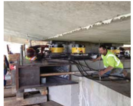
Installation and stressing of pier compression collars prior to jacking.
