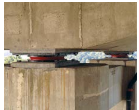
Completed disc bearing.
