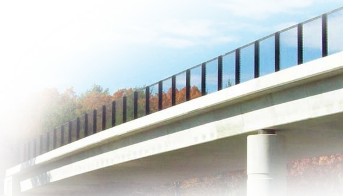
Photo Courtesy of MassDOT (Massachusetts Department of Transportation)
