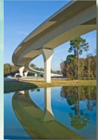
I-95/I-295 North Interchange (Photo Courtesy of Ray Stanyard Photographer)
