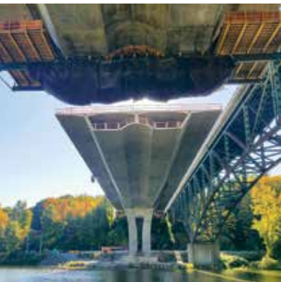
Photo Courtesy of FIGG
