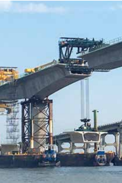
Photo Courtesy of PCL Civil Constructors, Inc.
