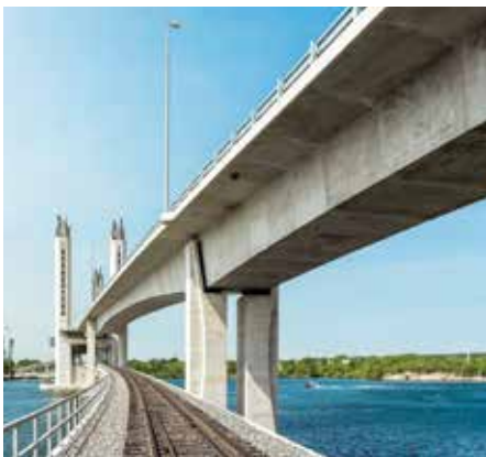
Photo Courtesy of FIGG
