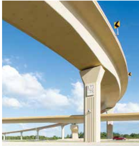
Photo Courtesy of PCL Civil Constructors, Inc.
