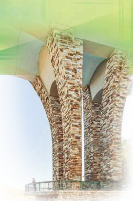
Photo Courtesy of FIGG
