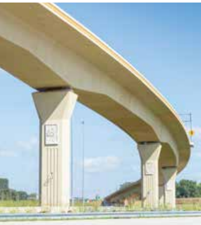
Photos Courtesy of PCL Civil Constructors, Inc.
