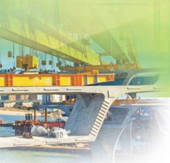
Photo Courtesy of FIGG
