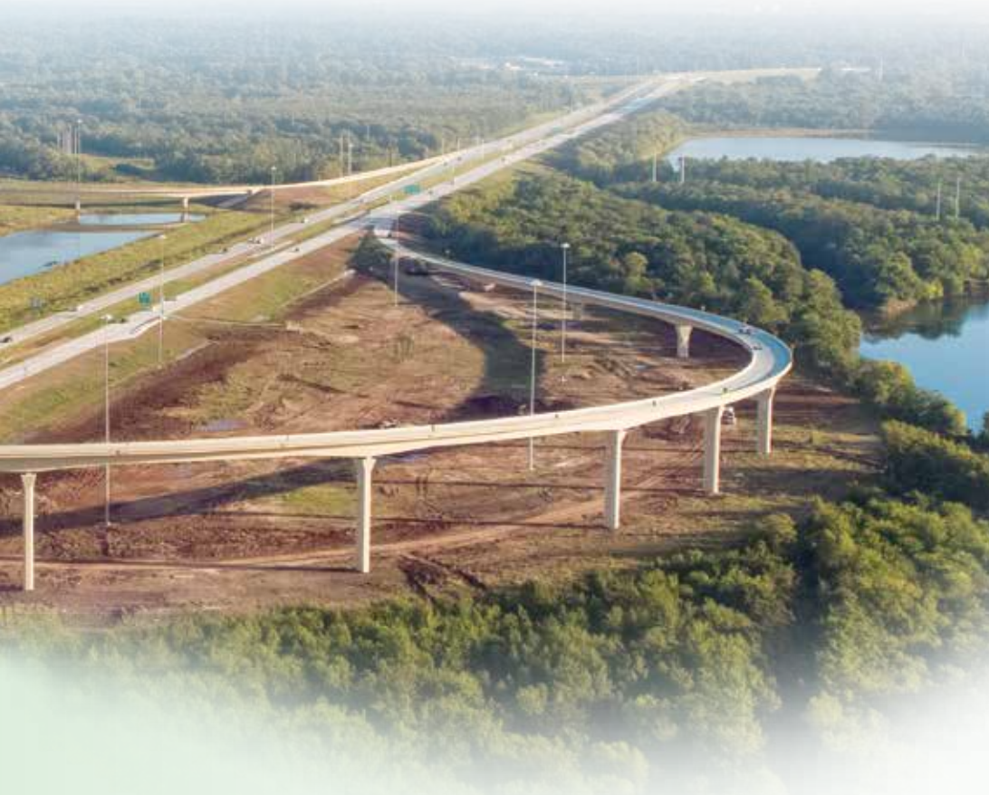
Photo Courtesy of PCL Civil Constructors, Inc.
