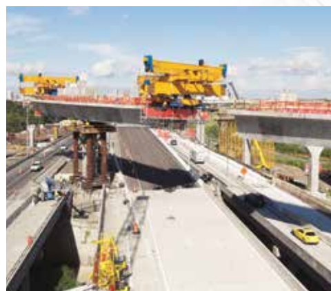
Photo Courtesy of PCL Constructors, Inc.
