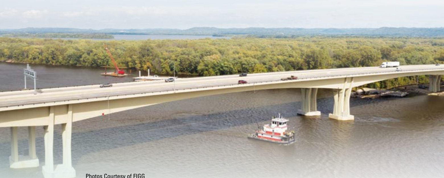
Photos Courtesy of FIGG
