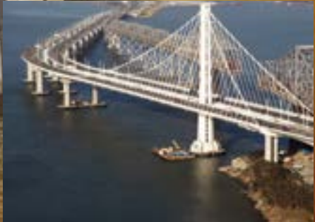
San Francisco-Oakland Bay Bridge, California Photos Courtesy of T.Y. Lin International
