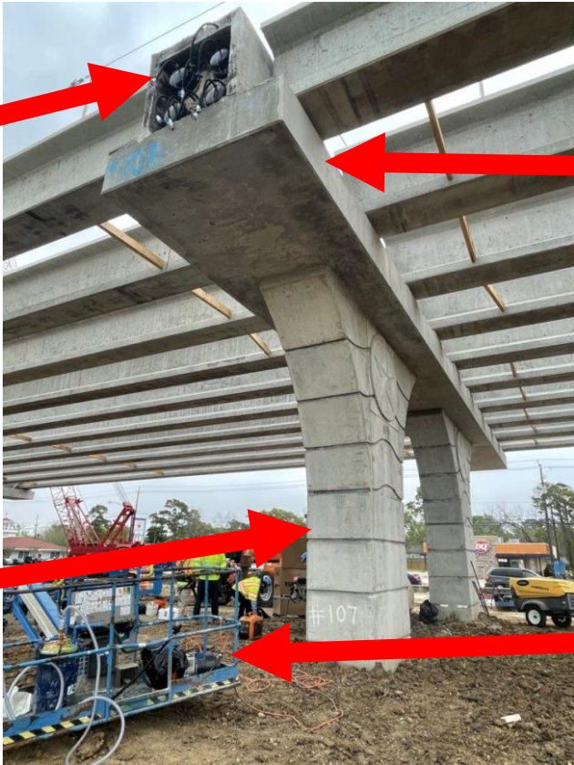
Post-tensioned Bent Cap
