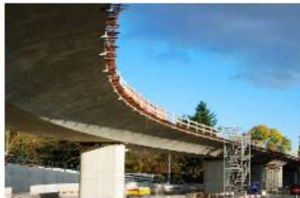
Lect Viaduct, Geneva, Switzerland - 2009
