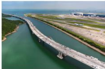
Hong Kong - Zhuhai Macau Bridge, Hong Kong - 2017
