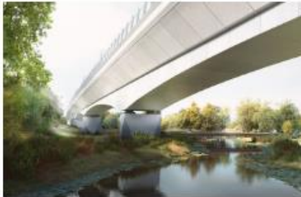
United Kingdom - HS2 - Colne Valley Viaduct 2022
