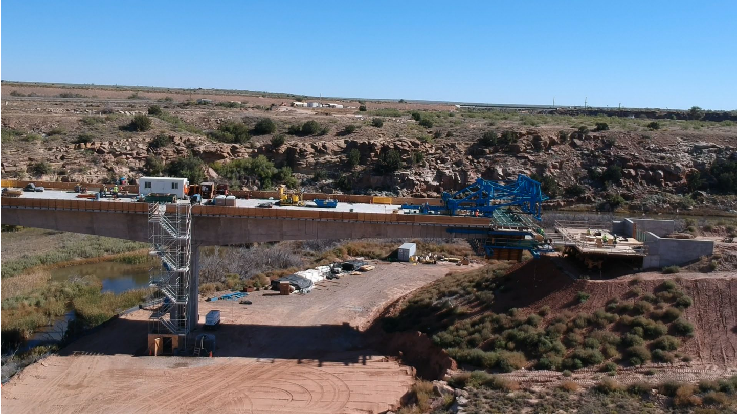
New Mexico's First Cast-In-Place Segmental Bridge
