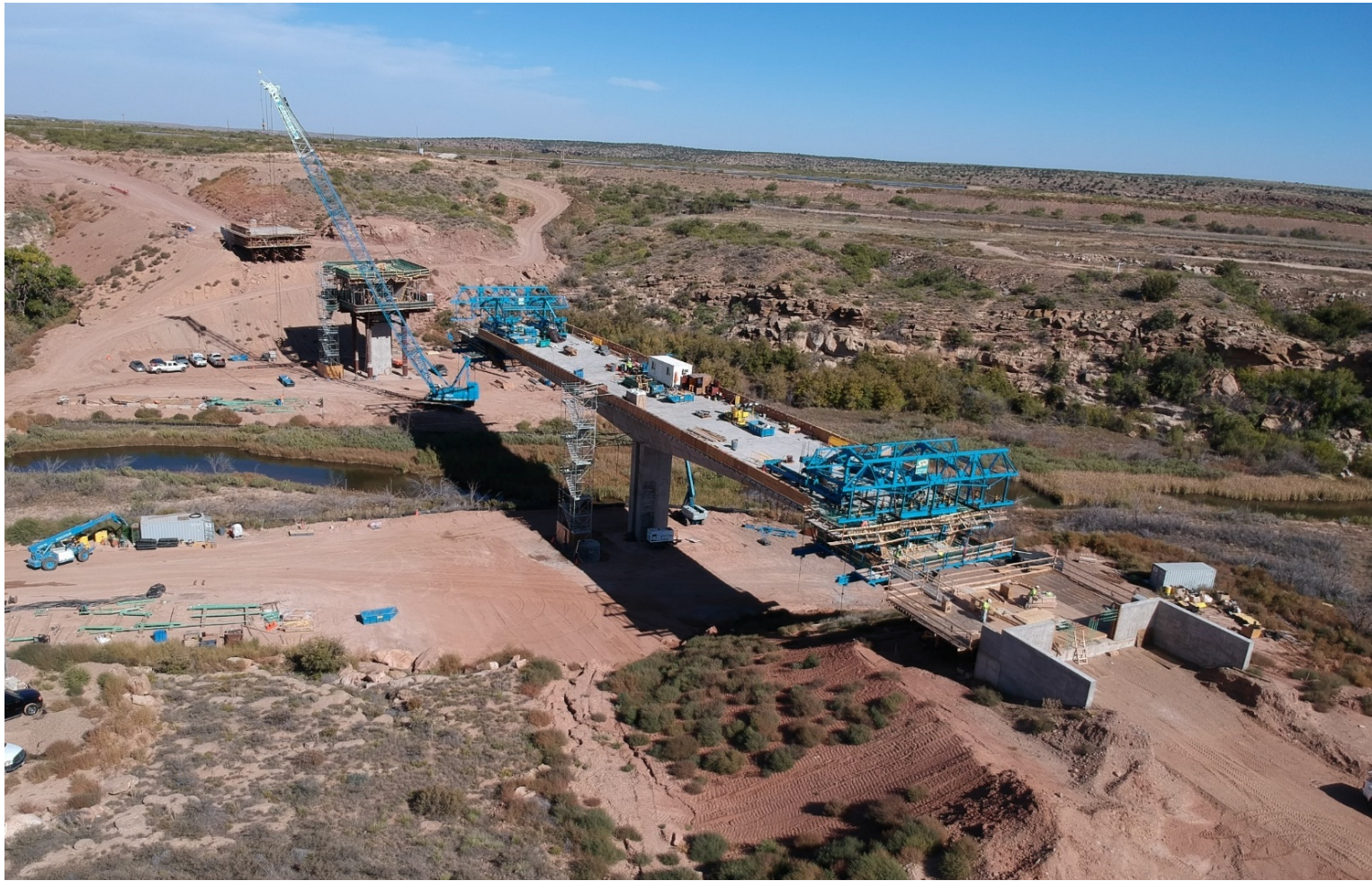
Construction of Pier Table 2 during the casting of Cantilever 1
