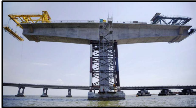
Precast Balanced Cantilever, Bonner Bridge, NC (Courtesy of RS&H)
