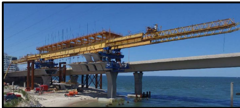
Precast Span-by Span, Lesner Bridge, VA (Courtesy RS&H)
