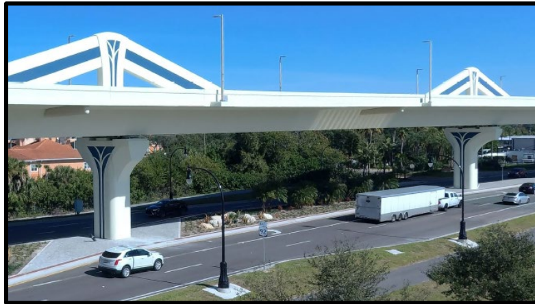
Precast Finback Bridge, Selmon West Extension, Tampa, FL (Photo Courtesy of Sarah Lesch)
