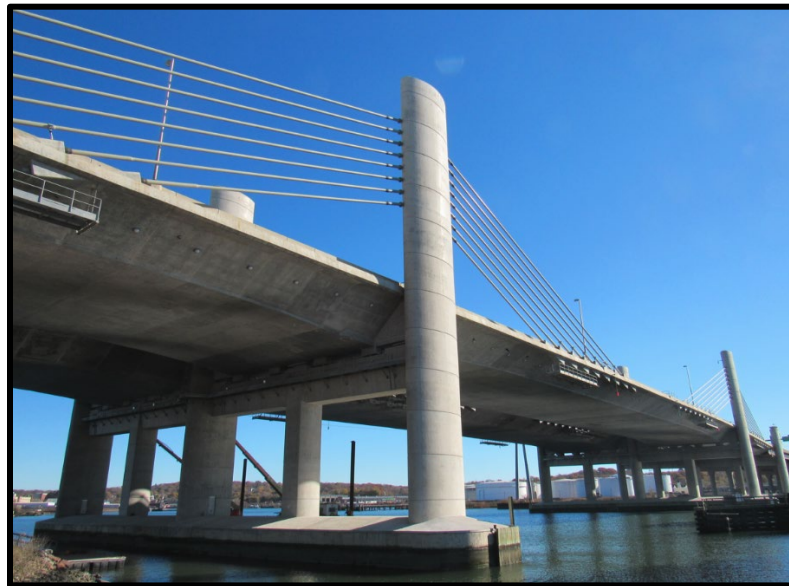
Extradosed Bridge, Pearl Harbor Memorial Bridge, in New Haven, CT (Photo Courtesy of Connecticut Department of Transportation)
