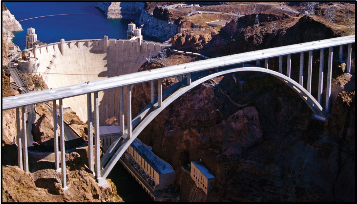
Precast Segmental Arch Bridge, O'Callaghan-Tillman Memorial Bridge Clark County, NV & Mohave County AZ (Photo Courtesy of FHWA)
