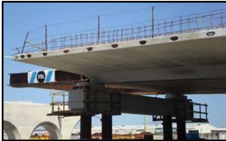
Incremental Launch, Belliare Beach Bridge, FL (Photo Courtesy of VSL)
