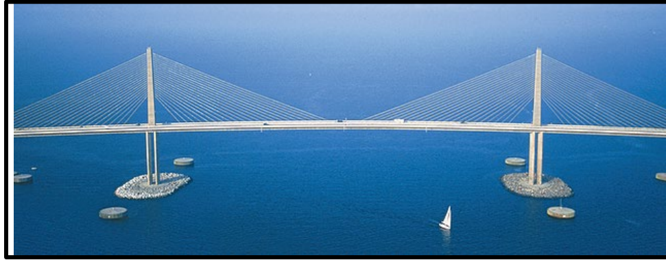
Concrete Segmental Cable-Stayed Bridge, Sunshine Skyway Bridge, FL (Photo Courtesy of FIGG Engineering Group)
