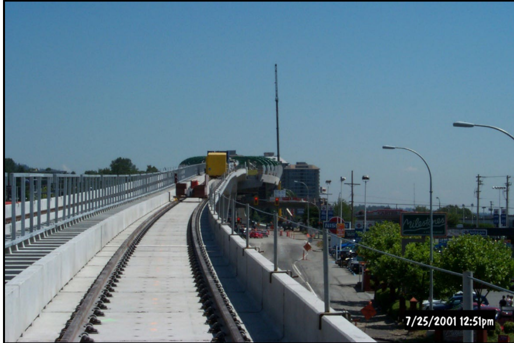
Figure 4-36. Plinthless Rail Attachment on Vancouver Rapid Transit in Vancouver, Canada (Photo Courtesy of SYSTRA IBT)
