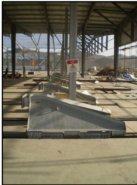
Figure 4-34. Elevation View of Friction Buffer Stop (Photo Courtesy of SYSTRA IBT)
