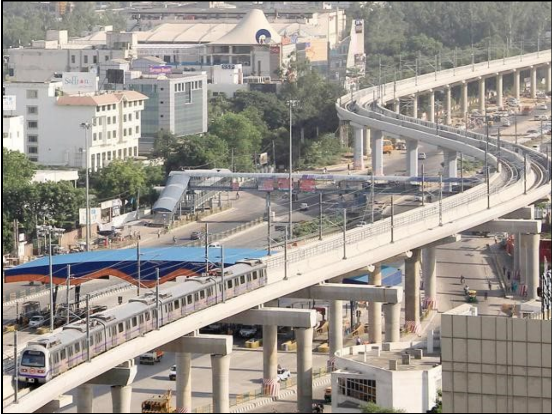
Figure 4-24. Chorded, Full-Span U-Girders in a Curve in Faridabad, India (Photo Courtesy of SYSTRA IBT)
