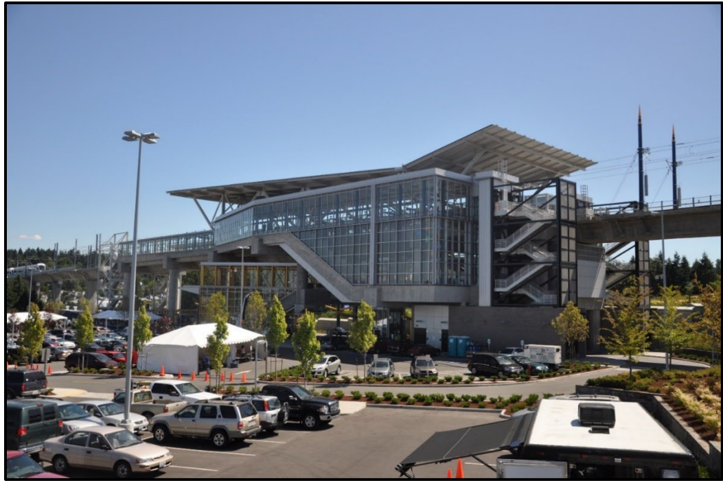
Figure 4-5. Station Structure for Sound Transit in Seattle, WA Independent of Box Girder Guideways at Each End (Photo Courtesy of SYSTRA IBT)
