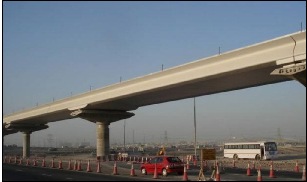
Figure 4-11. U-Section Guideway for Dubai Metro in the United Arab Emirates (Photo Courtesy of SYSTRA IBT)
