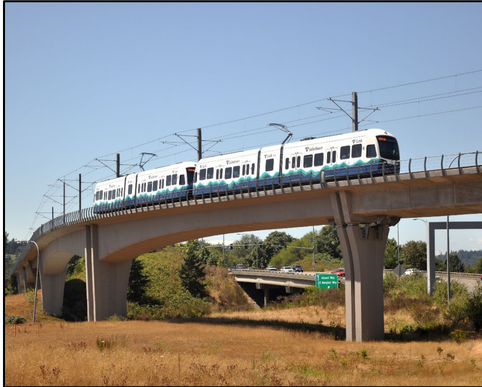
Figure 5-2. Active Trains Can Present Challenges for In-Service Inspection Sound Transit Line in Action (Photo Courtesy of ASBI)
