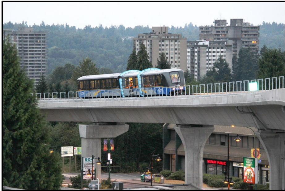
Figure 4-22. Test Run of Train with Clearance Envelope on Evergreen Line in Vancouver, Canada (Photo Courtesy of SYSTRA IBT)
