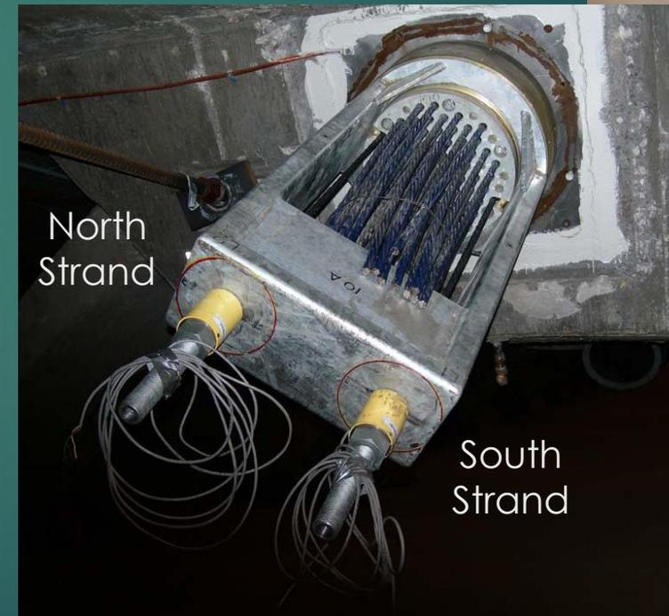
Completed carbon fiber anchor chair without permanent cap
