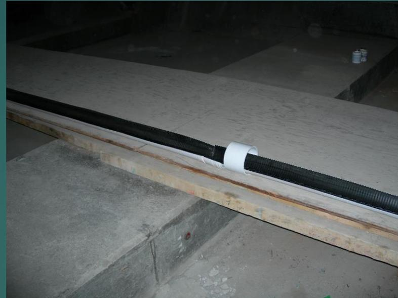
Tray to protect carbon strand during installation
