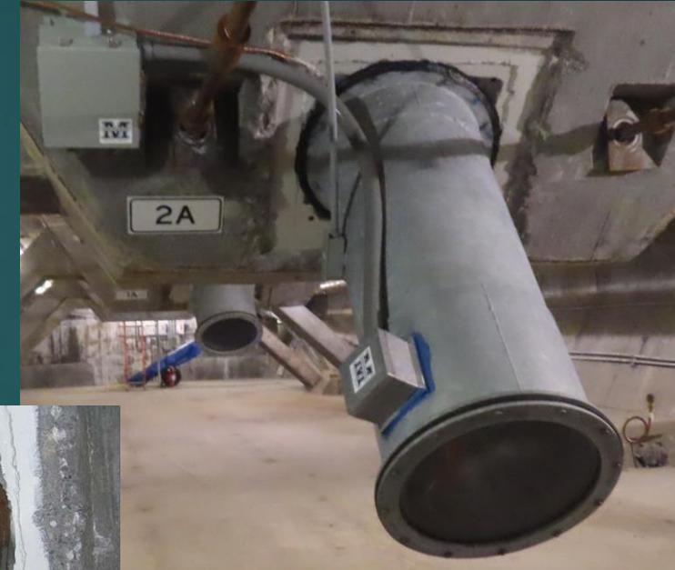
Carbon fiber anchor with permanent cap (note see-through end cap)
