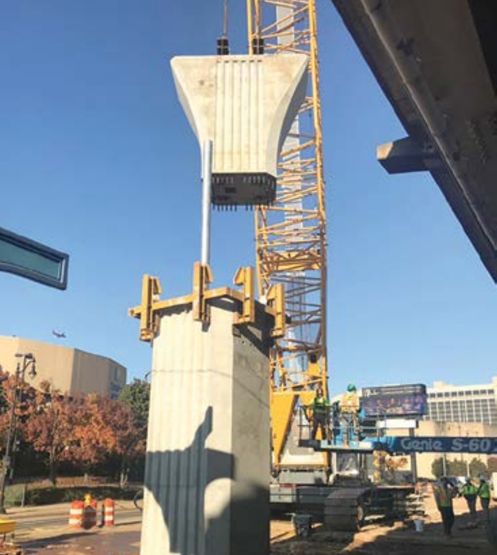
A precast concrete pier cap with fluted aesthetic detailing is erected on a column element. Segments are connected using grouted couplers. Photo: Volkert Inc.
