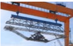
Flying a completed rebar cage to the long-line mold.
