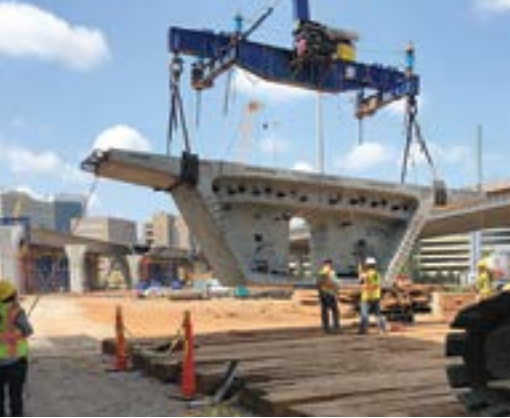
The erection of a split-pier segment. Photo: Structural Technologies.
