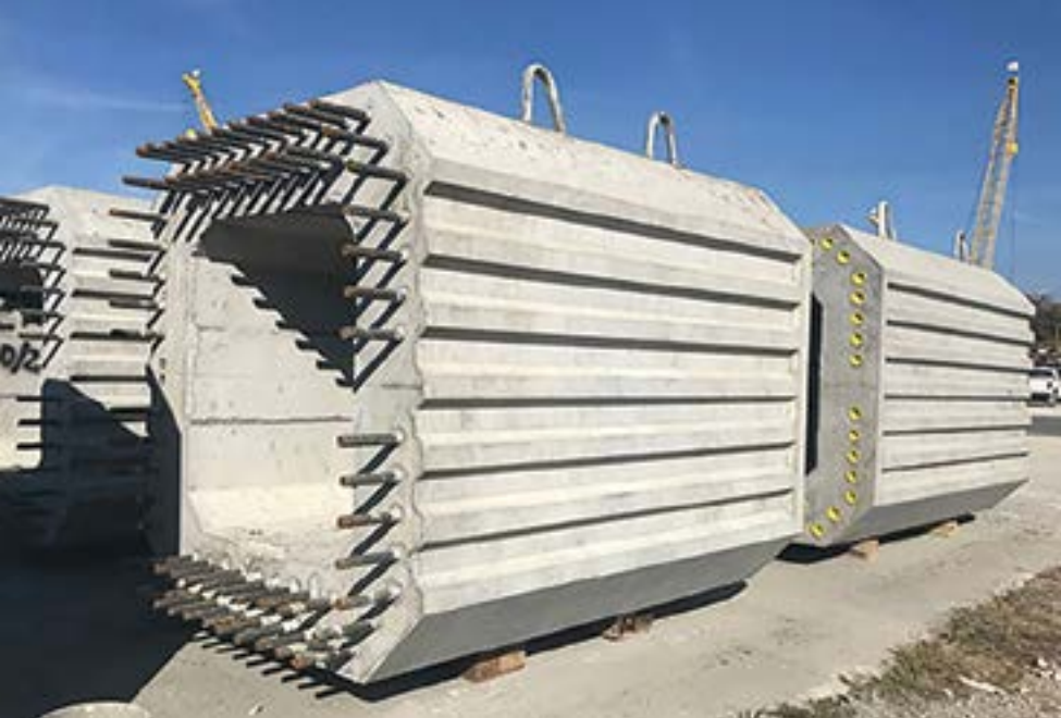
Precast concrete column segments in storage. Note the extended column reinforcement and grout sleeves that are visible on the ends of the segments. Photo: Johnson Bros.
