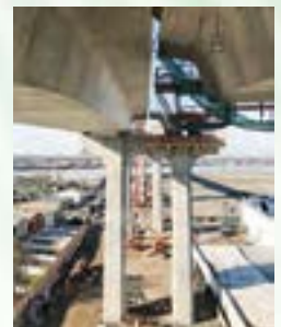
I-91 Brattleboro Bridge Photo Courtesy of Richard Tremblay
