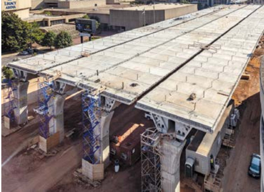
A typical span after erection of the four lines of box-girder segments. A longitudinal closure pour about 3 ft 6 in. in width was used to join the segments for each of the two bridges. The completed eastbound and westbound structures are separated by a 6 in. gap. Photo: Volkert Inc.
