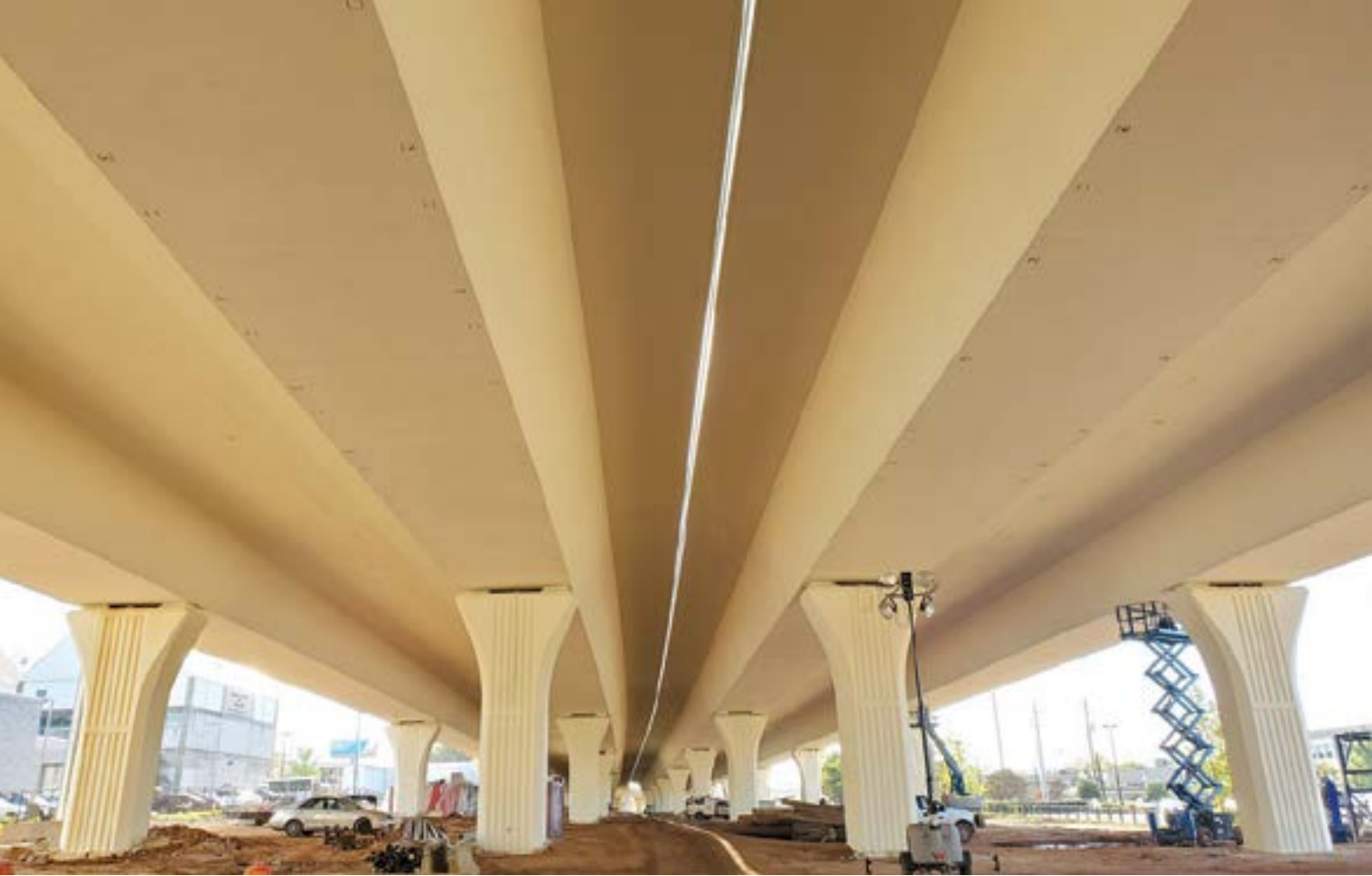
The area beneath the completed mainline spans after painting. City officials intend to use this area for public events. Photo: Johnson Bros.
