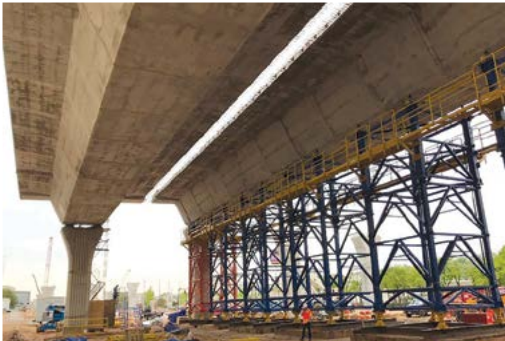
Falsework towers were used to support segments during erection. Photo: Volkert Inc.
