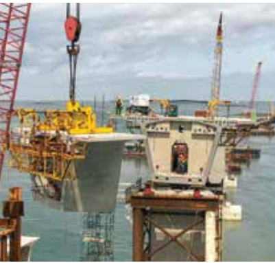
Photos courtesy of PCL.
