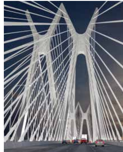
Projected growth in traffic to almost triple what it is today demanded an increase in travel lanes from 2 to 4 in each direction with full 10-foot shoulders and keep the new bridge in existing right of way. Nighttime rendering of the New Ship Channel Bridge. (Rendering courtesy of FIGG.)
