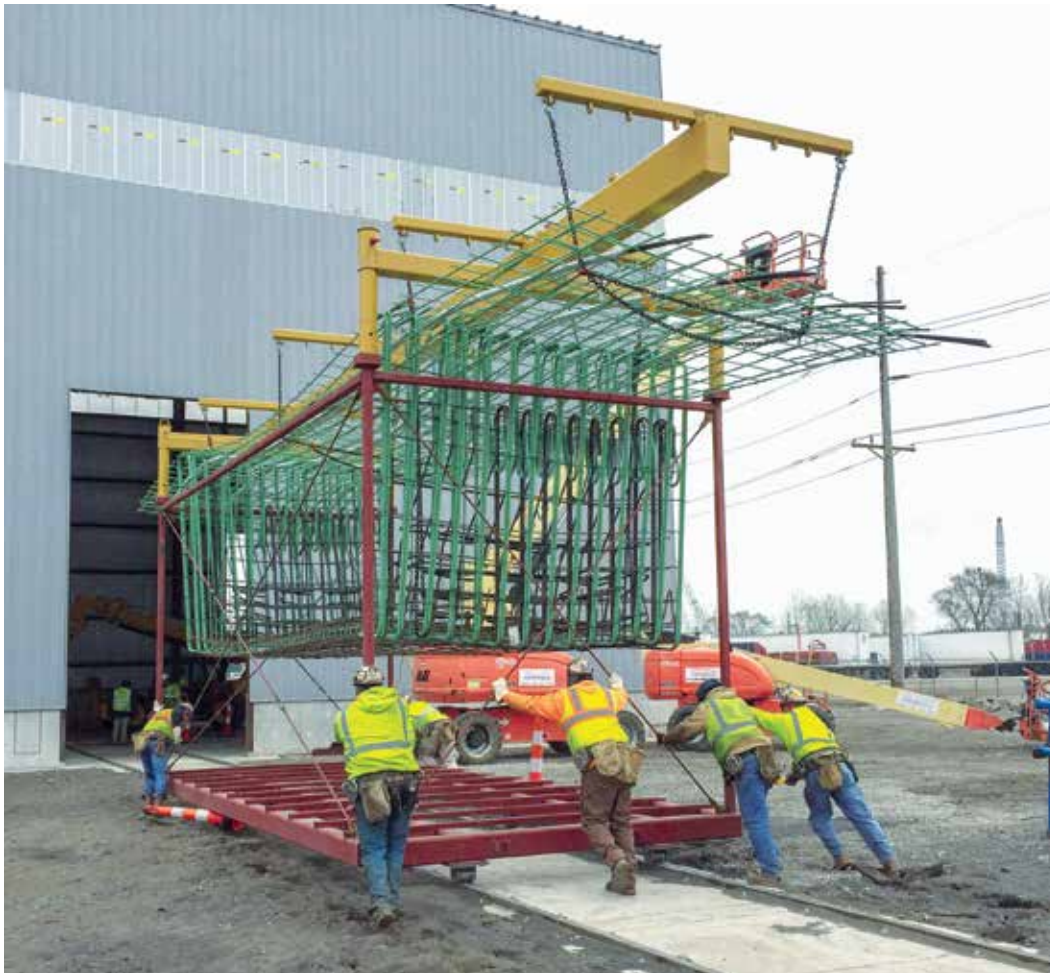
Moving pre-tied typical segment cage on transfer cart, (Photo courtesy of FIGG)
