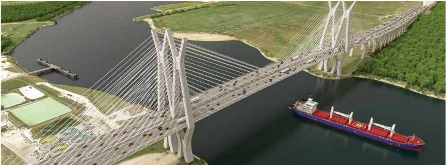
Rendering of the new concrete segmental cable-stayed Ship Channel Bridge carrying the Sam Houston Tollway (East), featuring a 1,320-foot main span over the Houston Ship Channel. (Rendering courtesy of FIGG.)
