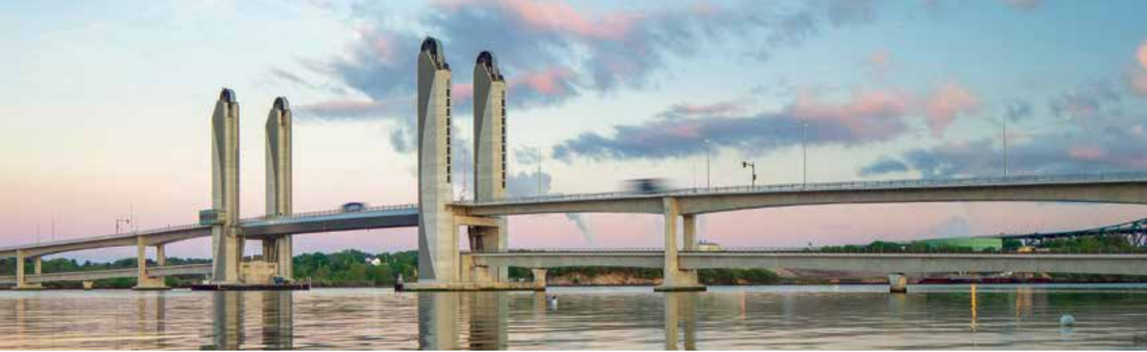
The New Sarah Mildred Long Bridge includes 2,803' of vehicular Bridge and 1,795' of railroad service across the Piscataqua River Built with a precast concrete segmental design. (Photo courtesy of FIGG)
