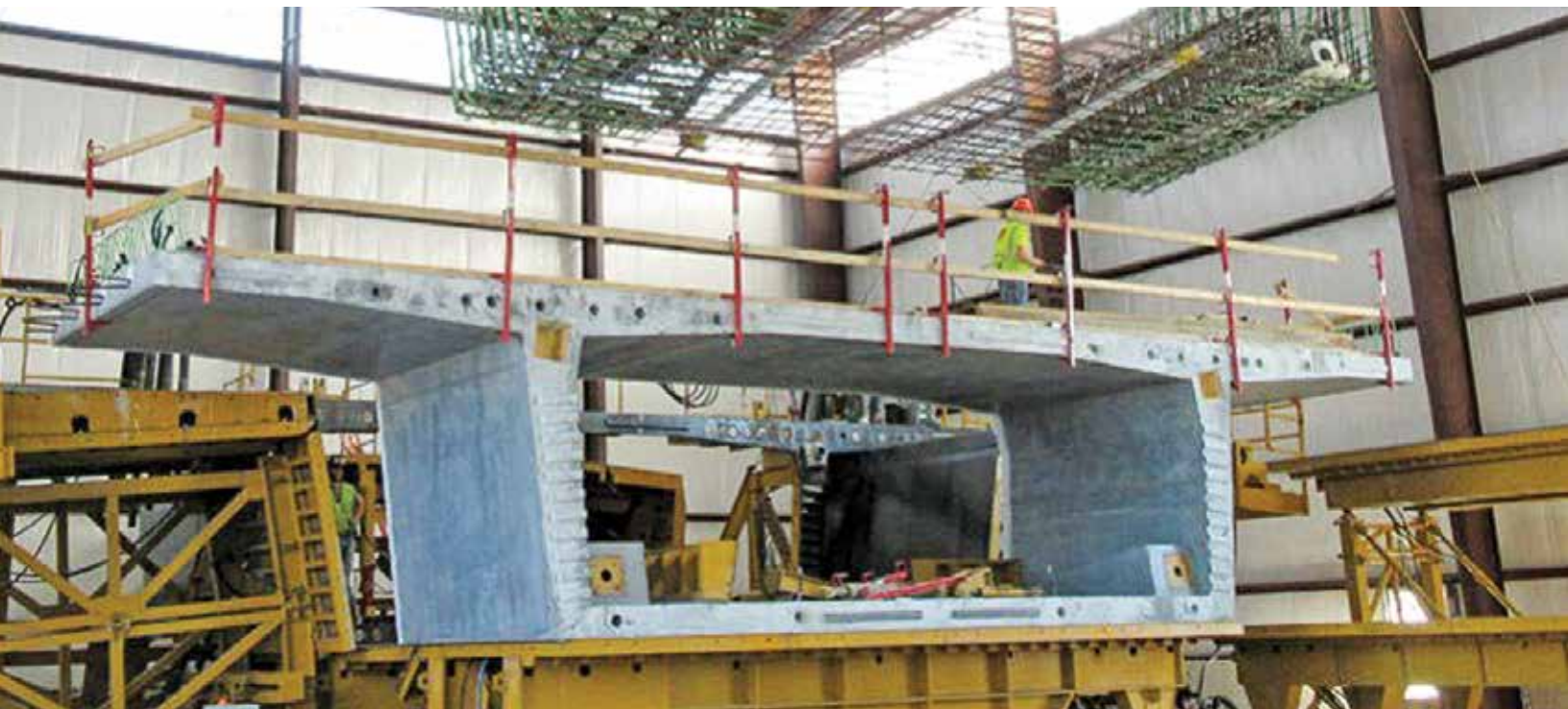
A casting bed inside the precast building is used for constant-depth segment casting. (Photo courtesy of FIGG.)
