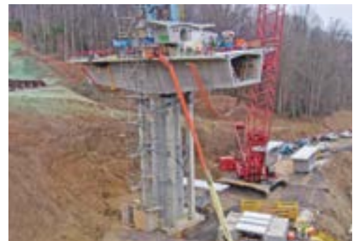
North pier as of December 2022.
