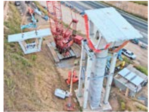
Segments being erected on north pier.
