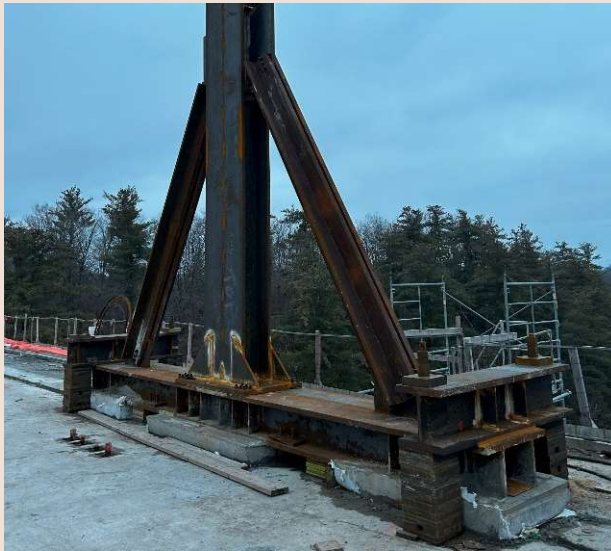
Bracing and base elements of tower
