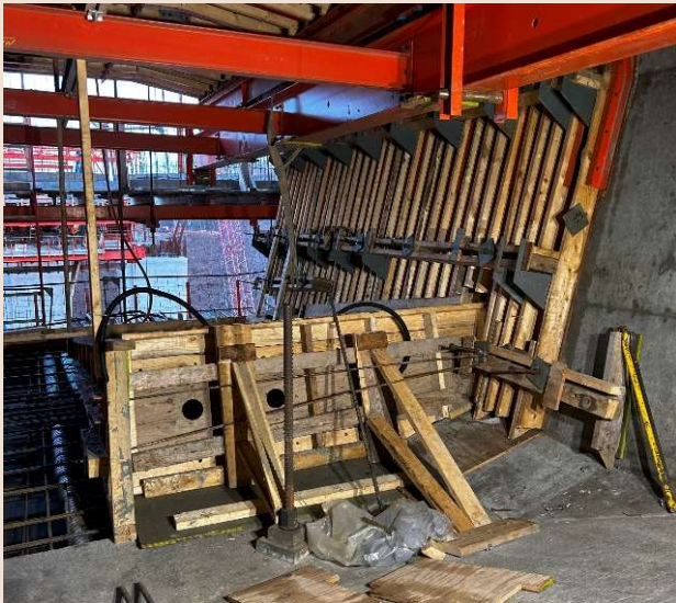
Launch MFT forward and setup formwork
