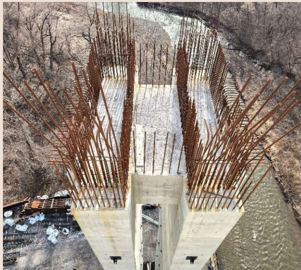
Columns bars extended for Pier Table
