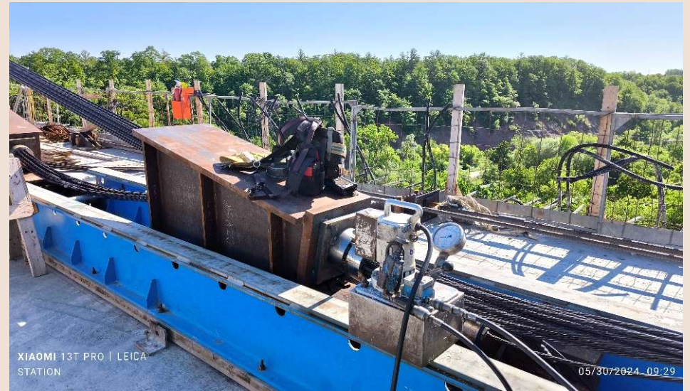
Anchor box fitted between MFT rails
