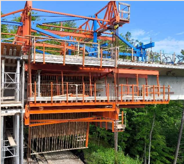
Uni-directional MFT construction
