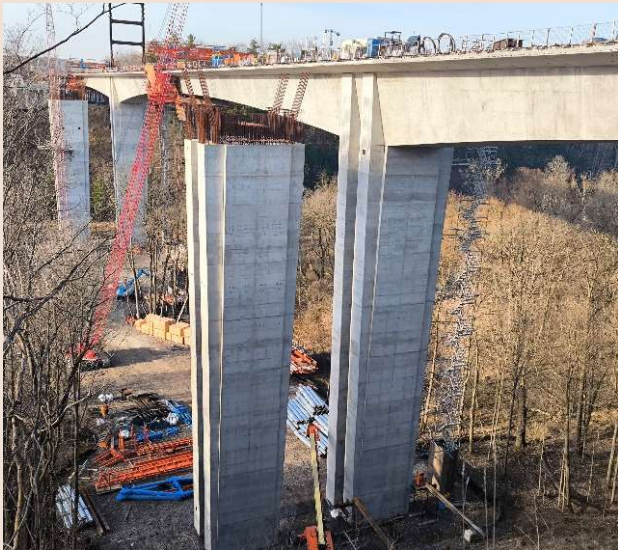
Pier Columns Constructed
