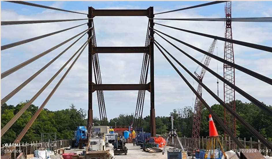
View of stay tower facing away from extended cantilever
