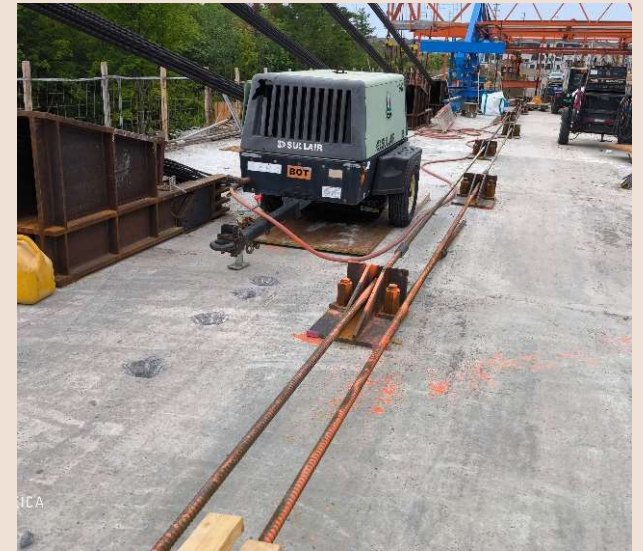
External PT Bars and Brackets
