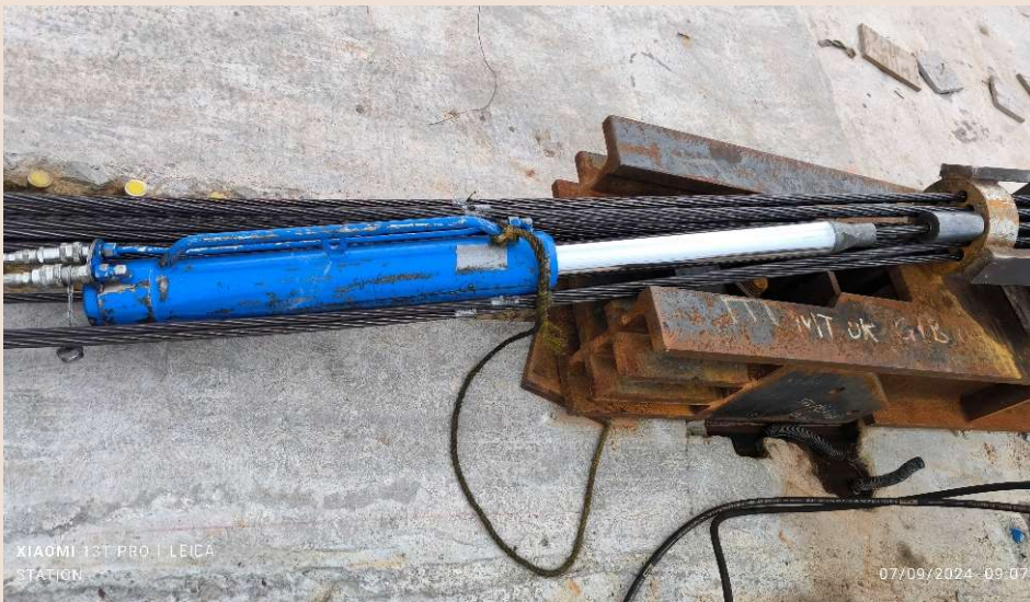
Mono-strand stressing jack fitted on anchor box
