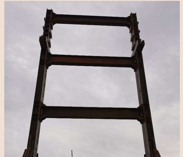
Columns and transverse beams of tower
