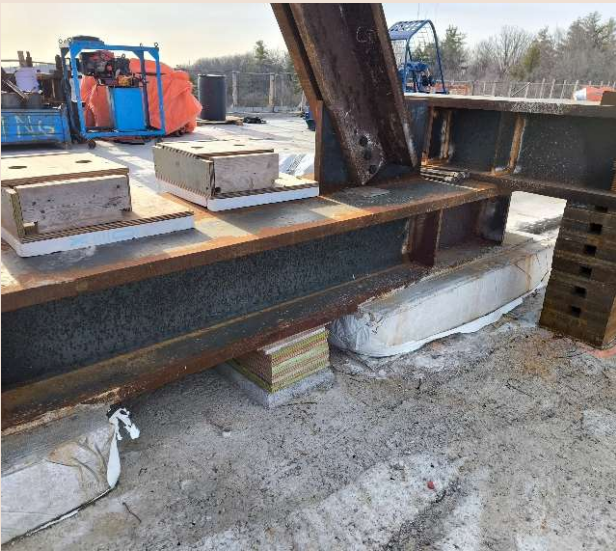
Grout pads & base connection to pier table
