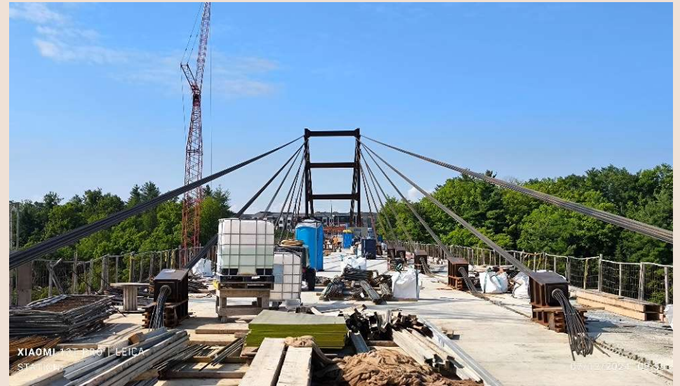
Layout of stay cables along extended cantilever
