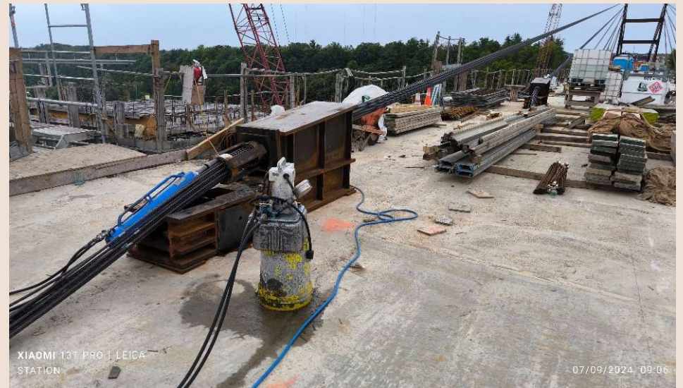
Stay cable path from anchor box to stay tower
