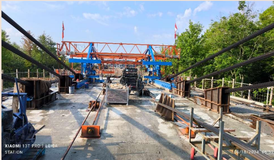
Arrangement on Extended cantilever
