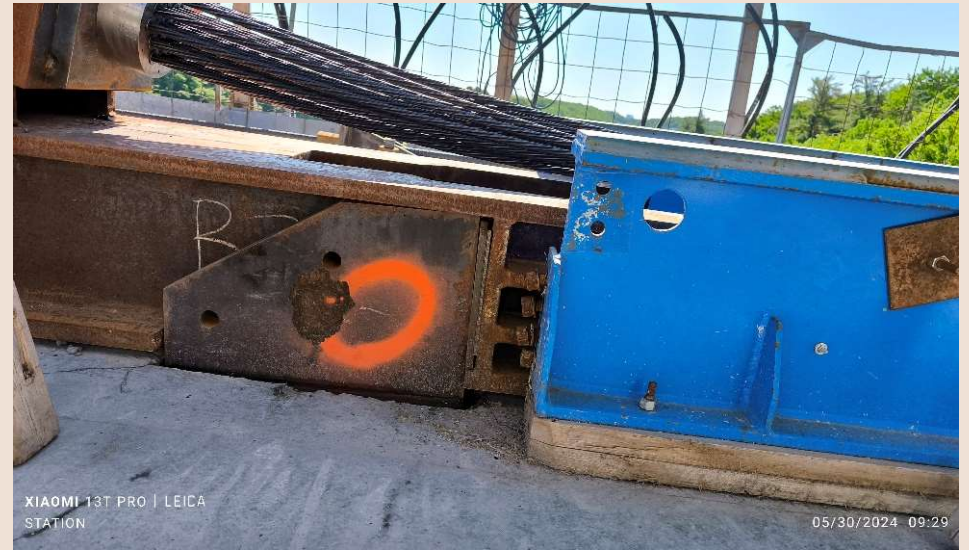
Interface of cast-in lug to anchor box
