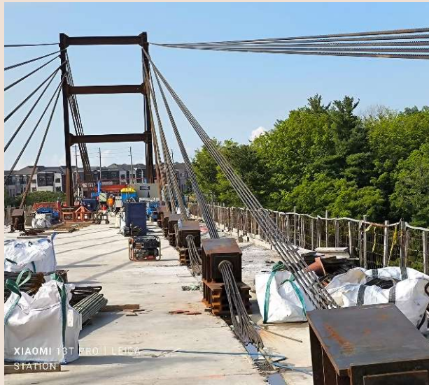
Temporary stay tower and anchors
