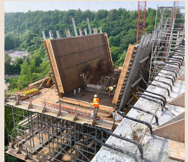
Installation of Formwork
