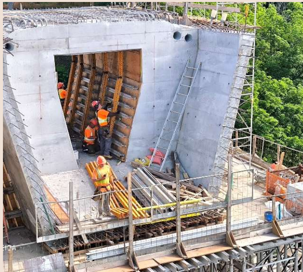
Casting of diaphragms
