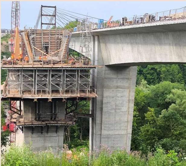
Casting of soffit and webs
