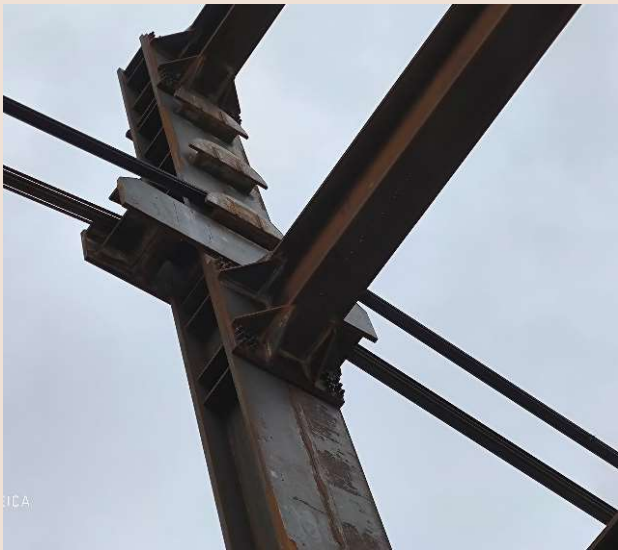
A1/A2 anchor points on tower
