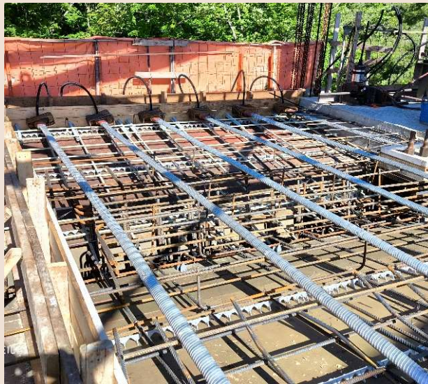
Install rebar, PT, inserts
