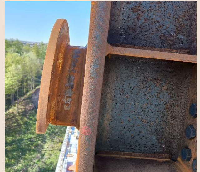
Saddle detail for typical stay
