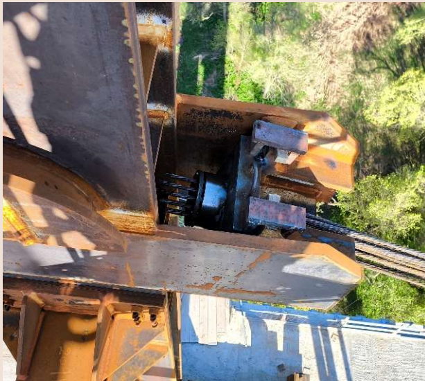
View of anchoring stay cable
