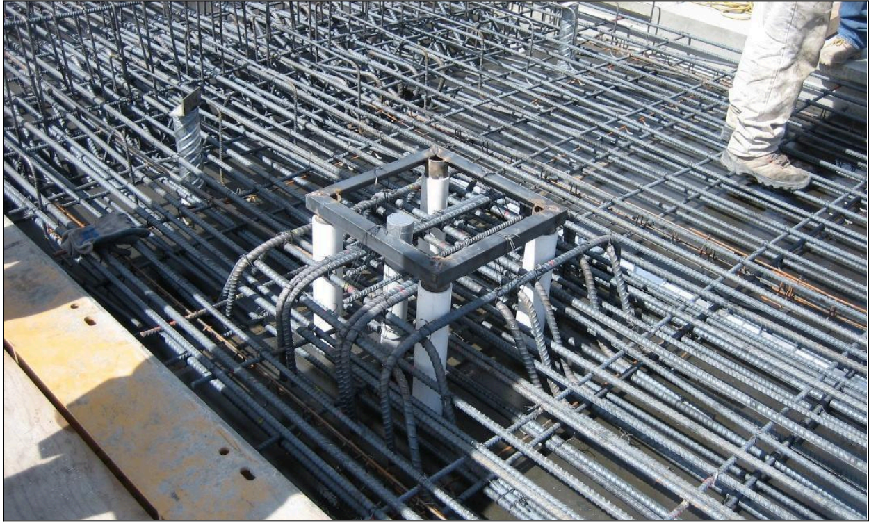
Figure 9.44 – Rebar Added for Center-Mount OCS Pole (Photo Courtesy of Fueled Photography/PCL Civil Constructors, Inc.)
