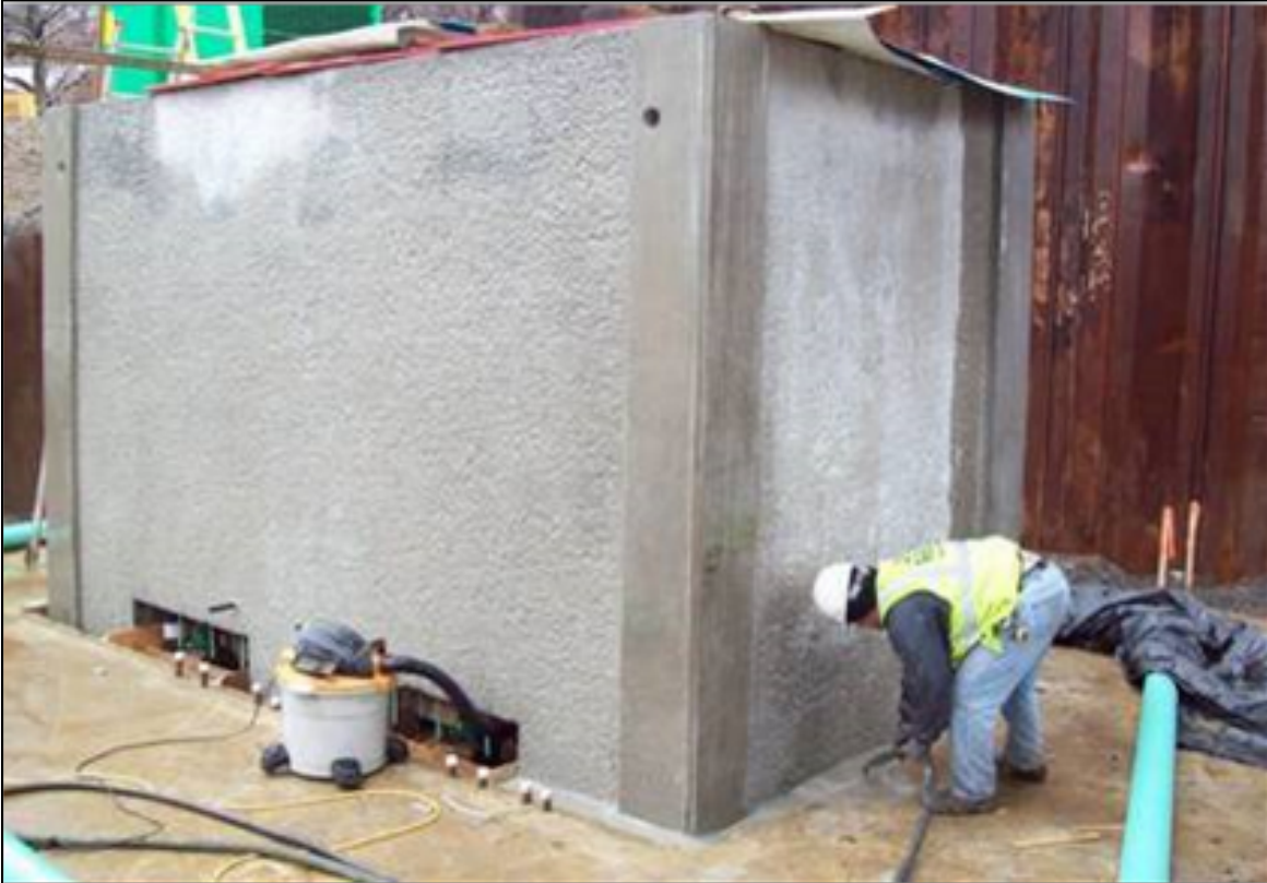
Figure 8.18 – Aligning and grading the starter (bottom) segment to achieve the proper geometry and positioning for the column. In this photo, pockets for jacks were used to align and grade the starter segment.
