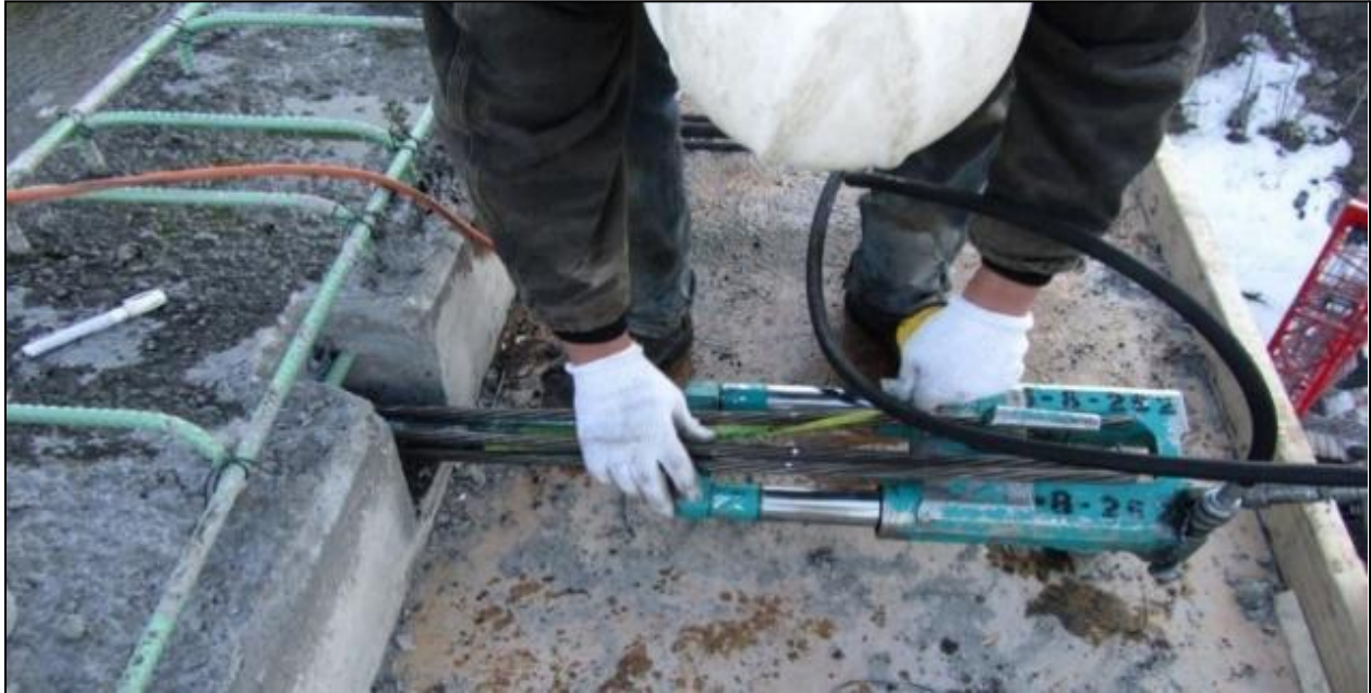
Figure 5.39 – Stressing transverse tendons (Photo Courtesy of NMDOT)
