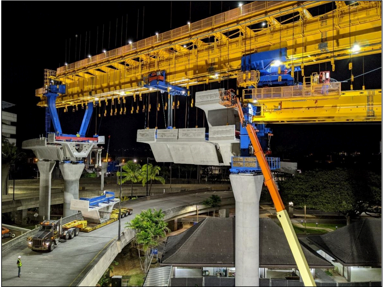
Figure 3.2 - Precast Segmental Erection with Overhead Articulating Gantry, (Photo Courtesy of Traylor Bros. Inc.)
