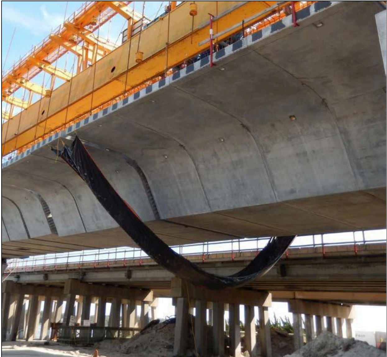
Figure 12.4 – Using an Epoxy Jointing Diaper (Photo Courtesy of FIGG)
