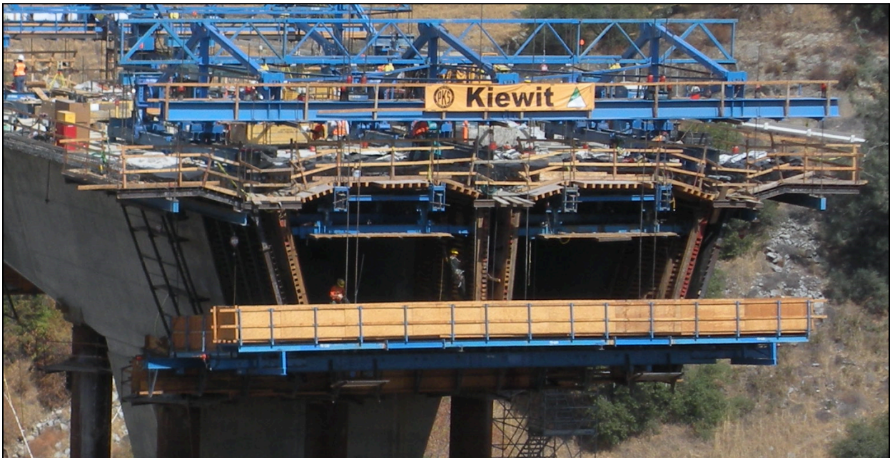
Figure 5.23 – Two cell box with three traveler frames, Folsom Dam Bridge, CA (Photo Courtesy of Kiewit)
