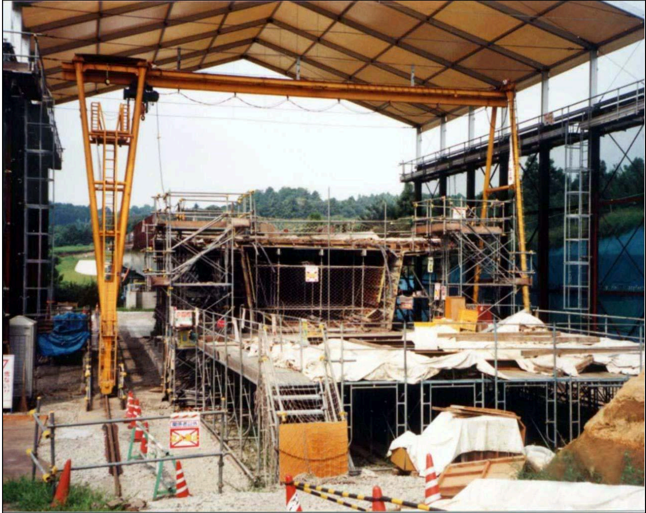
Figure 6.13 – Casting Yard Behind an Abutment (Photo Courtesy of PSM Construction USA, Inc.)
