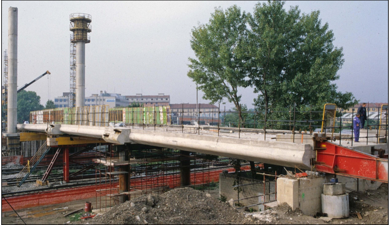
Figure 6.12 – Cable-Stayed Bridge: Launching the Superstructure on Temporary Piers Before Suspension – Italy (Photo Courtesy of Marco Rosignoli)
