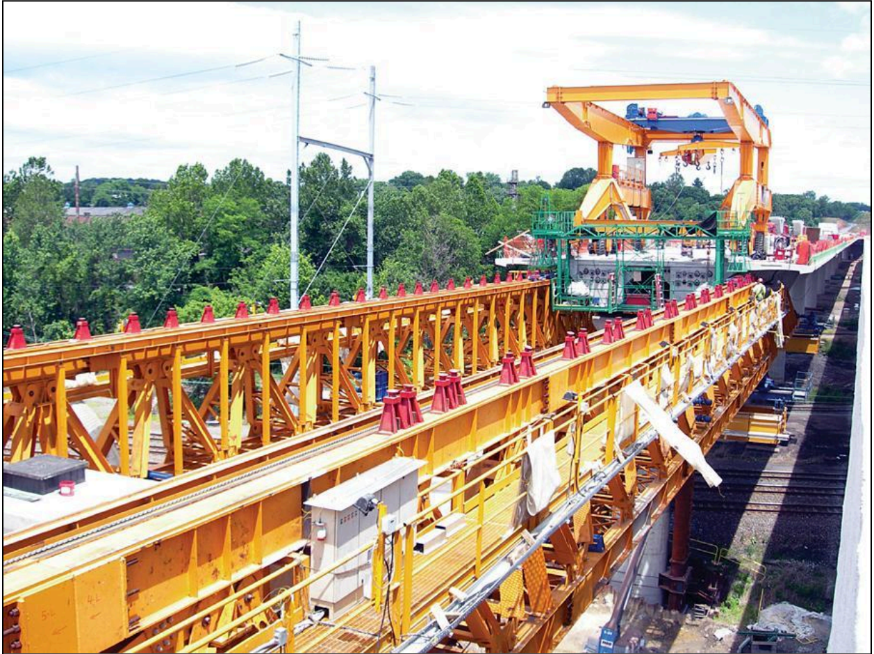
Figure 3.27 – Erection Equipment Required to Pass over the Railroad and Under the Power Lines (Photo Courtesy of FIGG)
