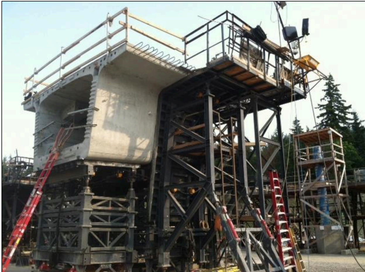
Figure 9.32 – Aligning the Match-Cast Segment in a Short-Line Casting Cell with Survey Tower in Background (Photo Courtesy of PCL Civil Constructors, Inc.)
