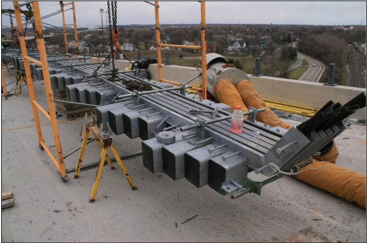
Figure 14.7 – Installation of a Modular Expansion Joint System, Veterans’ Glass City Skyway, OH (Photo Courtesy of FIGG)
