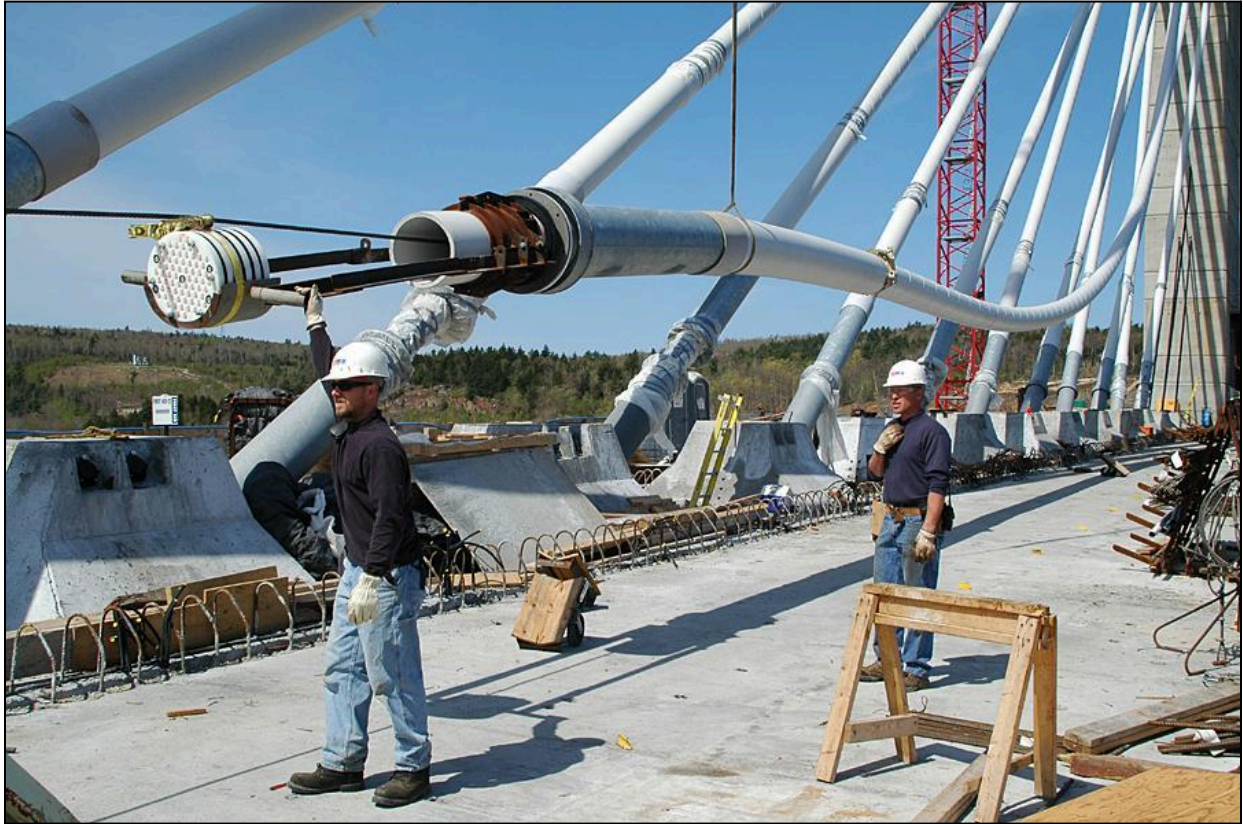
Figure 7.70 – HDPE Pipe Erection, Penobscot Narrows Bridge, ME (Photo Courtesy of FIGG)
