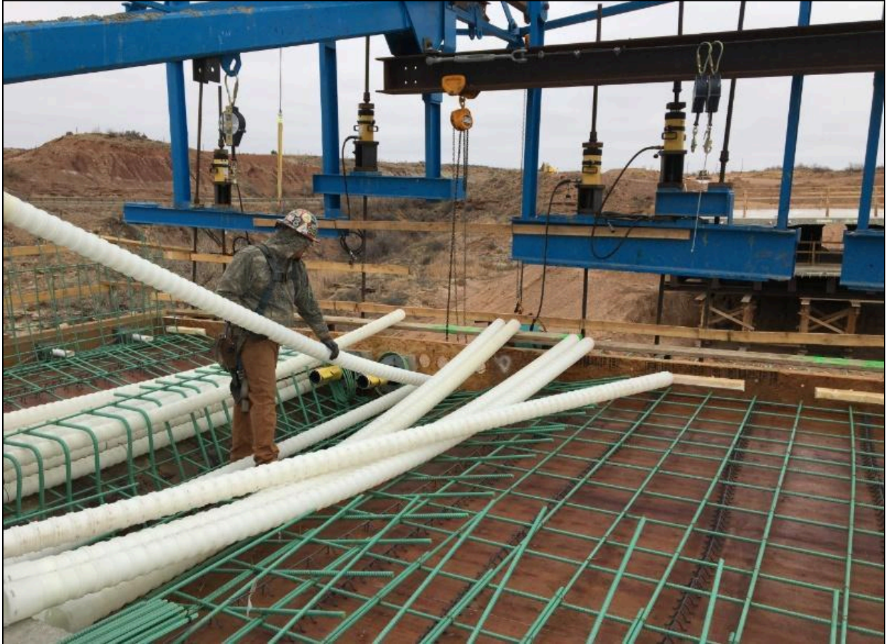
Figure 5.42 - Installing cantilever ducts for the top deck. (Photo Courtesy of NMDOT)
