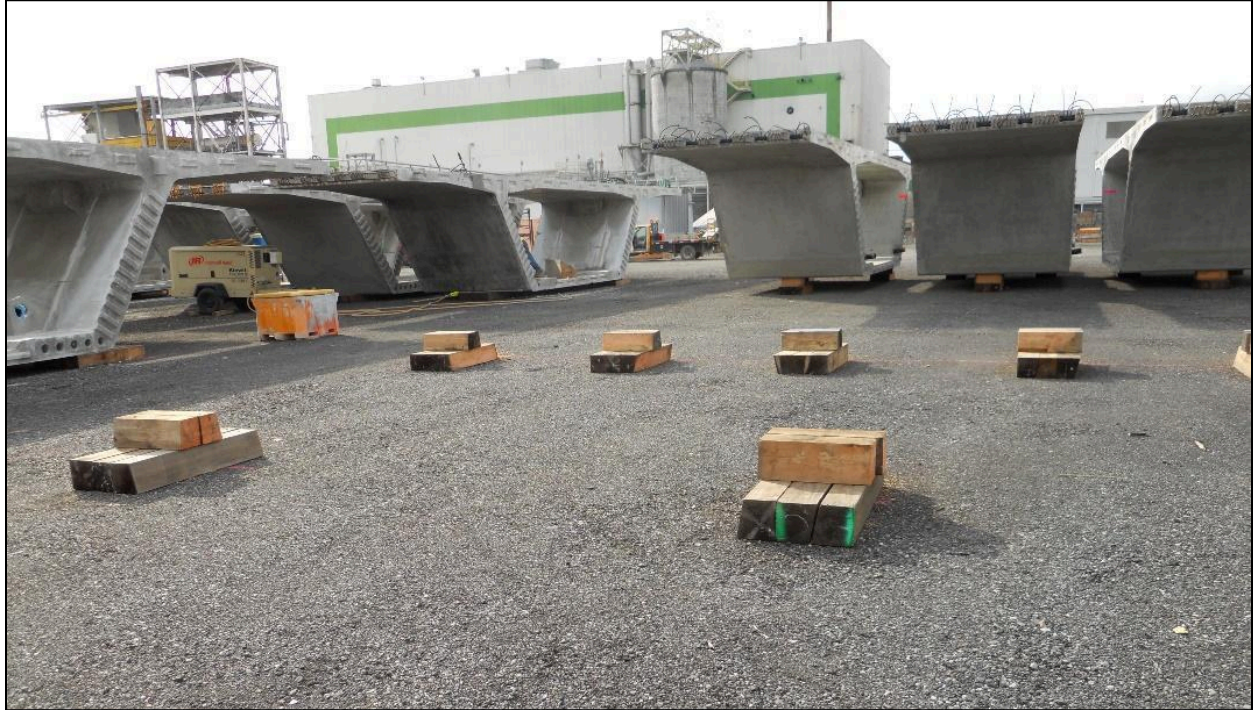
Figure 10.4 – Segment Storage Using Three-Point Support Configuration to Prevent Warping [Note Support Under the Webs] (Photo Courtesy of Elie Homs)
