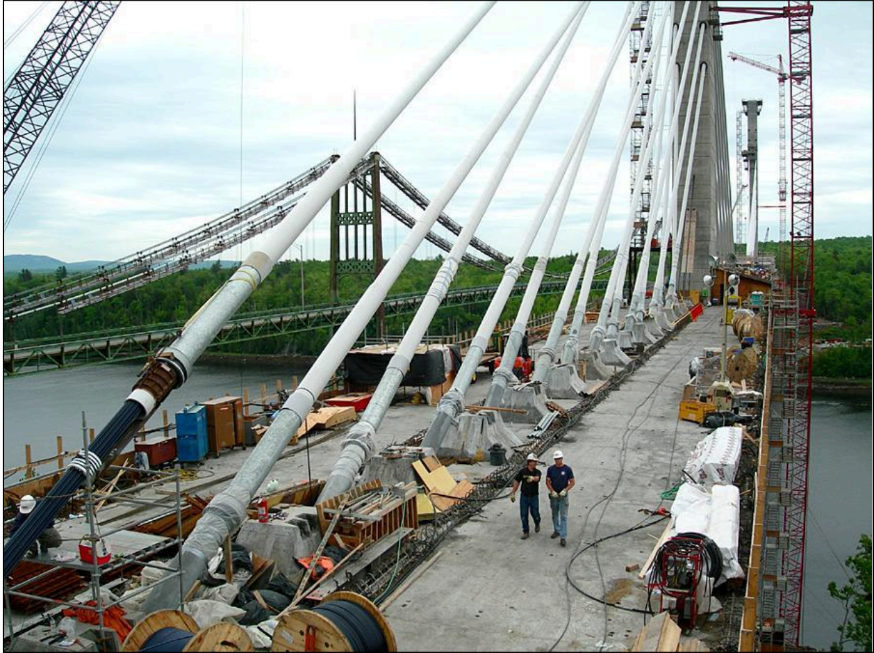
Figure 7.76 – Previously Installed Stay Cables with Temporary Protection during Construction (Photo Courtesy of FIGG)
