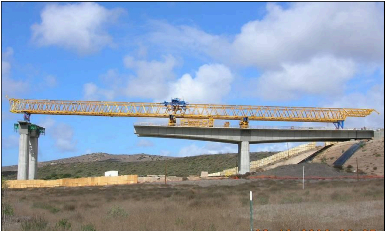
Figure 4.32 – Erection Gantry Launched Forward, Otay River Bridge, CA (Photo Courtesy of SYSTRA IBT)
