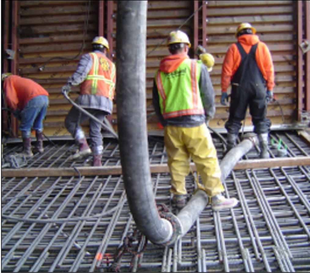
Figure 5.44 – Segment concrete placement (Photo Courtesy of McNary, Bergeron, and Johannesen)
