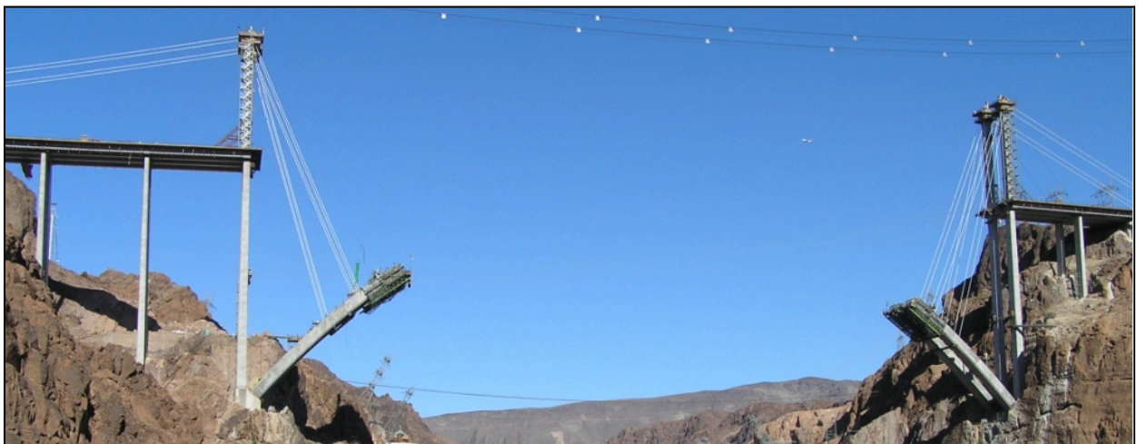
Figure 5.7 – Cast-in-Place Cantilever Arch: Hoover Dam Bypass Bridge, AZ-NV (Photo Courtesy of McNary Bergeron & Johannesen)
