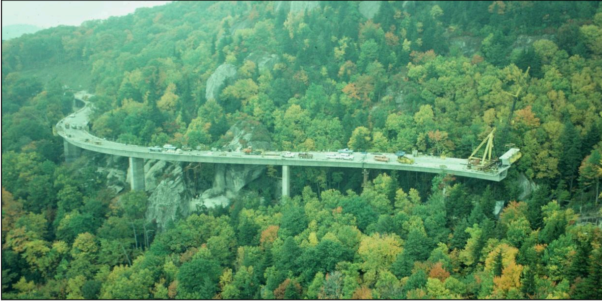
Figure 1.4 –Precast Segmental Progressive Placement, Linn Cove Viaduct, NC (Photo Courtesy of FIGG)
