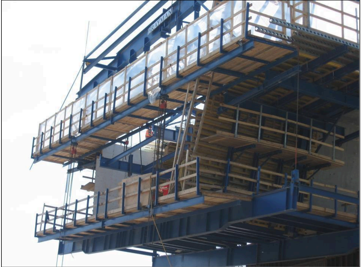
Figure 15.4 – Construction Access at the Leading Edges (Photo courtesy of Brayman Construction.)
