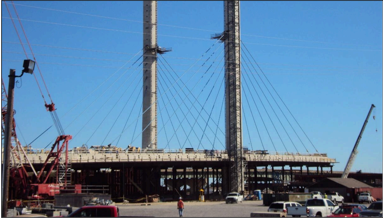
Figure 7.40 – Complete Back Span on Falsework – Potential for Entrainment, Charles W. Cullen Bridge, DE (Photo Courtesy of AECOM)
