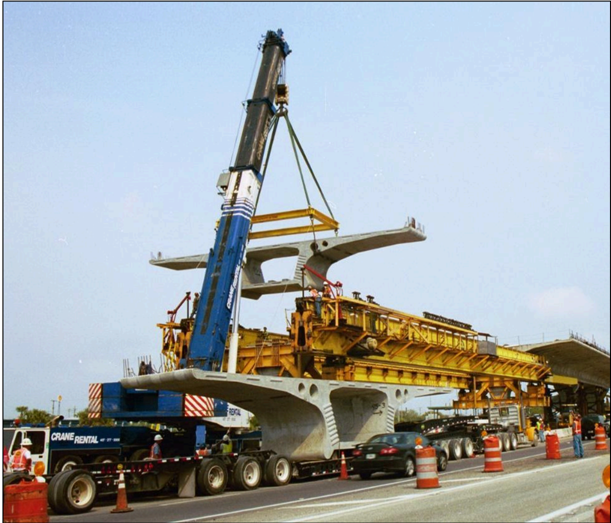
Figure 3.15 – Erecting Segments onto Trusses, Lee Roy Selmon Crosstown Expressway, FL (Photo Courtesy of PCL Civil Constructors, Inc.)
