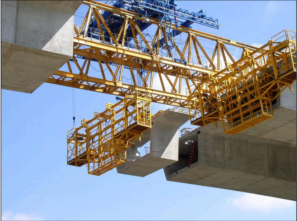
Figure 4.23 – Stressing Platforms on the Otoy River Bridge, CA (Photo Courtesy of SYSTRA IBT)
