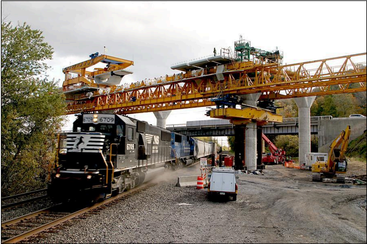
Figure 3.10 – Maintenance of Railway Traffic, Susquehanna River Bridge, PA (Photo Courtesy of FIGG)
