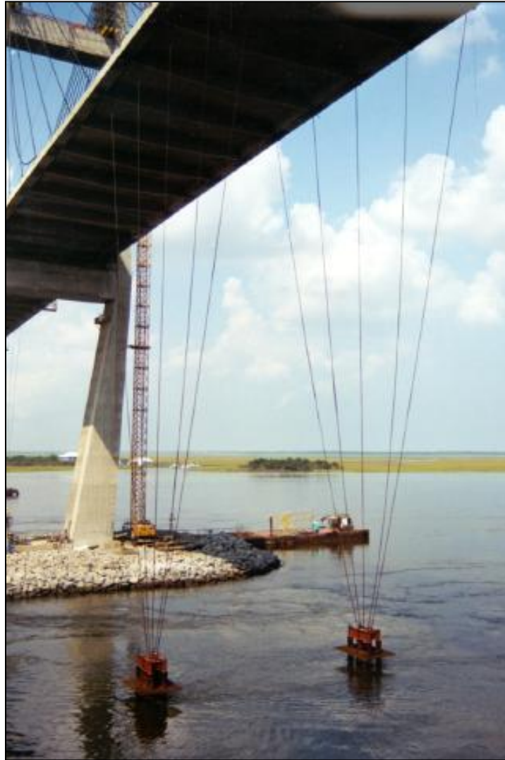
Figure 7.38 – Superstructure Stabilizing Cables, Sidney Lanier Bridge, GA (Photo Courtesy of FIGG)
