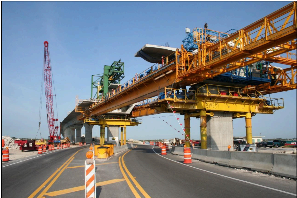
Figure 3.9 – Maintenance of Road Traffic, Ernest F. Lyons Bridge, FL (Photo Courtesy of PCL Civil Constructors, Inc.)
