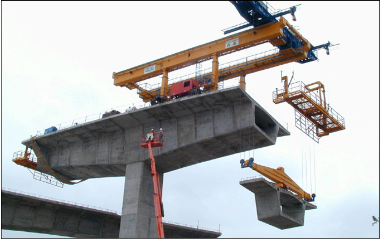
Figure 10.33 – Specialized Erector in Use, Dallas High Five Interchange Project, TX (Photo Courtesy of DEAL/Rizzani de Eccher USA)
