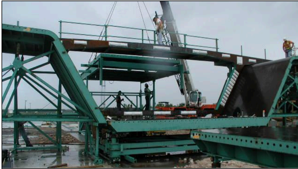
Figure 9.20 – Segment Form Assembly (Photo Courtesy of FIGG)
