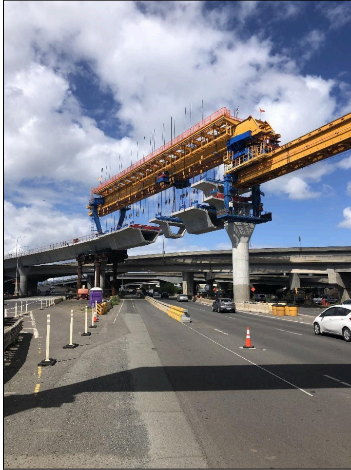
Figure 3.11 – Maintenance of Road Traffic, Honolulu Light Rail, HI (Photo Courtesy of Traylor Bros. Inc.)
