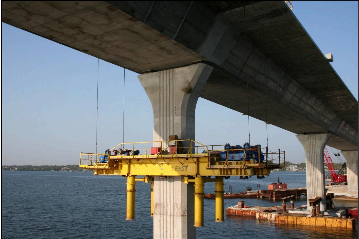
Figure 3.26 – Temporary Supports Being Lowered After Span is Complete, Ernest F. Lyons Bridge, FL (Photo Courtesy of PCL Civil Constructors, Inc.)
