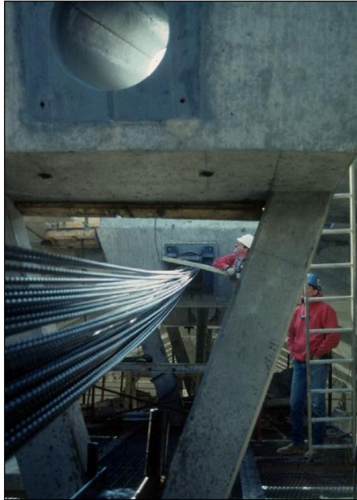
Figure 7.73 – Bundle of Strands Being Pulled through the Guide Pipe (Photo Courtesy of FIGG)
