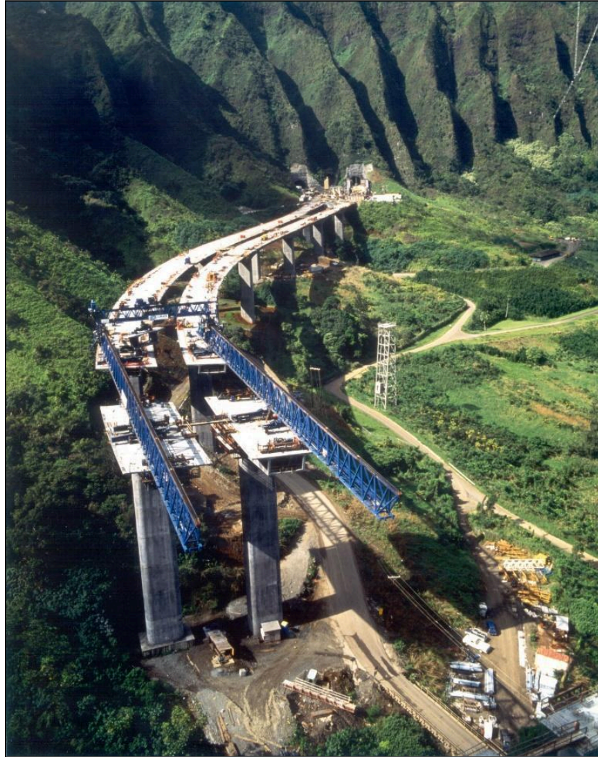
Figure 4.33 – Self-Launching Dual Erection Gantry, H-3 Windward Viaduct, Oahu, HI (Photo Courtesy of T.Y. Lin International)
