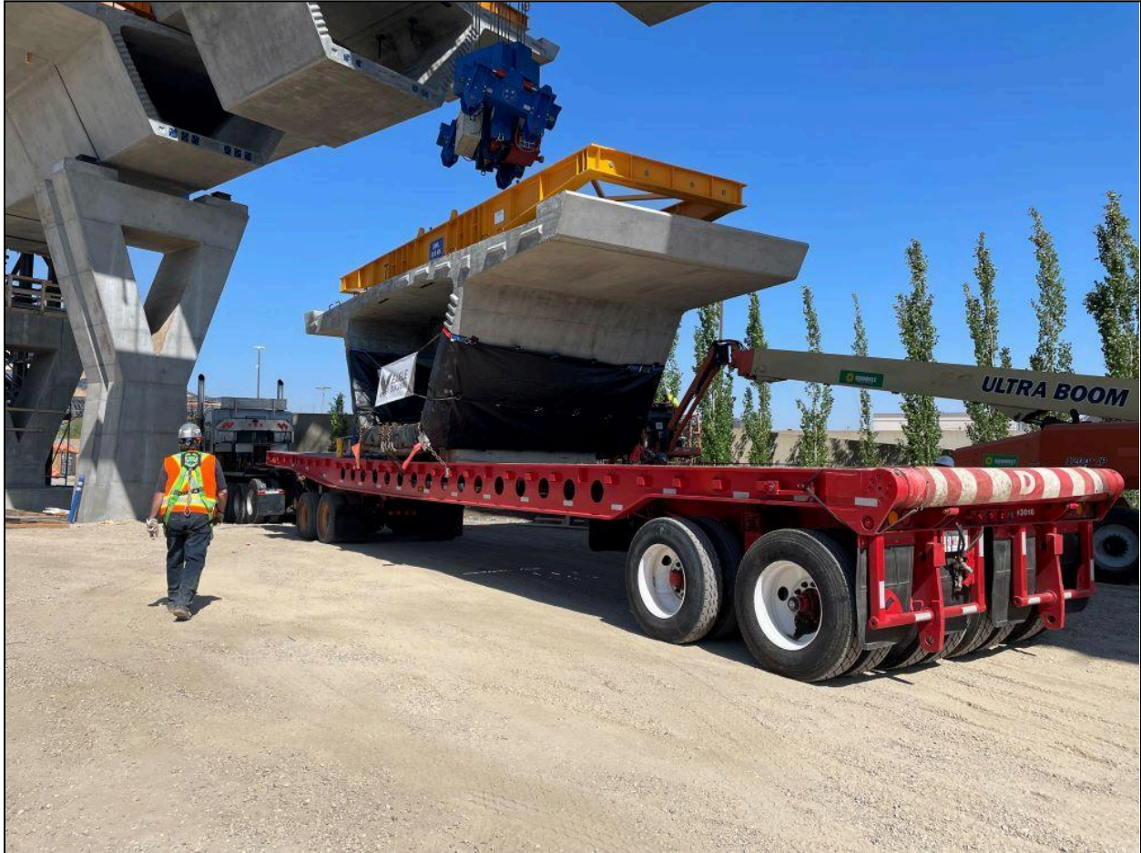
Figure 10.13 – Delivery of a 42 ton segment with tarping to protect the bottom of the segment from contamination during transport (Photo Courtesy of Parsons)
