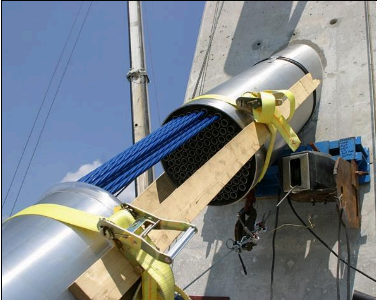
Figure 7.75 – Strands Being Threaded Through the Saddle (Cradle) Pipe (Photo Courtesy of FIGG)
