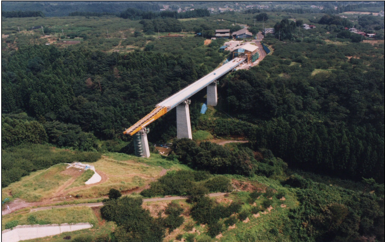
Figure 6.1 – Incremental Launching Segmental Bridge (Photo Courtesy of PSM Construction USA, Inc.)
