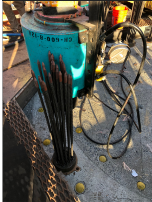
Figure 8.21 – Stressing Vertical Column Tendon, SoFi Stadium, CA (Photo Courtesy of McNary, Bergeron, and Johannesen)
