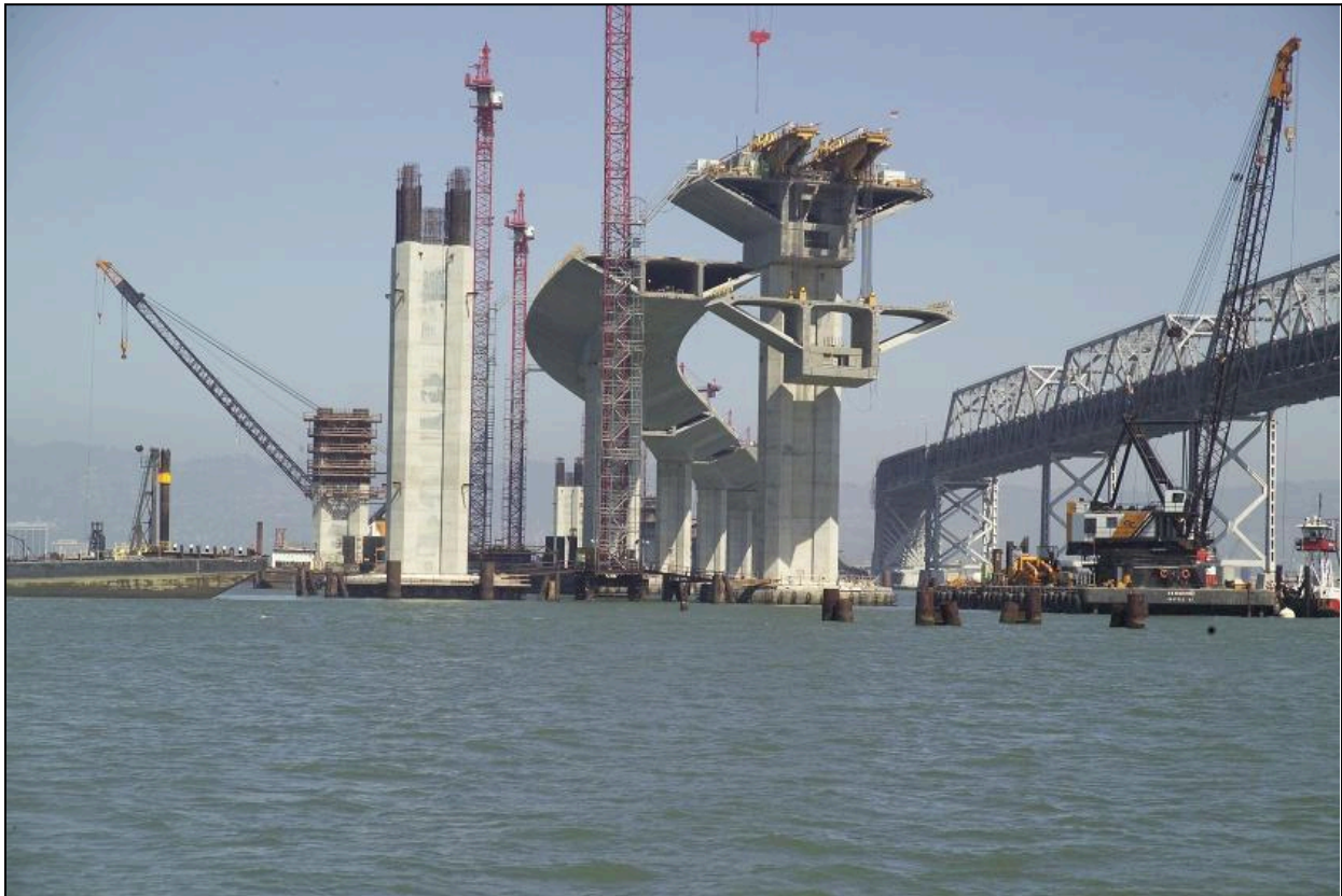
Figure 10.31 – Balanced-Cantilever Erection using Beam-and-Winch, San Francisco-Oakland Skyway, CA (Photo Courtesy of Kiewit/Flatiron/Manson Joint Venture)
