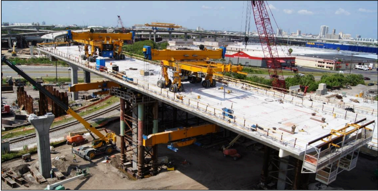
Figure 4.29 – Mobile Lifters Erecting Cantilevers on the I-4 Connector Project, FL (Photo Courtesy of PCL/Archer-Western JV)
