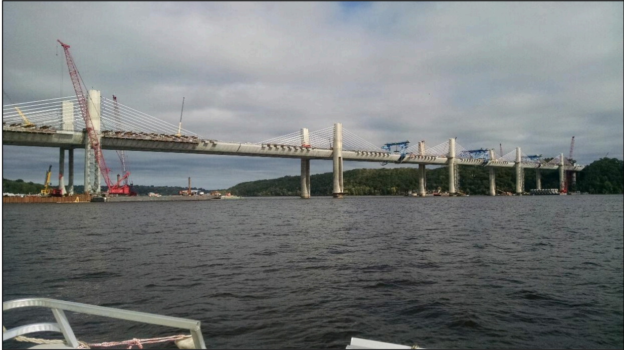
Figure 7.88 – Saint Croix Bridge, MN-WI (Photo Courtesy of Structural Technologies)
