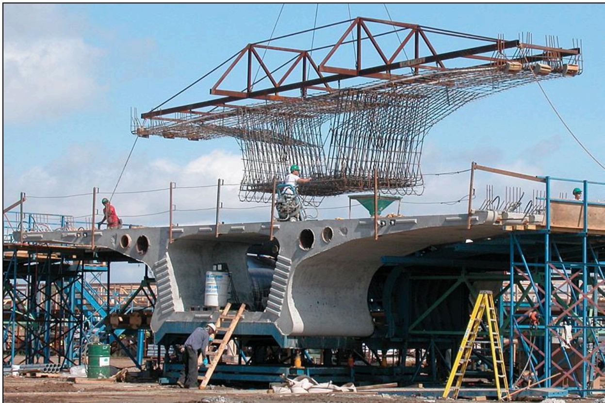
Figure 9.8 - Short-Line Form, Lee Roy Selmon Crosstown Expressway, FL (Photo Courtesy of FIGG)
