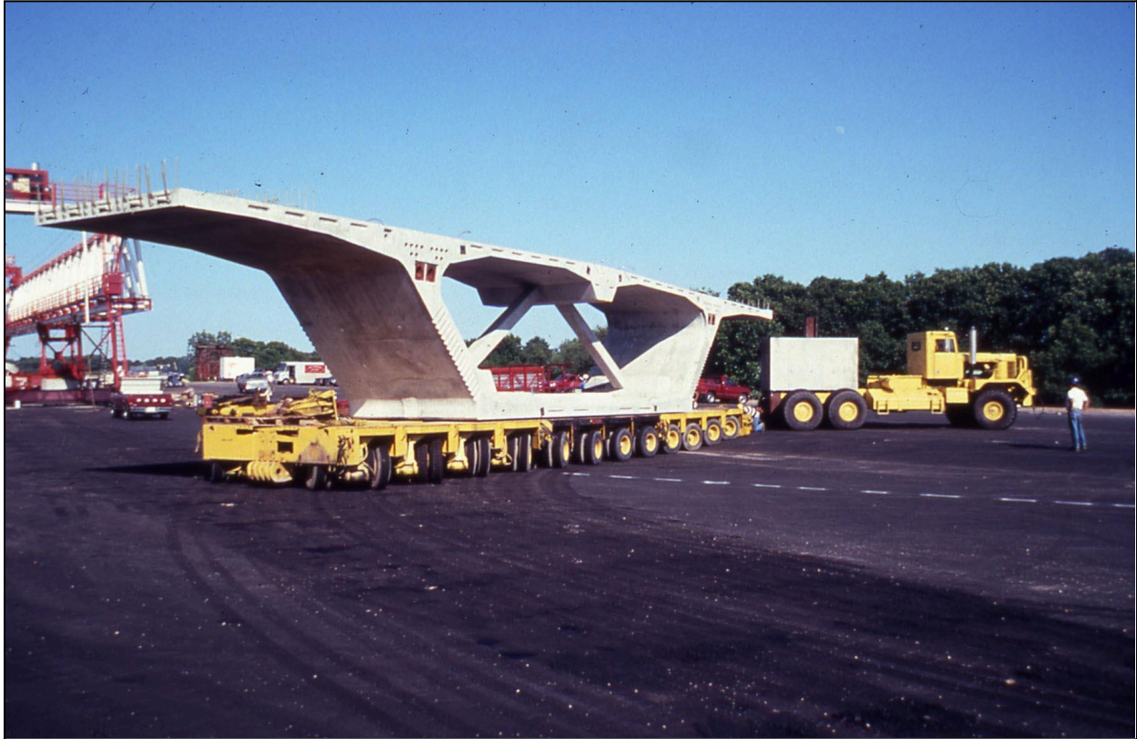
Figure 10.9 – Truck and Segment on a Trailer, Baldwin Bridge, CT (Photo Courtesy of Perini/Homsi)
