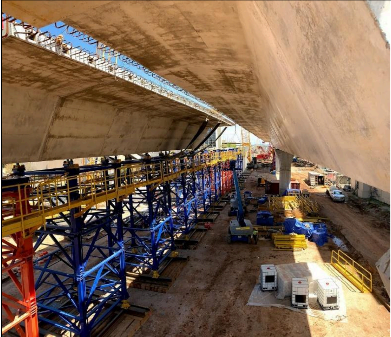
Figure 10.23 – Full Span Erection on Shoring Falsework, I-59/I-20 Project, AL (Photo Courtesy of McNary Bergeron & Johannesen)
