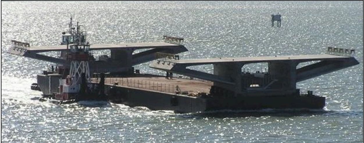
Figure 10.7 – Barge Transporting Segments (Photo Courtesy of Flatiron Constructors, Inc.)
