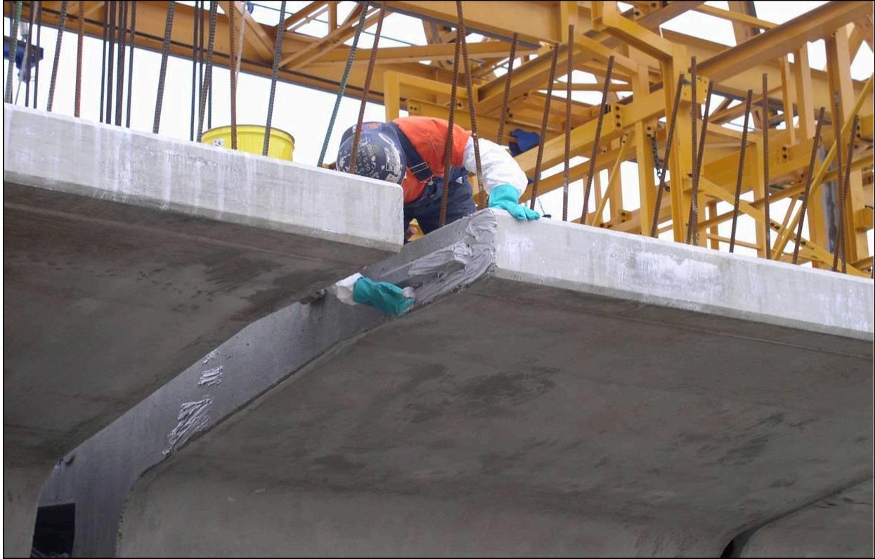
Figure 4.20-1 – Epoxy Application (Photo Courtesy of SYSTRA IBT)
