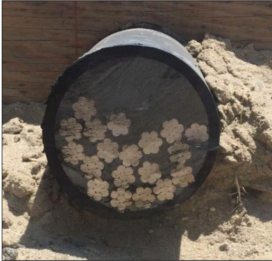
Figure 12.9 – Completely Filled Duct with Prepackaged Grout (Photo Courtesy of FIGG)
