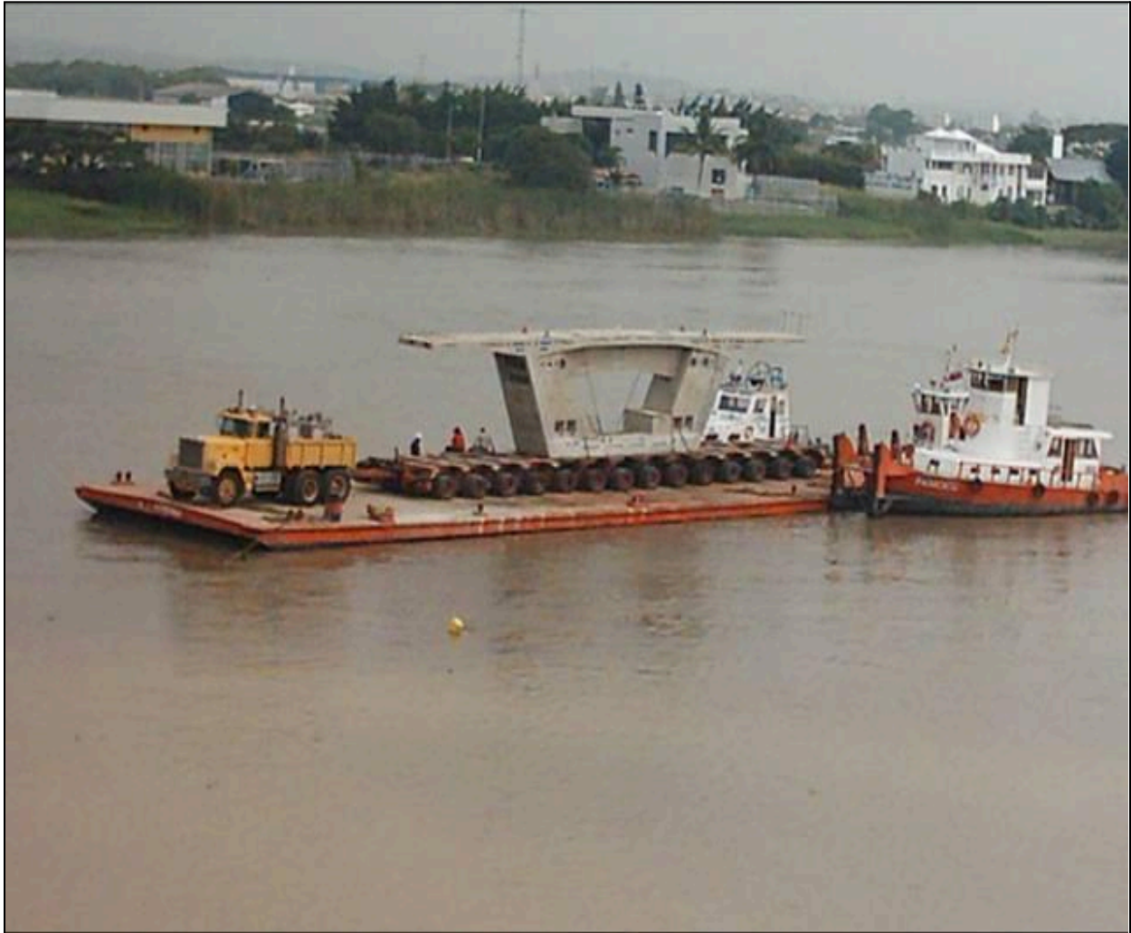
Figure 10.6 – Barge Transporting a Segment Hauler (Photo Courtesy of Elie Homsi)
