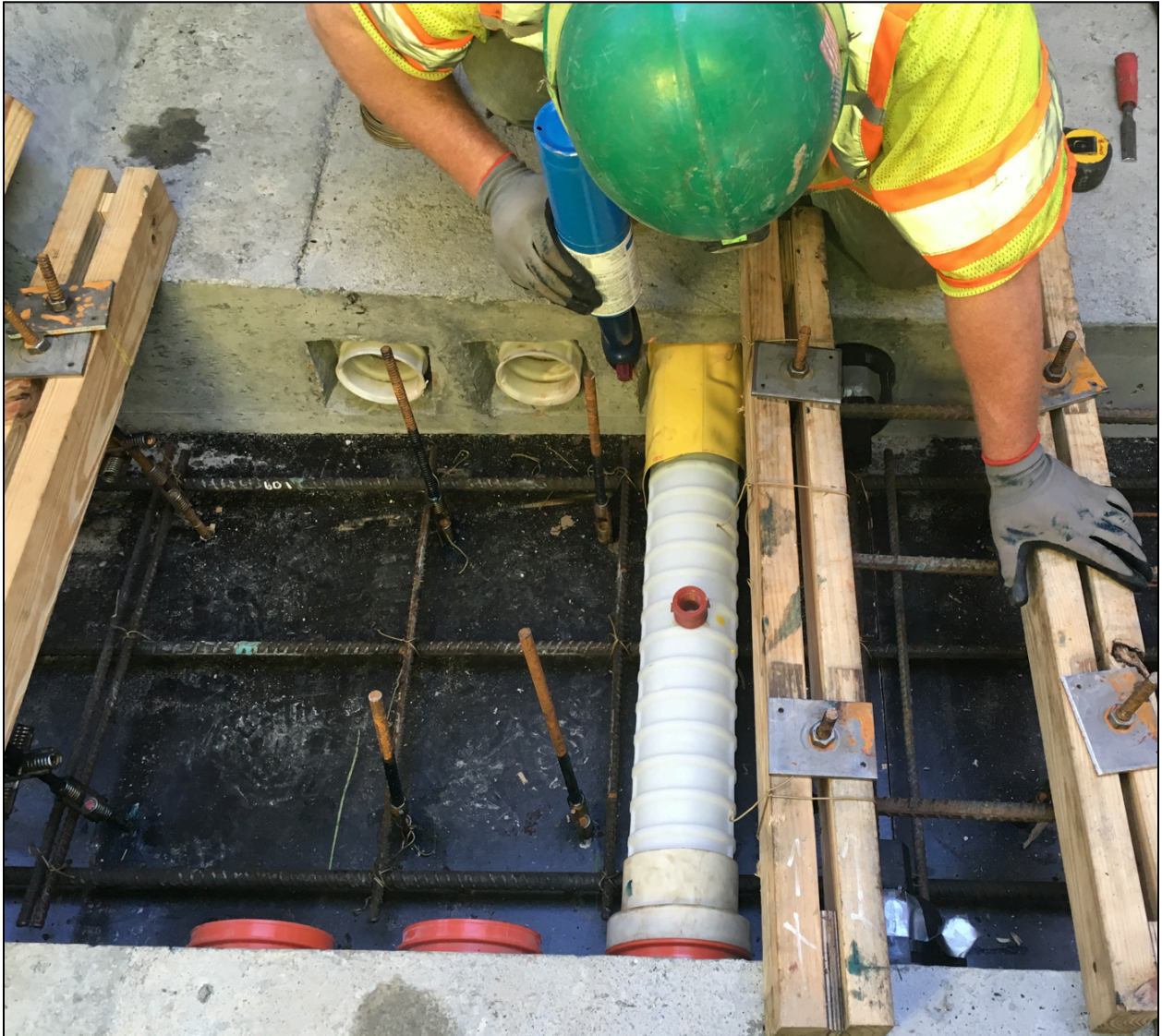
Figure 4.38 – Coupling of Ducts at Cast-in-Place Closure Joint (Photo Courtesy of SYSTRA IBT)
