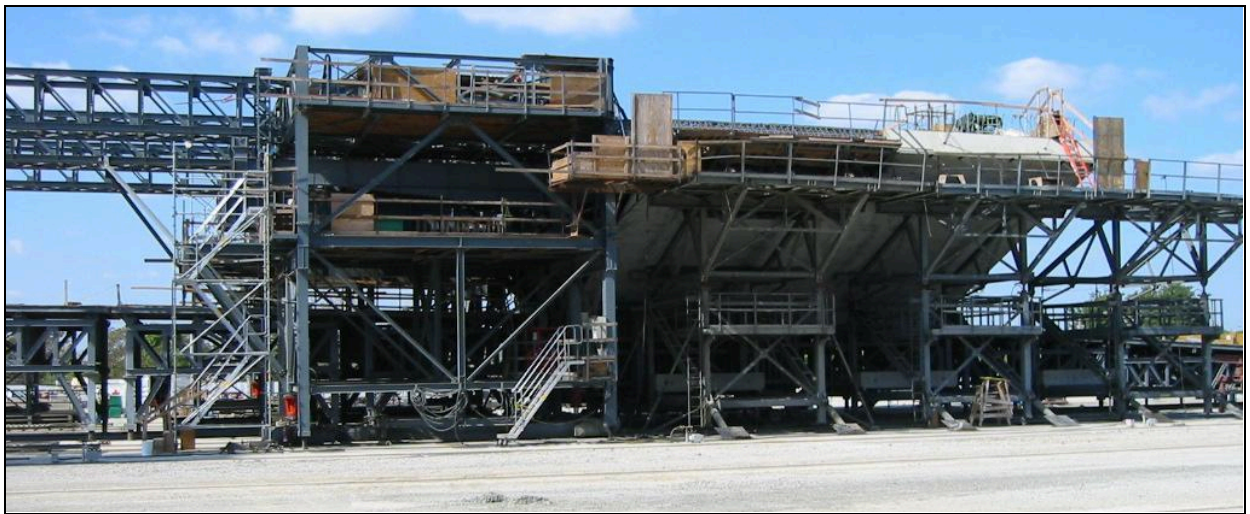
Figure 9.5 – Side View of a Long-Line Casting Bed, San Francisco-Oakland Bay Bridge Skyway, CA (Photo Courtesy of Flatiron Construction)
