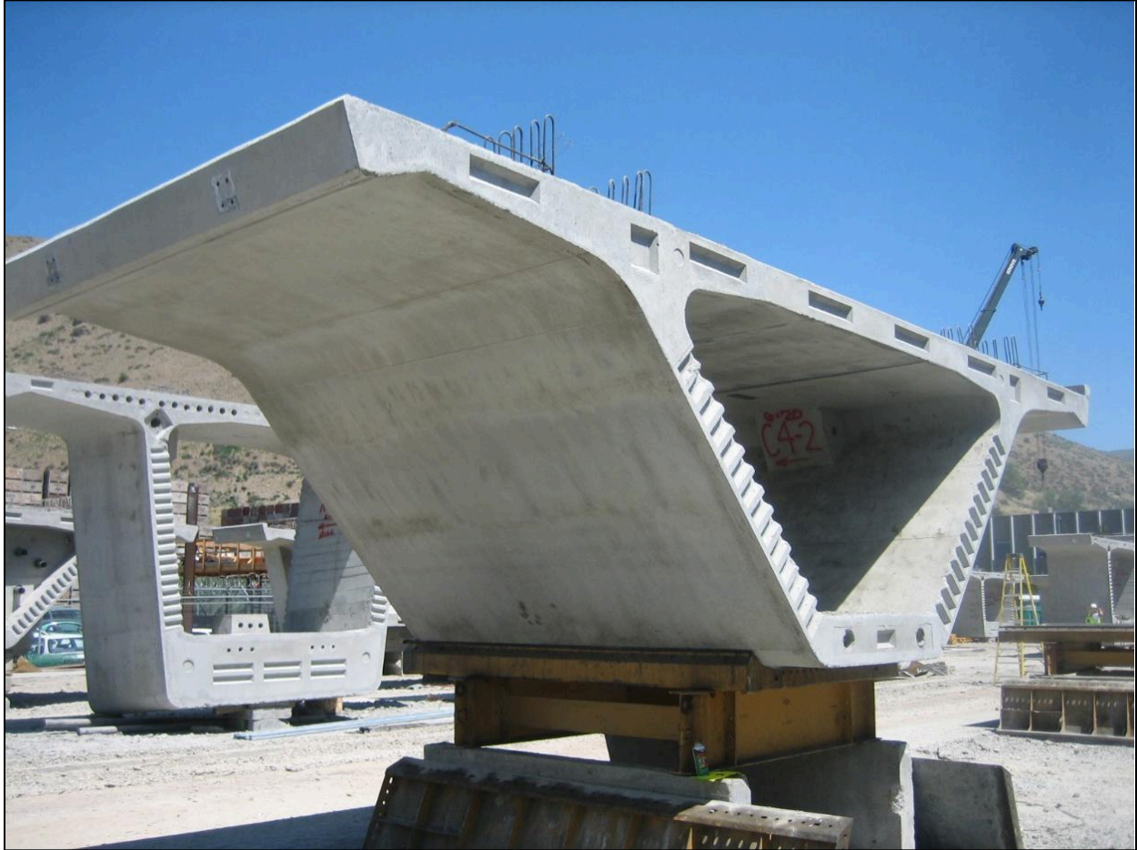
Figure 9.42 – Precast Segment with North- and Southbound Steel Plinths Cast-in-Place On-Site (Photo Courtesy of Fueled Photography/PCL Civil Constructors, Inc.)
