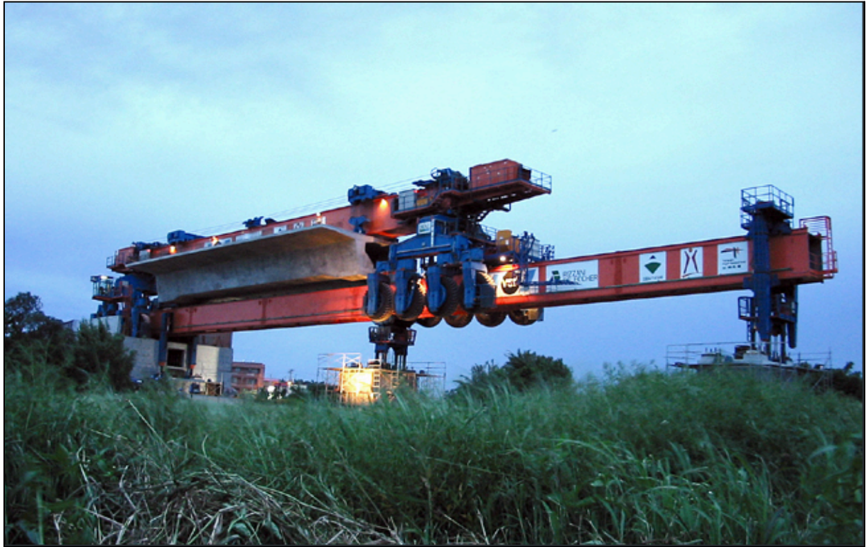
Figure 10.21 – Full Span Carrier / Erector (Photo Courtesy of DEAL/Rizzani de Eccher USA)
