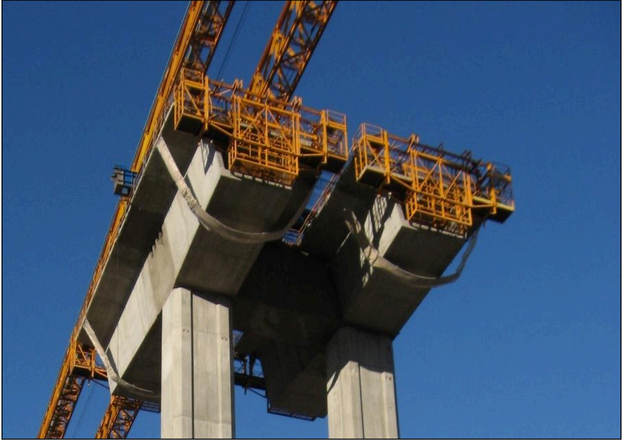
Figure 4.20-2 – Epoxy Application (Photo Courtesy of SYSTRA IBT)
