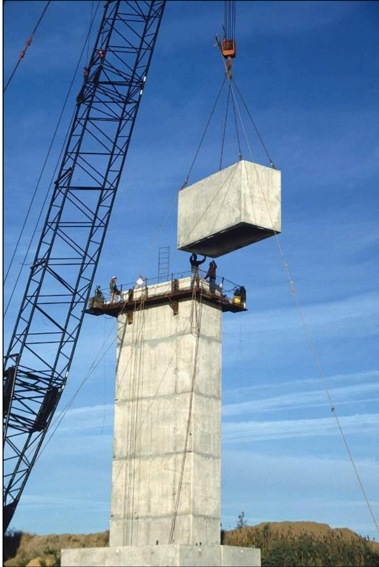
Figure 8.11 – Precast Column Erection, Korean War Veterans Memorial Bridge, DE (Photo Courtesy of Recchi America)
