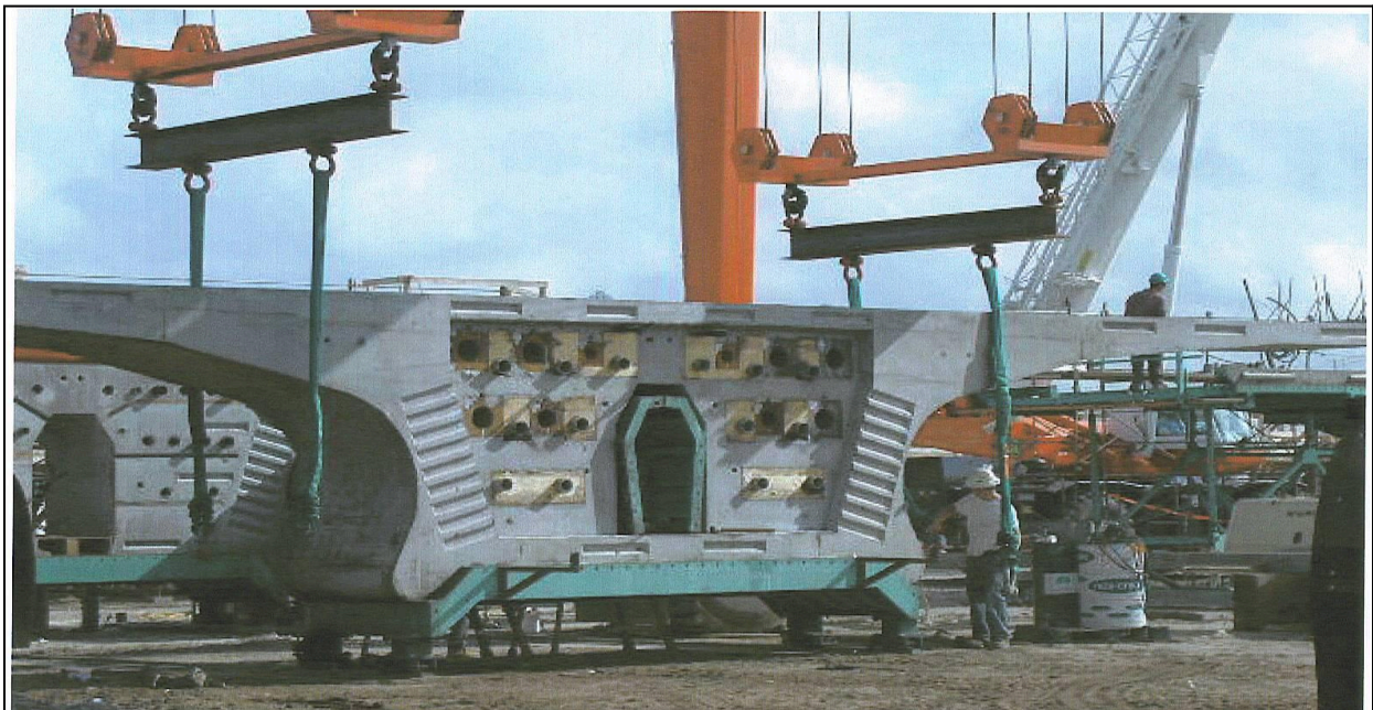
Figure 9.15 – Completed Diaphragm Segment, Lee Roy Selmon Crosstown Expressway, FL (Photo Courtesy of PCL Civil Constructors, Inc.)
