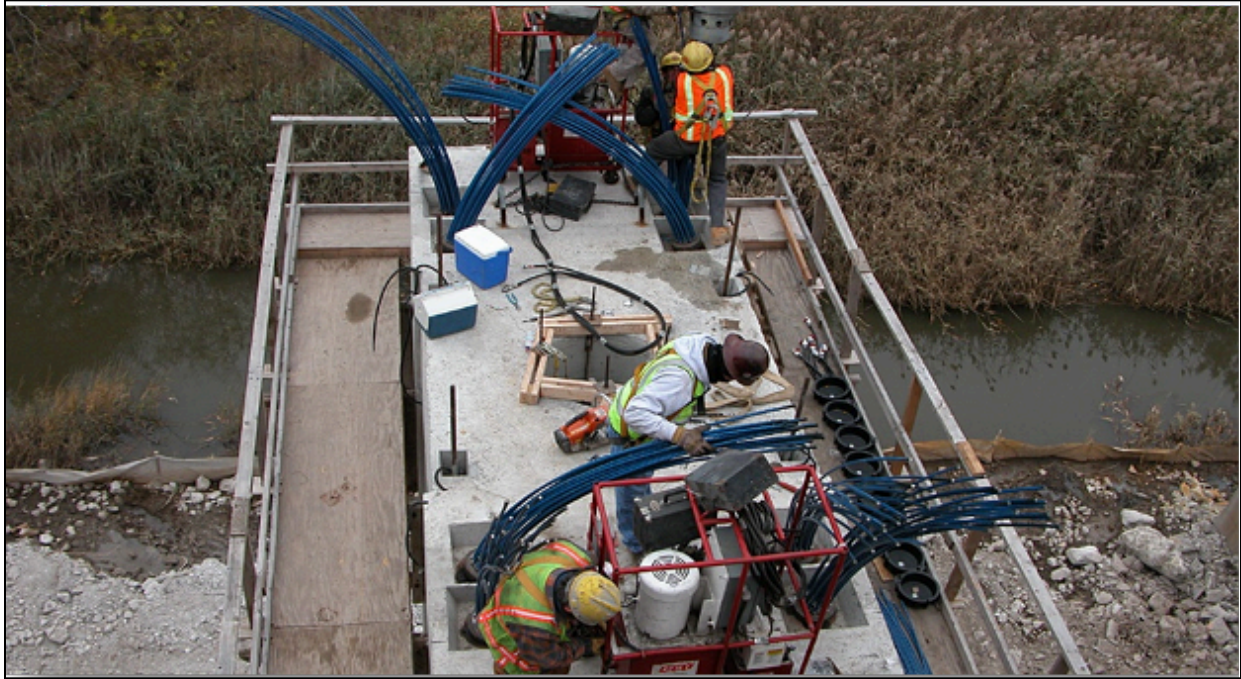
Figure 8.22 – Stressing Vertical Column Tendon, Route 36 Highlands Bridge, NJ (Photo Courtesy of J.H. Reid General Contractors)
