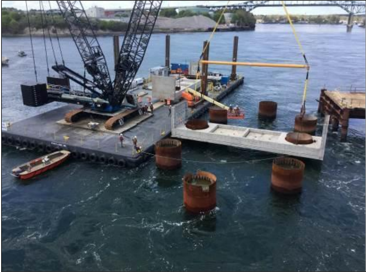
Figure 8.24 – Installation of Precast Tub Footing Segment (Photo Courtesy of Cianbro)
