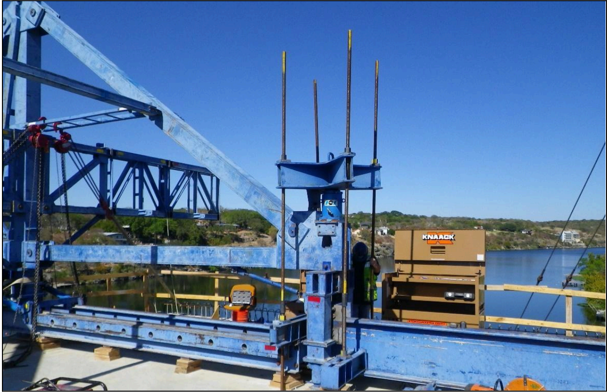
Figure 5.27 – Form Traveler Installation Step 3: Install Rear Tie-Down System (Photo Courtesy of Archer Western)
