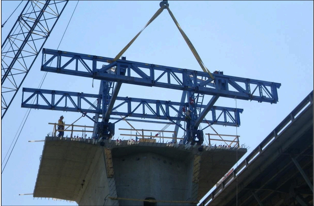
Figure 5.28 – Form Traveler Installation Step 4: Set Front Truss, Inner Frame, and Formwork (Photo Courtesy of Archer Western)
