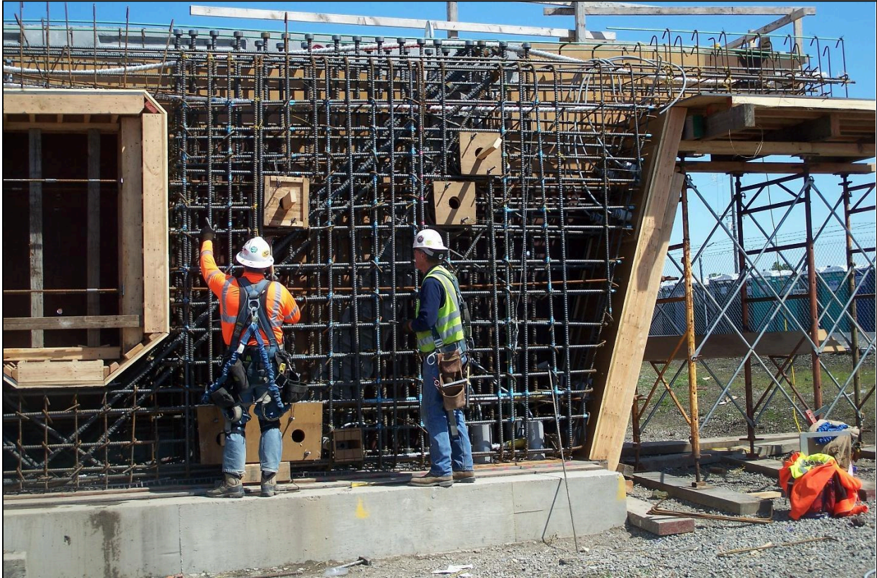
Figure 9.14 – Abutment Segment Form, SW Line Bridge, WA (Photo Courtesy of Atkinson Construction)
