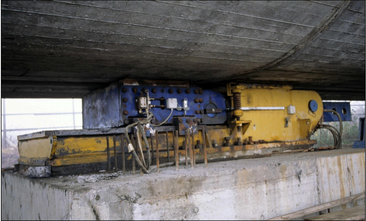
Figure 6.16 – Axial Friction Launching System (Photo Courtesy of Marco Rosignoli)
