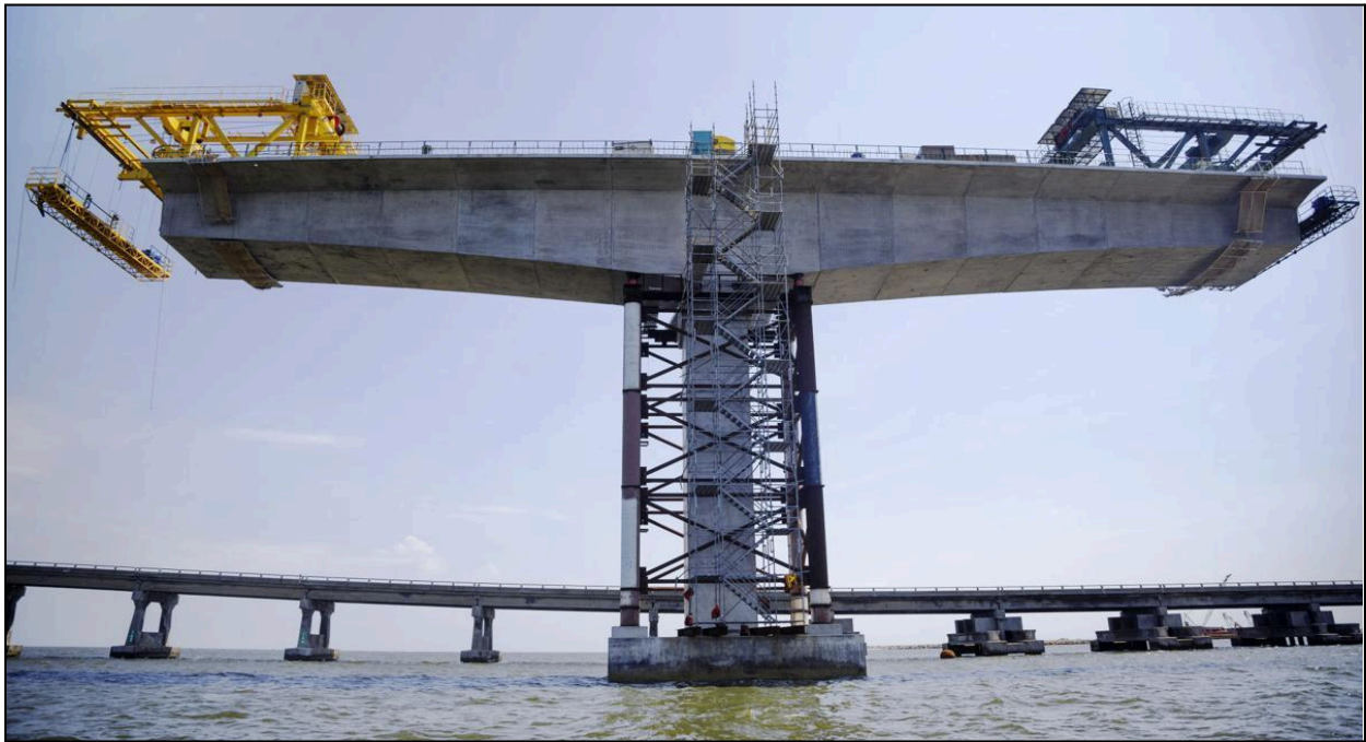
Figure 1.2 – Precast Balanced Cantilever, Bonner Bridge, NC (Photo Courtesy of RS&H)
