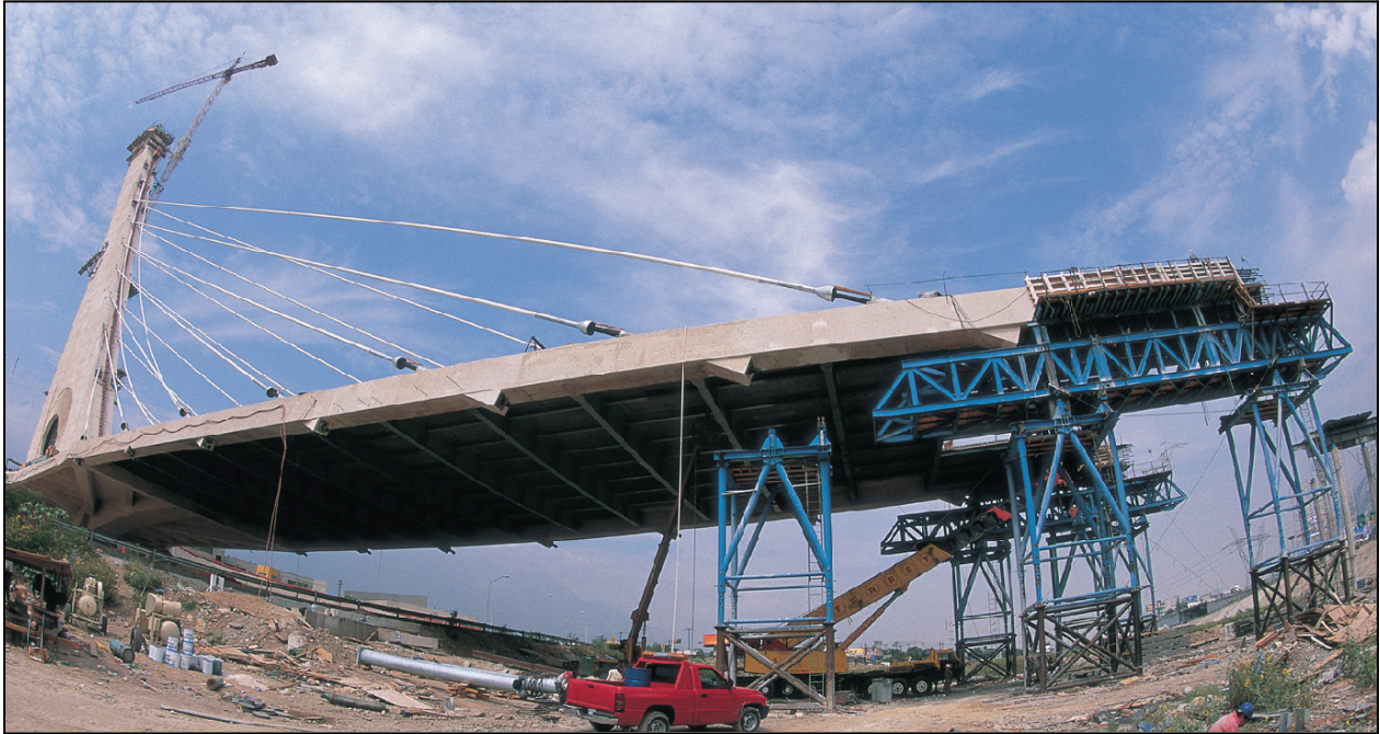
Figure 7.25 - Traveling Forms on Shoring for Edge Girders, Puente de la Unidad, Mexico (Photo Courtesy of VSL Mexico)
