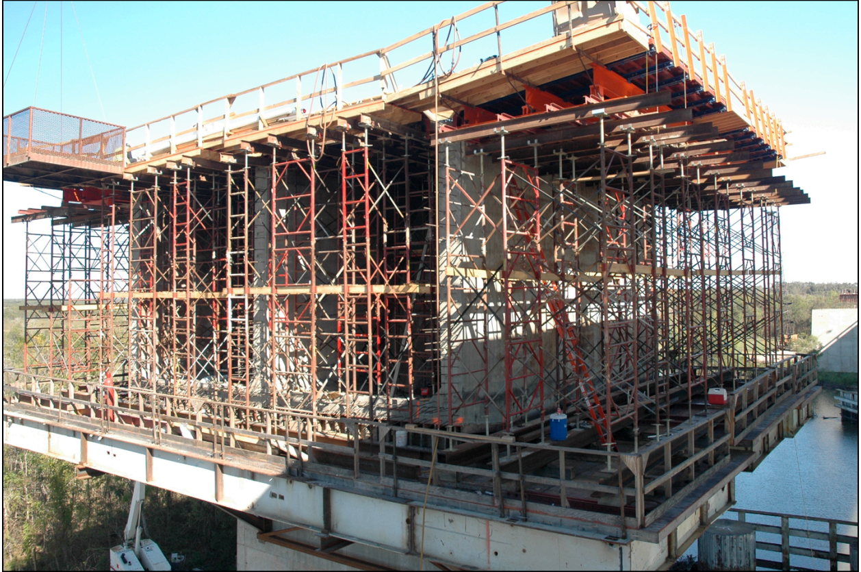
Figure 5.10 – Pier Table Top Slab Construction: Trinity River Bridge, TX (Photo Courtesy of Williams Brothers Construction)
