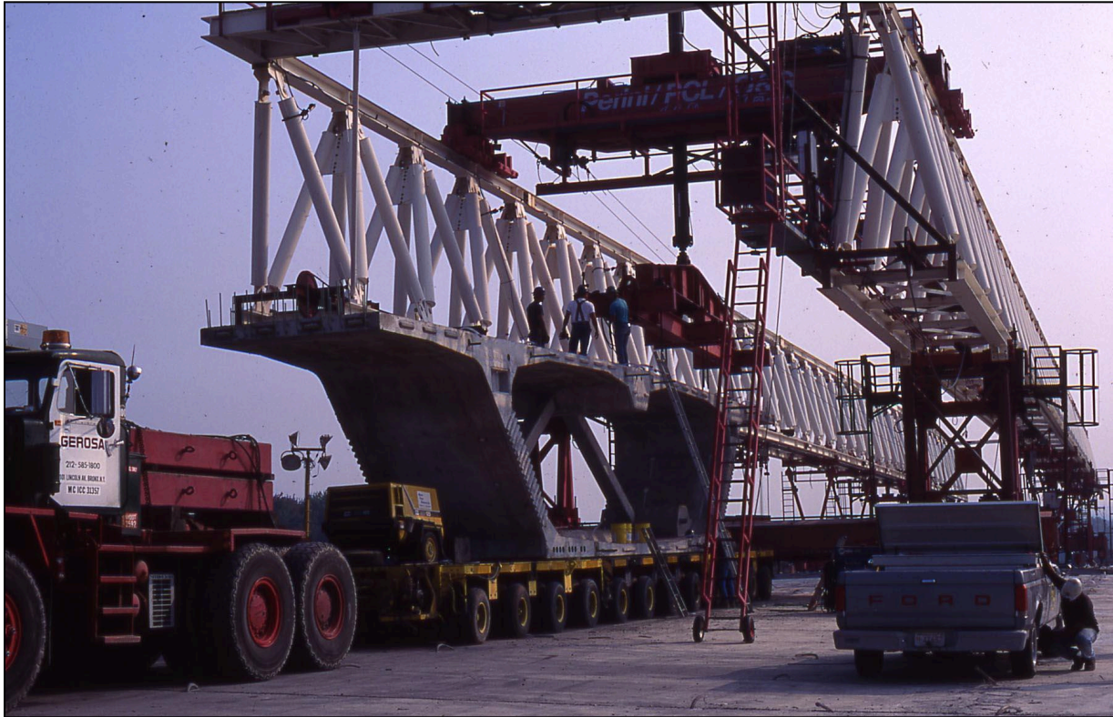
Figure 10.10 – Delivery of a Segment to the Launching Gantry, Baldwin Bridge, CT (Photo Courtesy of Perini/Homsi)
