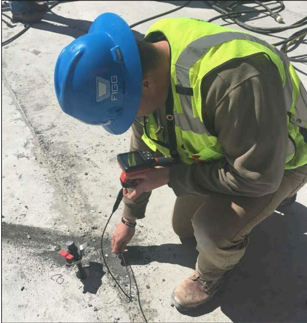
Figure 12.8 - Post-Grout Inspection Using Borescope (Photo Courtesy of FIGG)
