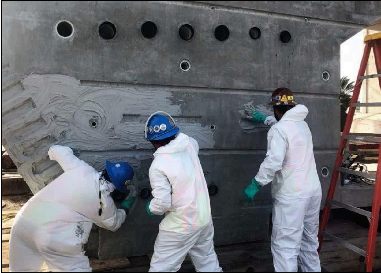
Figure 12.2 – Applying Epoxy onto Face of Segments (Photo Courtesy of FIGG)
