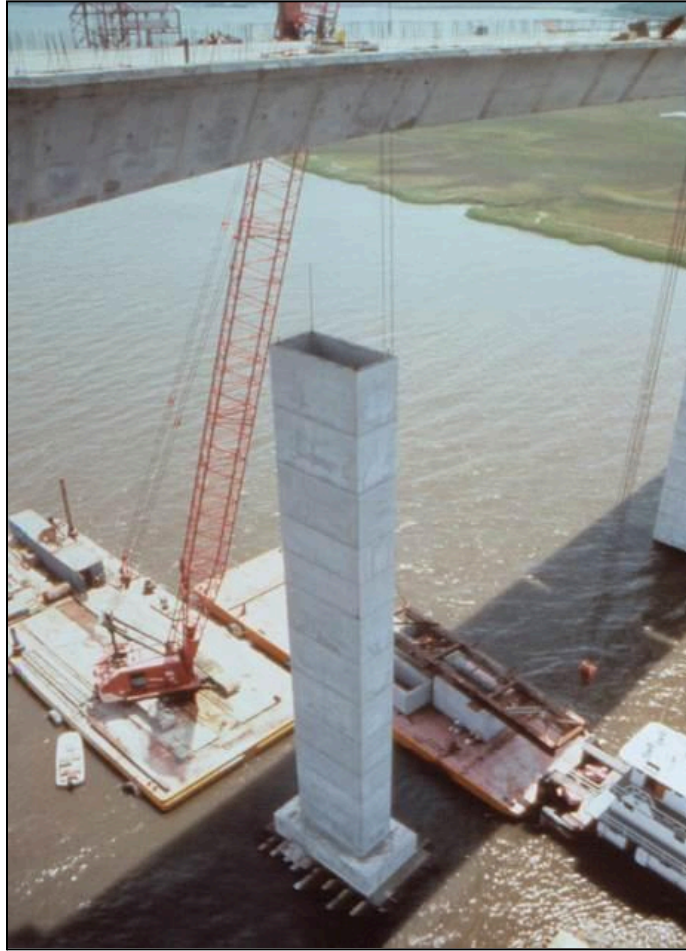
Figure 8.8 – Pier Column Disassembly, James Burroughs Edwards Bridge, SC (Photo Courtesy of FIGG)
