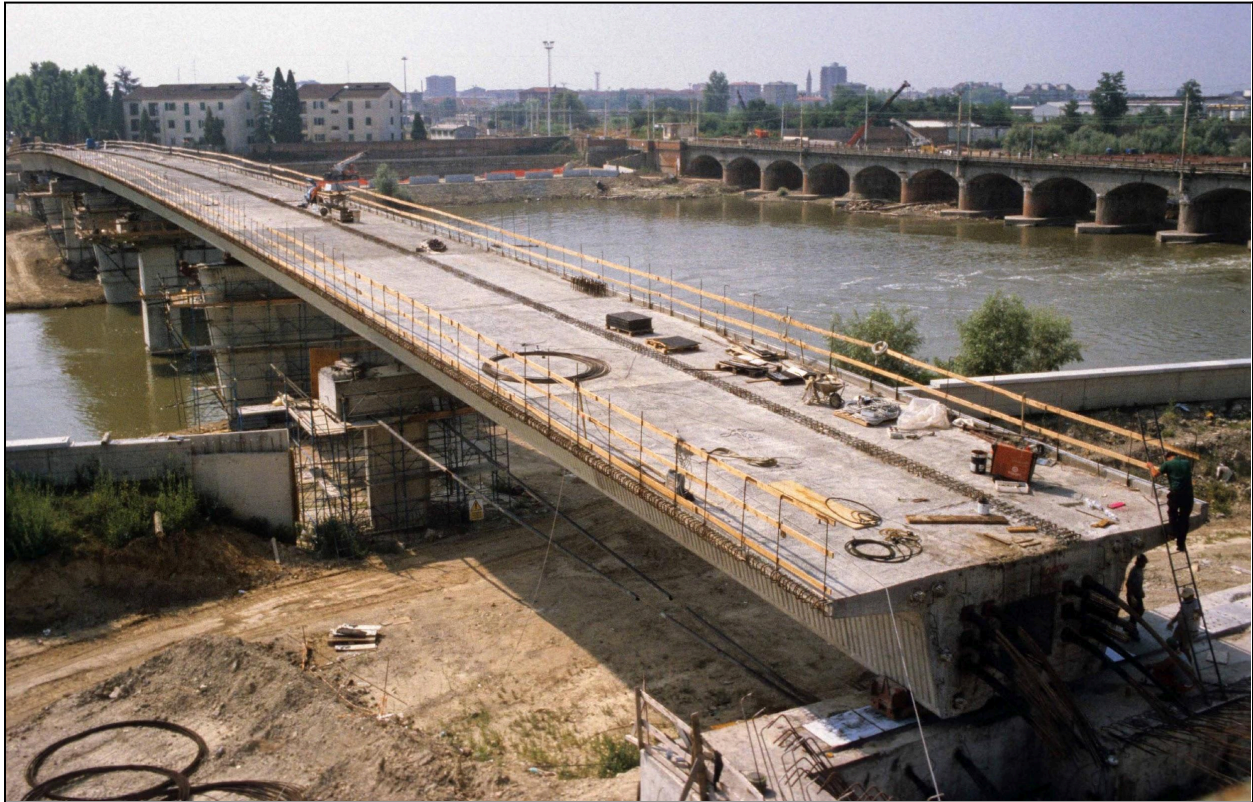
Figure 6.10 – Transverse Shift of the First Half of a Twin-Box Section on Launch Completion – Italy (Photo Courtesy of Marco Rosignoli)
