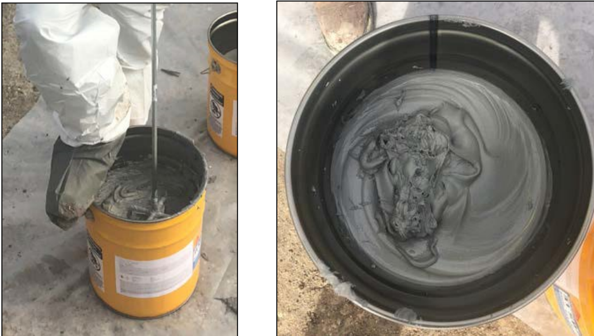
Figure 12.1 – Mixing Segmental Bridge Epoxy (Photos of Courtesy of FIGG)
