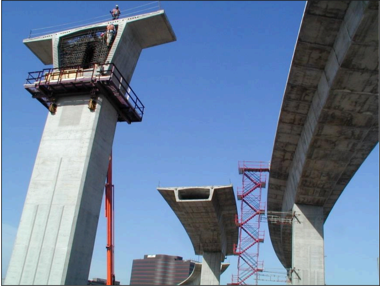
Figure 4.43 – Installation of Supplemental Rebar Inside Precast Shell, Dallas High-5, TX (Photo Courtesy of Zachry-Rizzani, JV)
