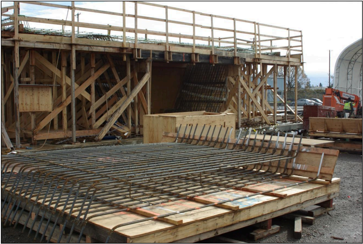
Figure 9.28 – Rebar Jig in Use with Wall Component Jig in Foreground (Photo Courtesy of Atkinson Construction)
