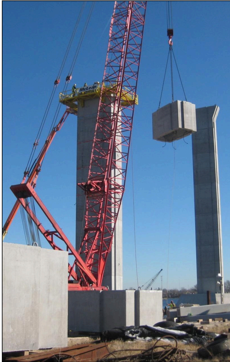
Figure 8.10 – Pier Column Segment Erection, South Norfolk Jordan Bridge, VA (Photo Courtesy of FIGG)
