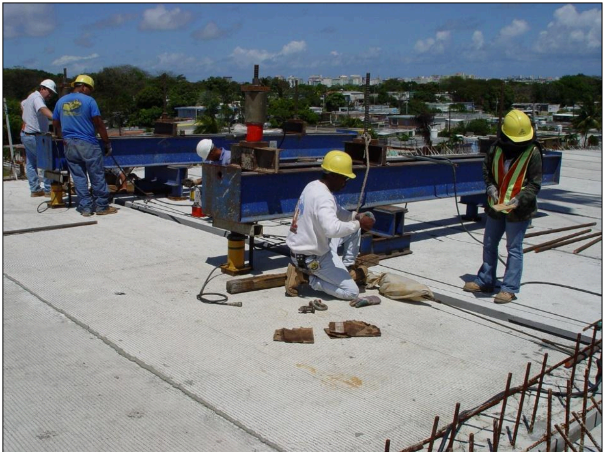
Figure 4.51 – Strongback Beams at Closure Joint Pour (Photo Courtesy of SYSTRA IBT)
