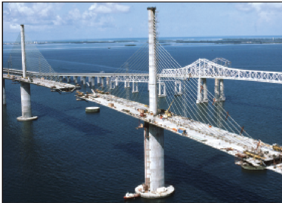
Figure 7.35 - Twin Wall Pier Pylon, Sunshine Skyway, FL (Photo Courtesy of Figg and Muller Engineers)
