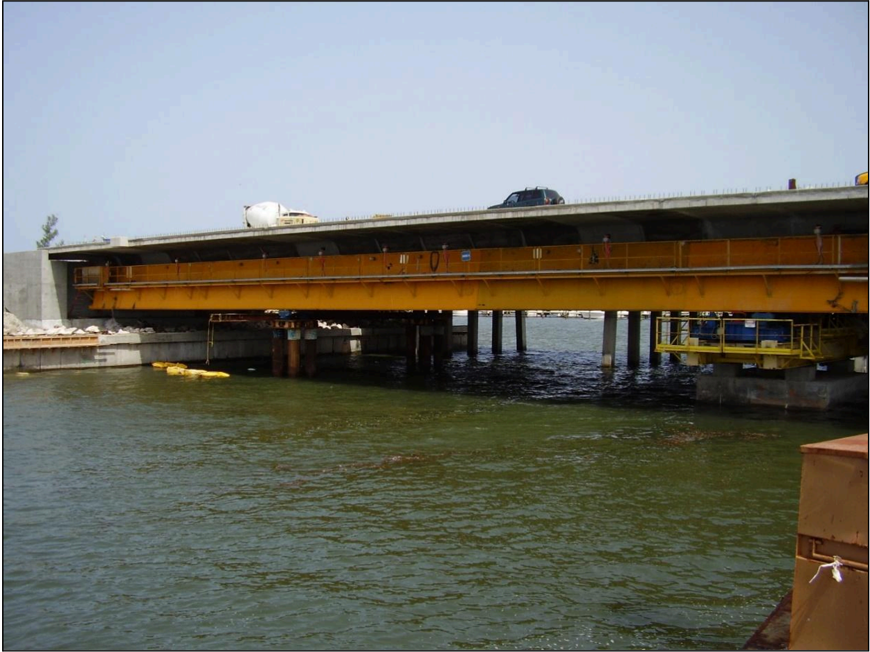
Figure 3.28 – Typical Conditions of Trusses After Erection of Final Span, Ernest F. Lyons Bridge, FL (Photo Courtesy of PCL Civil Constructors, Inc.)
