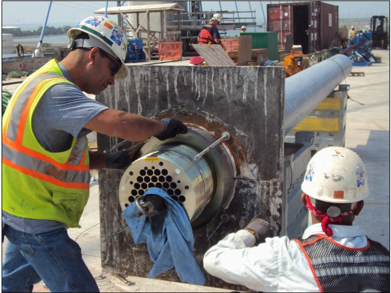
Figure 7.65 – Bearing Plate and Guide Pipe with Anchorage Installed (Photo Courtesy of AECOM)
