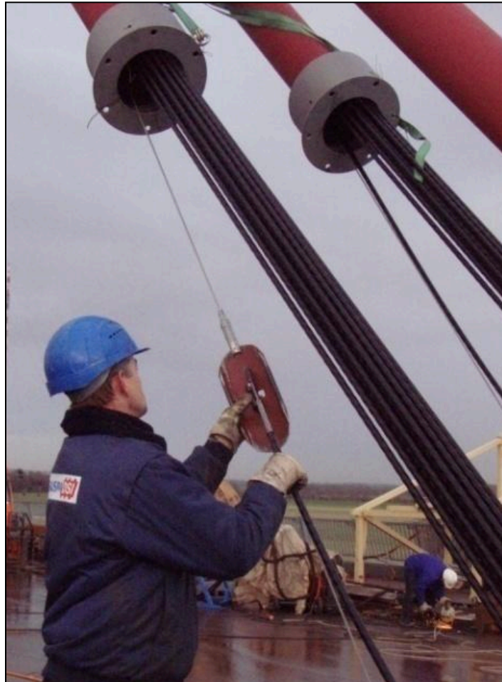
Figure 7.74 – Stay Cable Strand Being Connected to the Strand Shuttle (Photo Courtesy of SYSTRA IBT)
