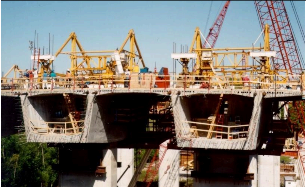
Figure 5.24 – Two single cell boxes cast together with four traveler frames, Creve Coeur Lake Memorial Bridge, MO (Photo Courtesy of Finley-McNary Engineers)
