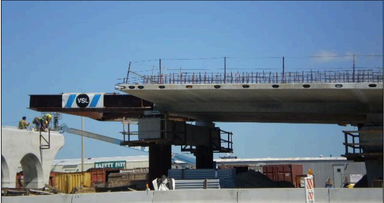
Figure 1.5 – Incremental Launch, Bellaire Beach Bridge, FL (Photo Courtesy of VSL)
