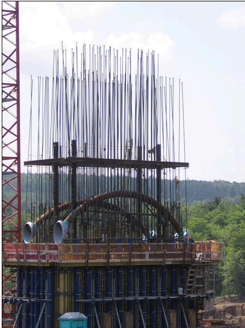
Figure 7.68 – Saddle (Cradle) Positioned in the Pylon (Photo Courtesy of FIGG)
