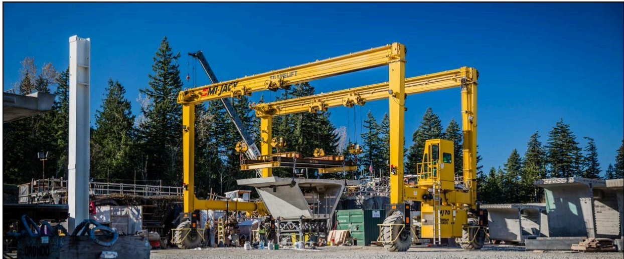
Figure 9.23 – Gantry Crane Handling Segment; RT Crane Servicing Bed (Photo Courtesy of Fueled Photography/PCL Civil Constructors, Inc.)
