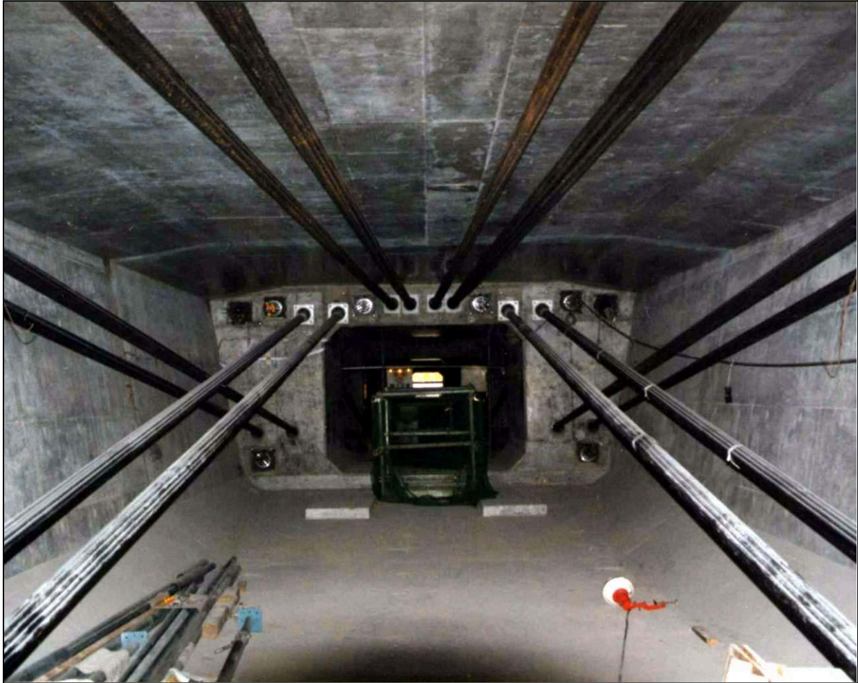
Figure 6.8 – Temporary (Launch) and Permanent External Tendons (Photo Courtesy of PSM Construction USA, Inc.)
