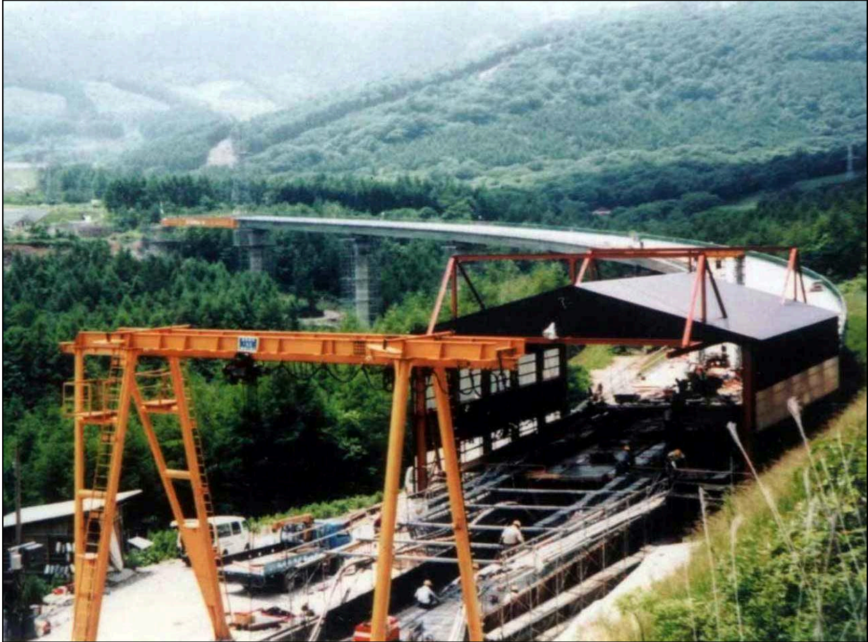
Figure 6.7 – Incremental Launching of a Bridge with Plan Curvature (Photo Courtesy of PSM Construction USA, Inc.)
