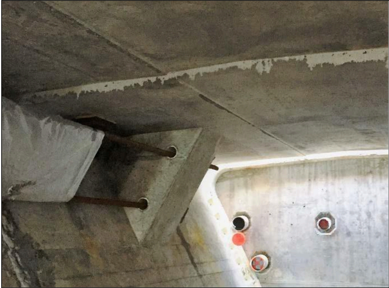
Figure 12.3 – Epoxy Squeeze Out After Application of Post-Tensioning Force (Photo Courtesy of RS&H)
