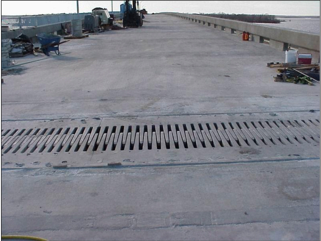
Figure 14.9 - Typical Finger Joint System in Place, Sailboat Bridge, OK (Photo Courtesy of FIGG)
