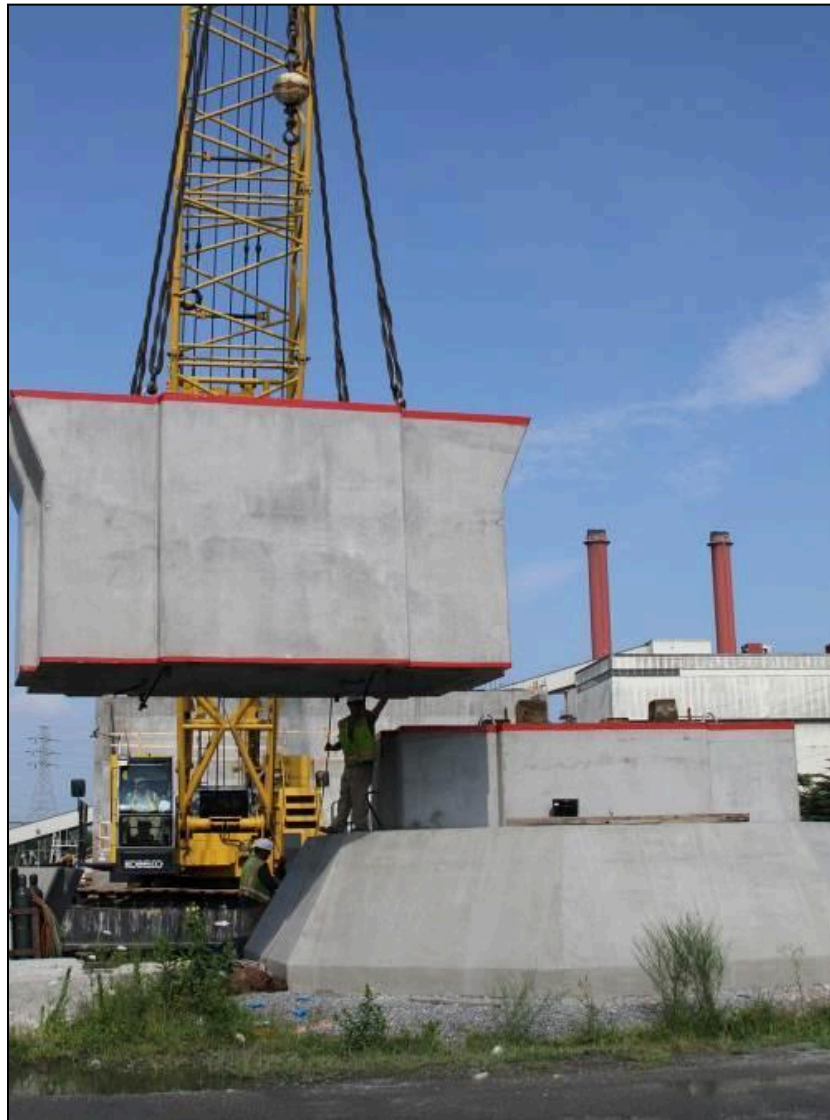
Figure 8.19 – Pier Column Erection with a Ground-Based Crane (Photo Courtesy of FIGG)
