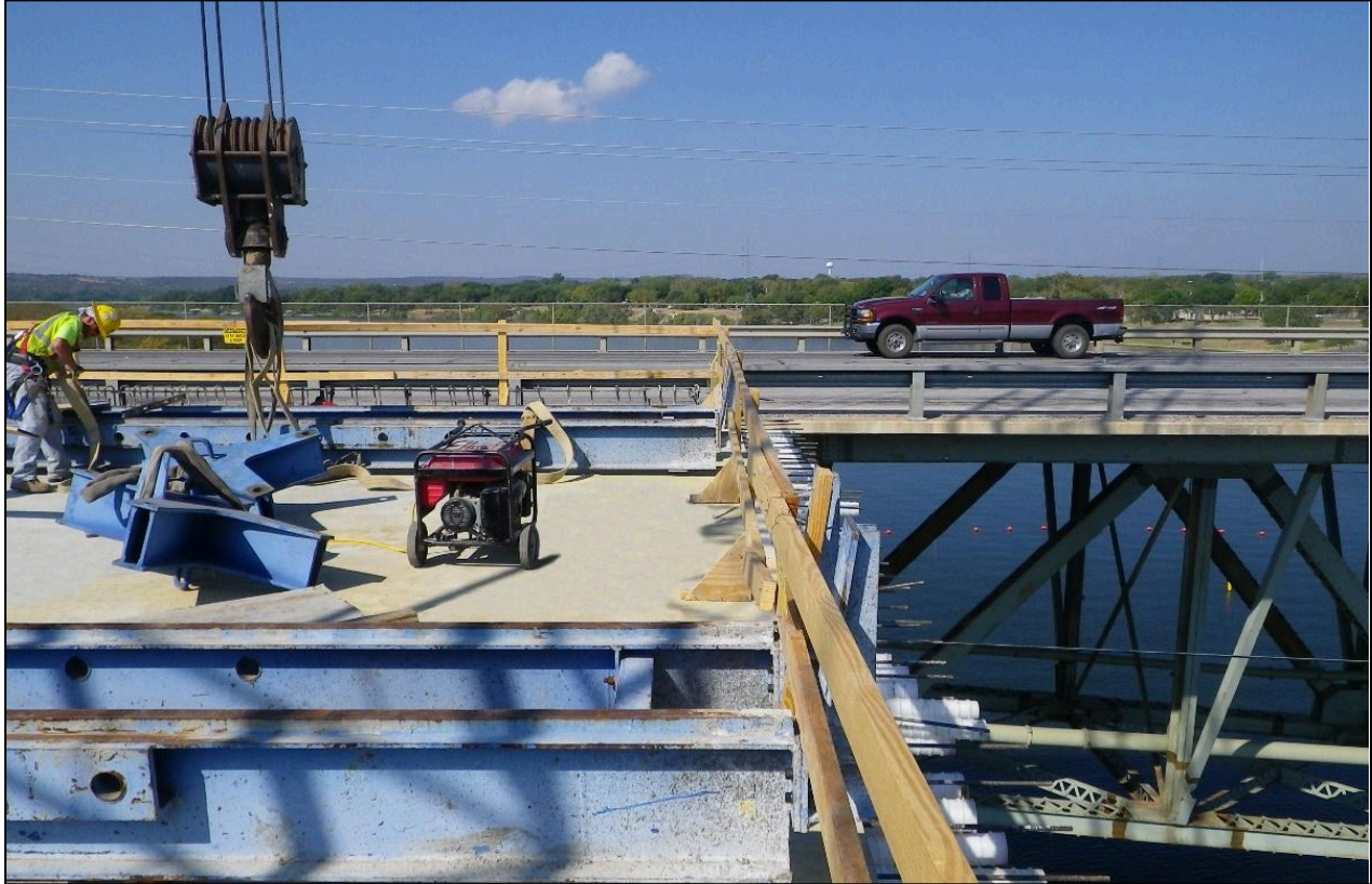
Figure 5.25 – Form Traveler Installation Step 1: Set Rails (Photo Courtesy of Archer Western)
