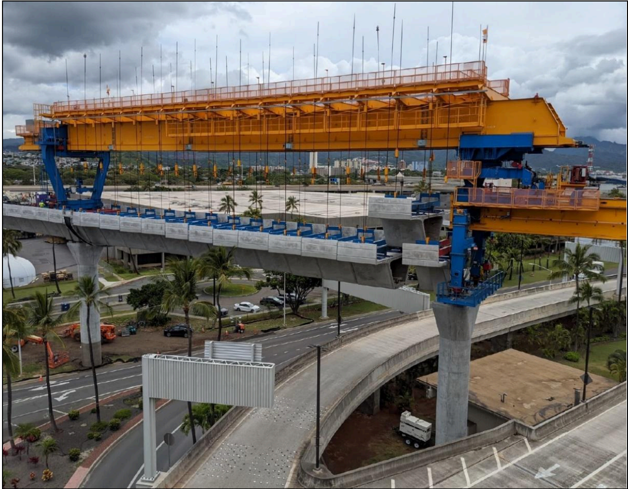
Figure 1.1 –Precast Span-by-Span, Honolulu Light Rail, HI (Photo Courtesy of Parsons)
