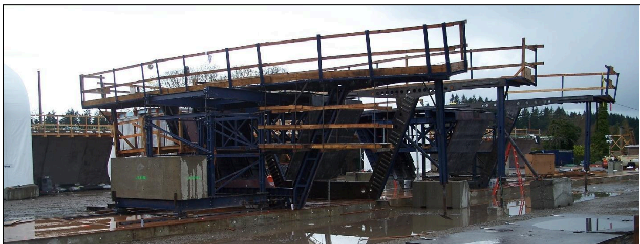
Figure 9.2 – Long-Line Bulkheads and Core Forms Being Erected for Starter Segments, SW Line Bridge, WA (Photo Courtesy of Atkinson Construction)
