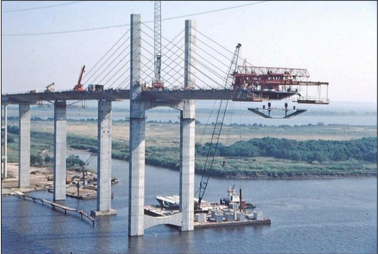
Figure 7.37 - Temporary Backspan Bent, Veterans Memorial Bridge, TX (Photo Courtesy of FIGG)
