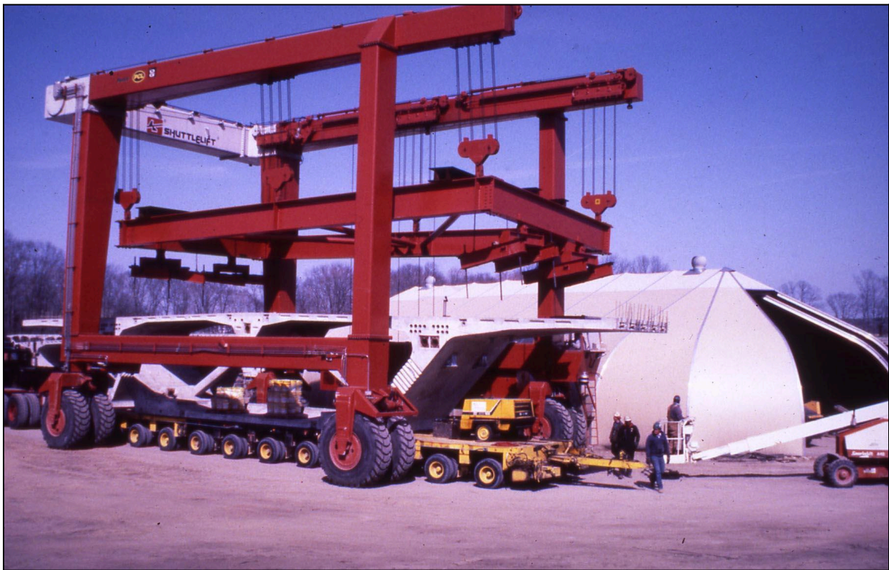
Figure 10.8 – Gantry Loading a Segment on a Segment Transport Vehicle, Baldwin Bridge, CT (Photo Courtesy of Perini/Homsi)
