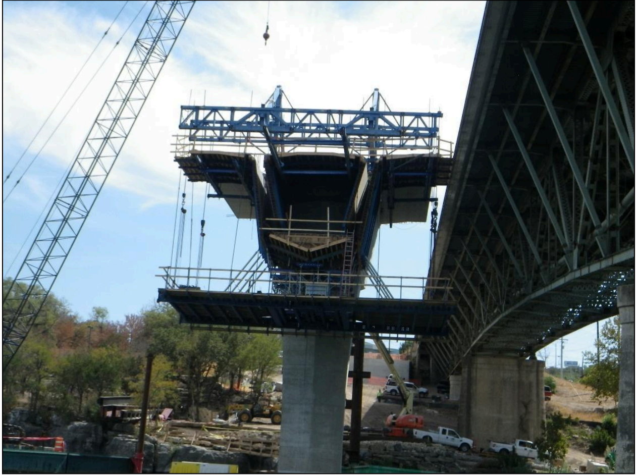
Figure 5.31 – Form Traveler Operation: Traveler and Formwork Assembled (Photo Courtesy of Archer Western)
