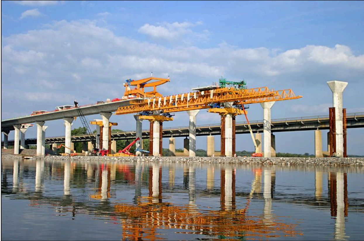
Figure 3.4 – Underslung Erection Truss Used in Top-Down Erection, Susquehanna River Bridge, PA (Photo Courtesy of FIGG)
