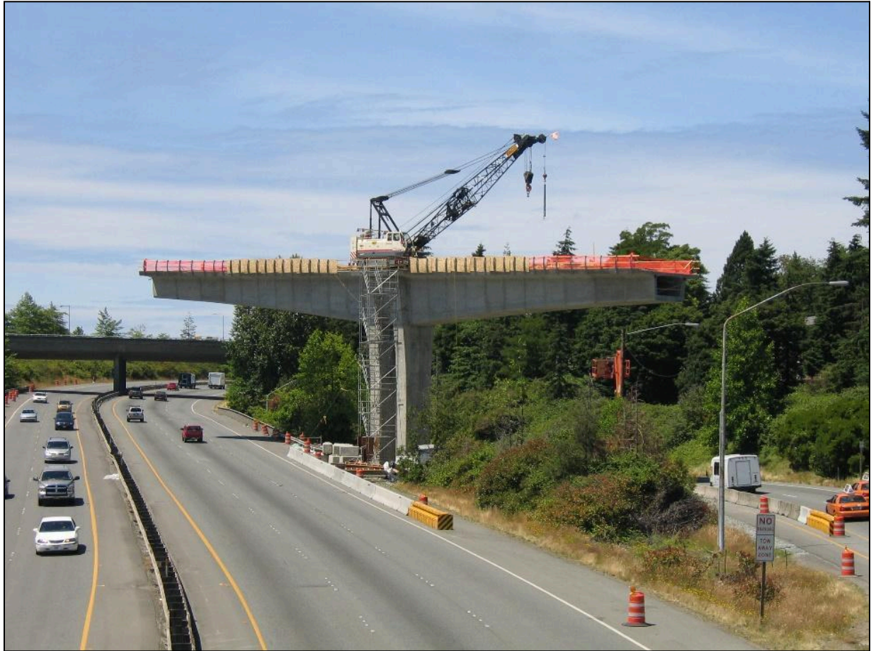
Figure 4.26 – Deck-Mounted Crane Erection, Sound Transit Tukwila Line, WA (Photo Courtesy of SYSTRA IBT)
