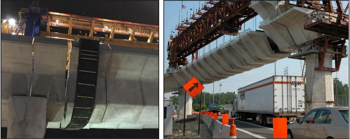
Figures 3.7 and 3.8 – Tarps Underneath the Segments During Epoxy Operations (Photos Courtesy of Traylor Bros. Inc. and FIGG)
