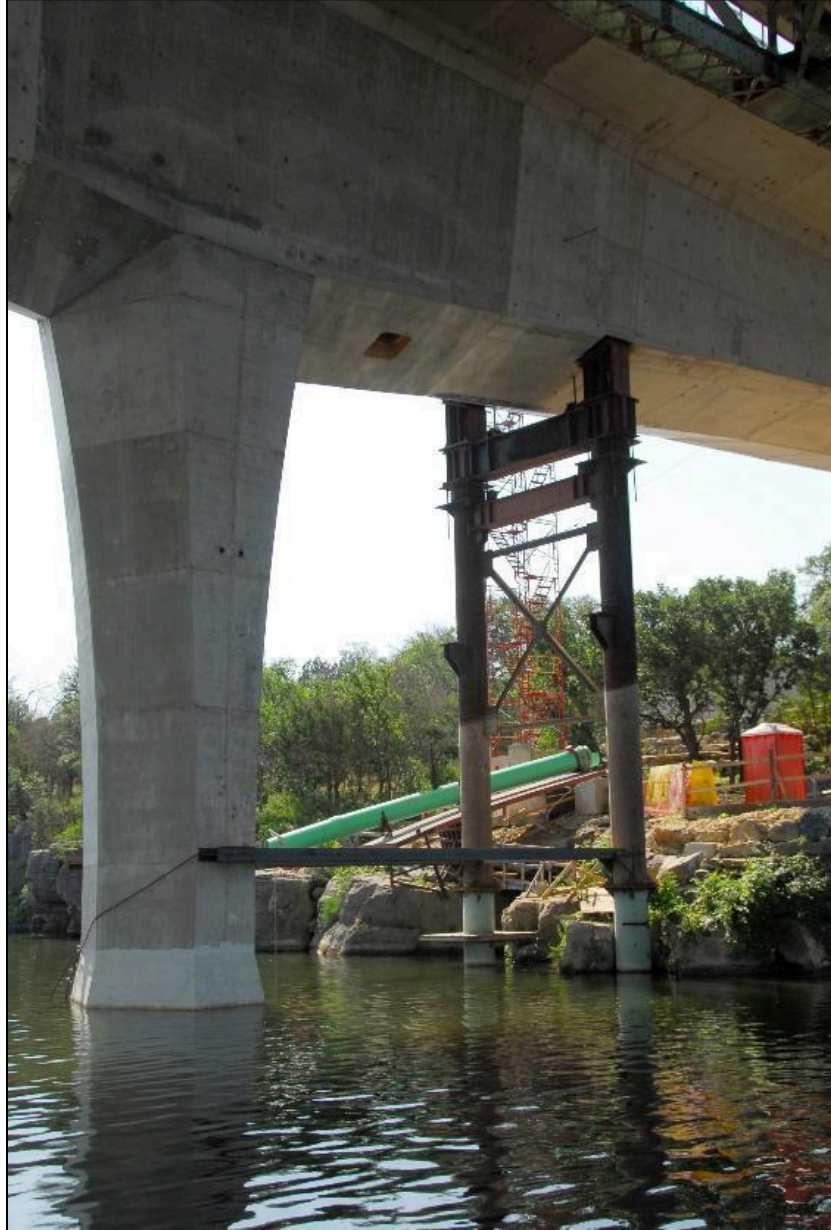
Figure 5.15 - Temporary support during construction for the US-281 Colorado River Bridge, Marble Falls, TX (Photo Courtesy of Archer Western)
