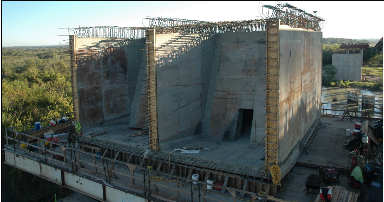
Figure 5.9 – Pier Table Web and Diaphragm Construction: Trinity River Bridge, TX (Photo Courtesy of Williams Brothers Construction)
