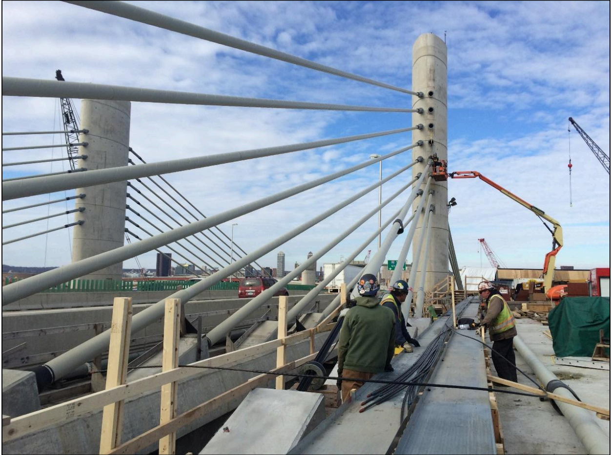
Figure 7.89 – Pearl Harbor Memorial Bridge, CT (Photo Courtesy of FIGG)
