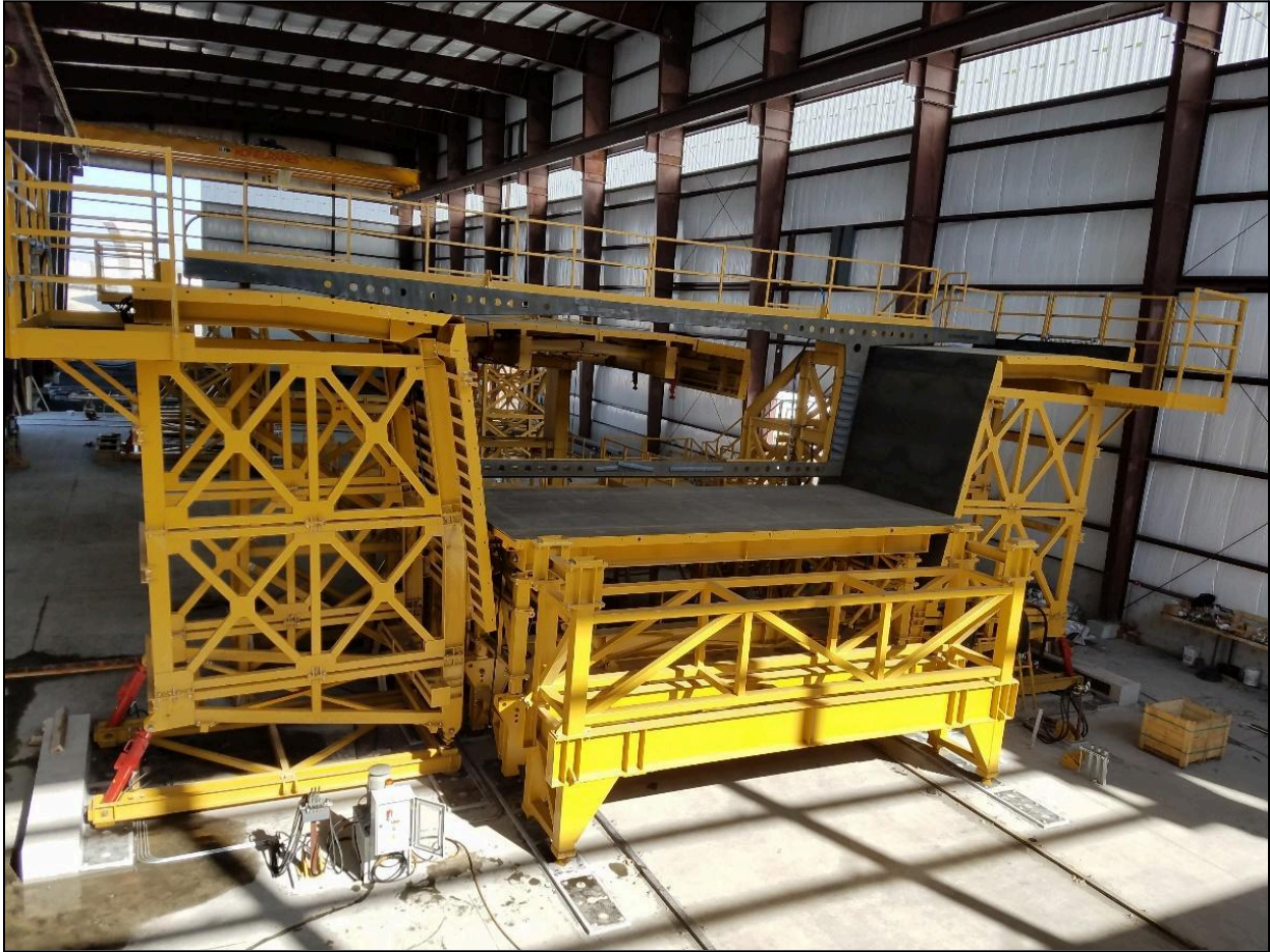
Figure 4.8 – Typical Form and Fixed Bulkhead (Photo Courtesy of FIGG)
