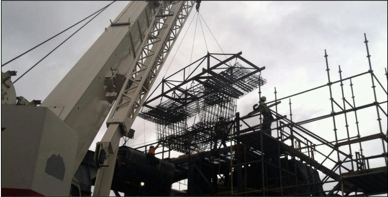
Figure 9.31 – Setting Rebar Cage in Oiled Casting Cell (Photo Courtesy of PCL Civil Constructors, Inc.)
