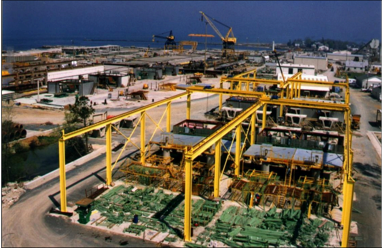
Figure 9.18 – Material Laydown Design is Critical for Productivity (Photo Courtesy of FIGG)
