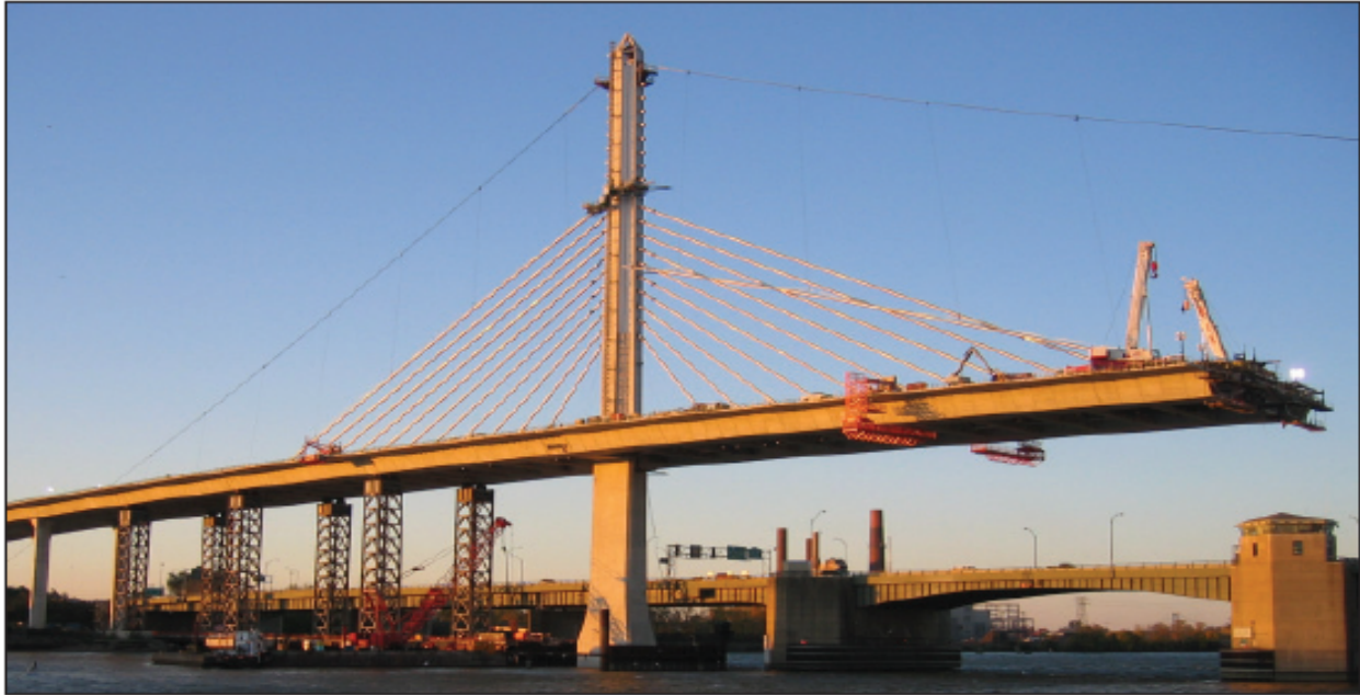
Figure 7.69 – Steel Pipe Erection with Highline, Veterans’ Glass City Skyway, OH (Photo Courtesy of Bilfinger & Berger)
