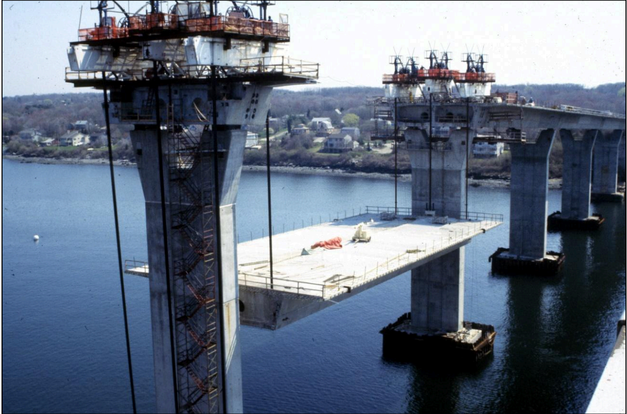
Figure 3.3 – Lifting an Entire Span, Jamestown-Verrazzano Bridge, RI (Photo Courtesy of FIGG)
