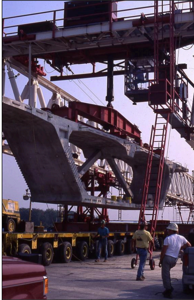
Figure 10.11 – Segment Being Lifted by the Launching Gantry, Baldwin Bridge, CT (Photo Courtesy of Perini/Homsi)
