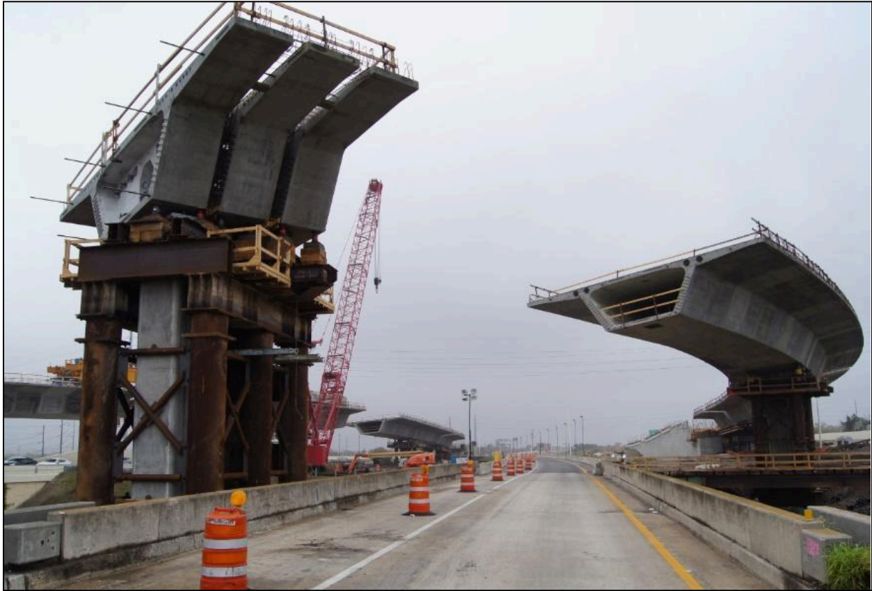
Figure 4.44 – Precast Segments with CIP Diaphragms, I-4 Connector Project, FL (Photo Courtesy of PCL/Archer-Western JV)
