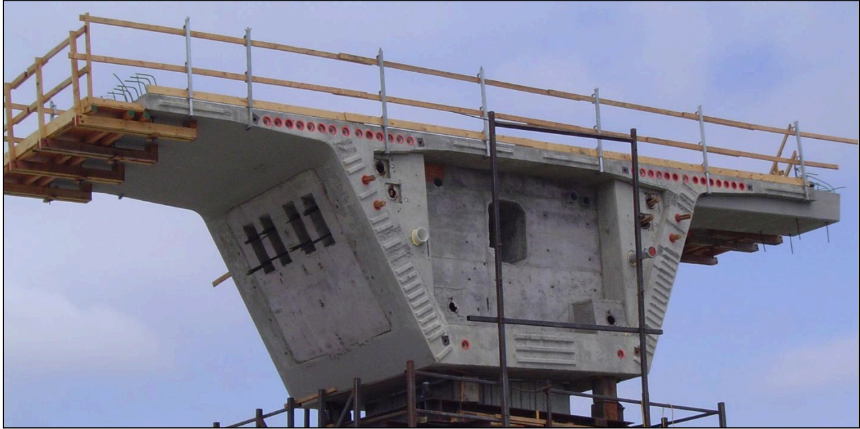
Figure 9.13 – Precast Pier Segment Shell Completed with Diaphragm [Note Transverse and Longitudinal Post-Tensioning] (Photo Courtesy of Atkinson Construction)
