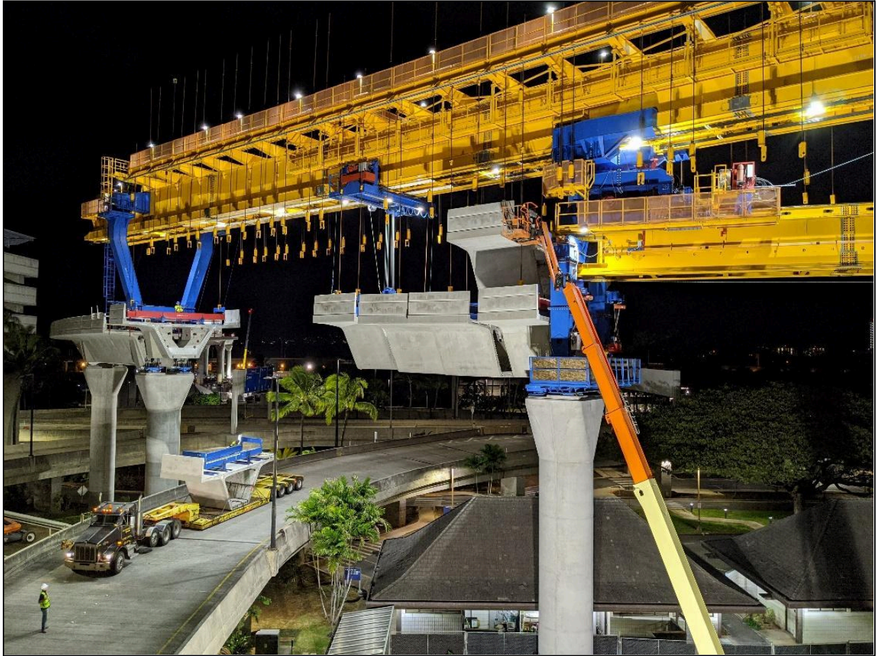
Figure 10.18 – Span-by-Span Overhead Gantry Segment Erection, Honolulu Light Rail, HI (Photo Courtesy of Traylor Bros., Inc.)
