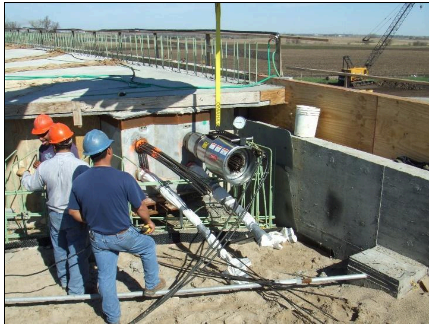
Figure 11.10 – Stressing Personnel Located Away from the Stressing Ram (Photo Courtesy of DYWIDAG Systems International)
