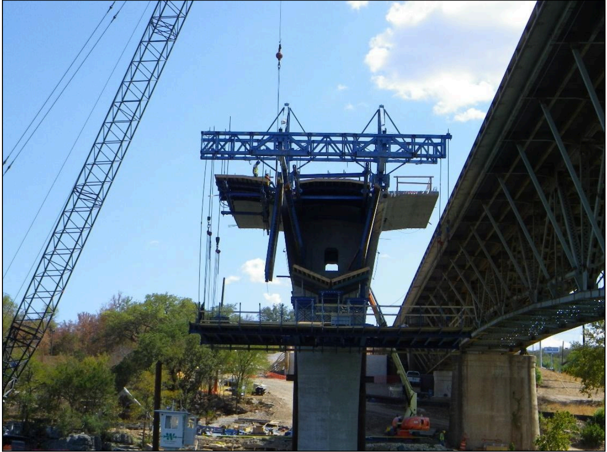
Figure 5.30 – Form Traveler Installation Step 6: Set Outer Wings and Formwork (Photo Courtesy of Archer Western)
