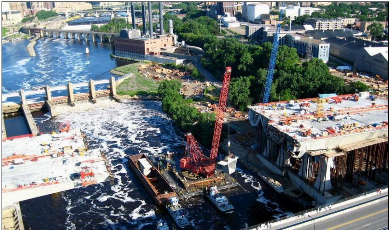
Figure 4.1 – Uni-Directional Cantilever Erection (Photo Courtesy of FIGG)
