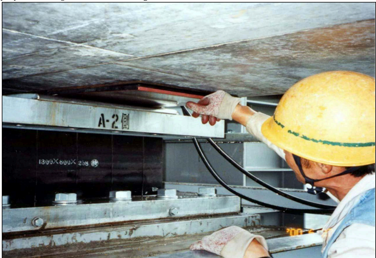
Figure 6.19 – Permanent Bearing Which Serves as Launch Bearing (Photo Courtesy of PSM Construction USA, Inc.)
