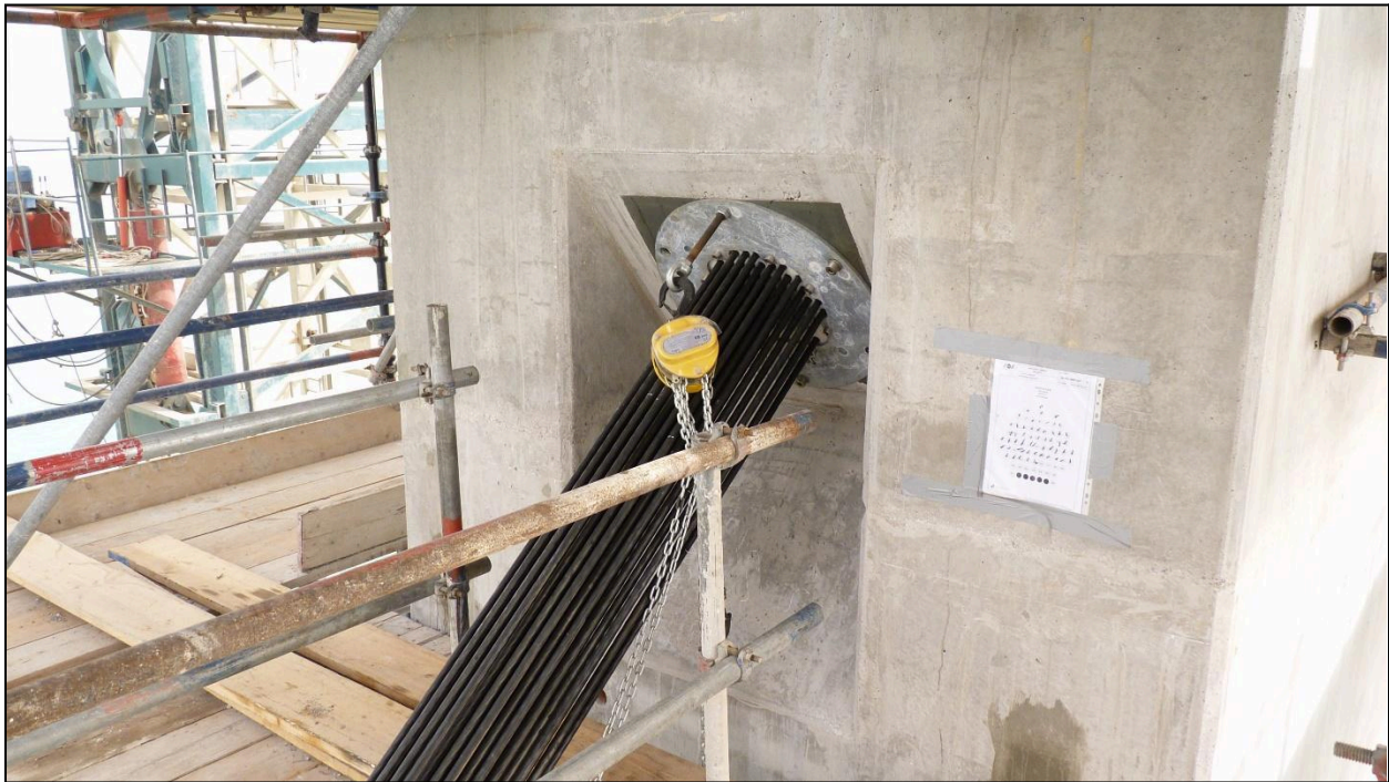
Figure 7.43 – Saddle in Pylon with Stay Cable Strands Exiting Saddle, Hodariyat Bridge, Abu Dhabi (Photo Courtesy of VSL)
