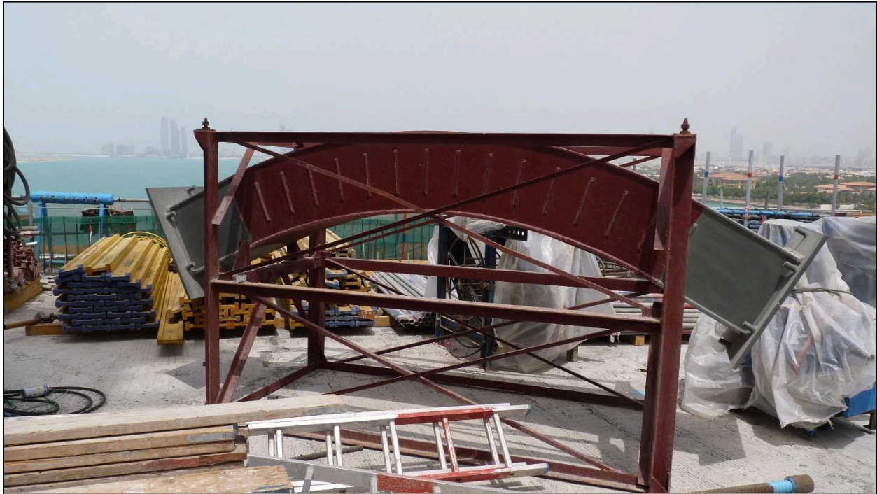
Figure 7.42 – Prefabricated Saddle, Hodariyat Bridge, Abu Dhabi (Photo Courtesy of VSL)
