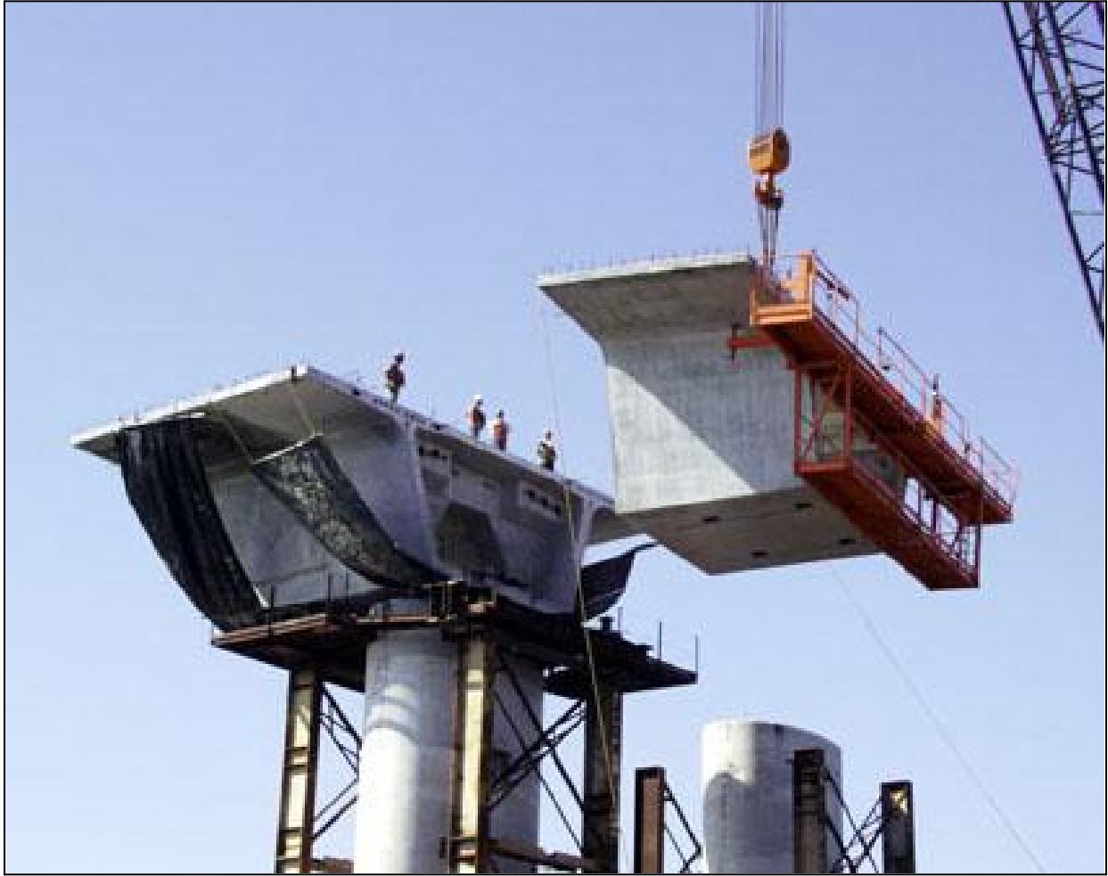
Figure 10.25 - Balanced-Cantilever Erection by Crane (Photo Courtesy of Flatiron Constructors, Inc.)
