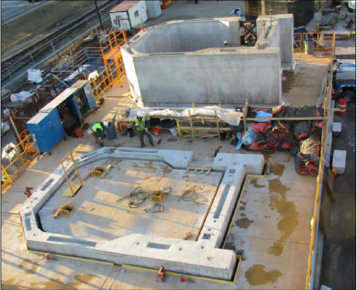
Figure 8.15 – Match-Cast Pier Column Segment During Precasting Operations (Photo Courtesy of Cianbro)
