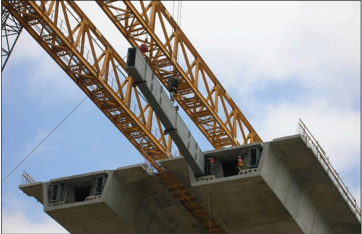
Figure 4.46 – Mid-Span Hinge Beam Installation, Otay River Bridge, CA (Photo Courtesy of SYSTRA IBT)
