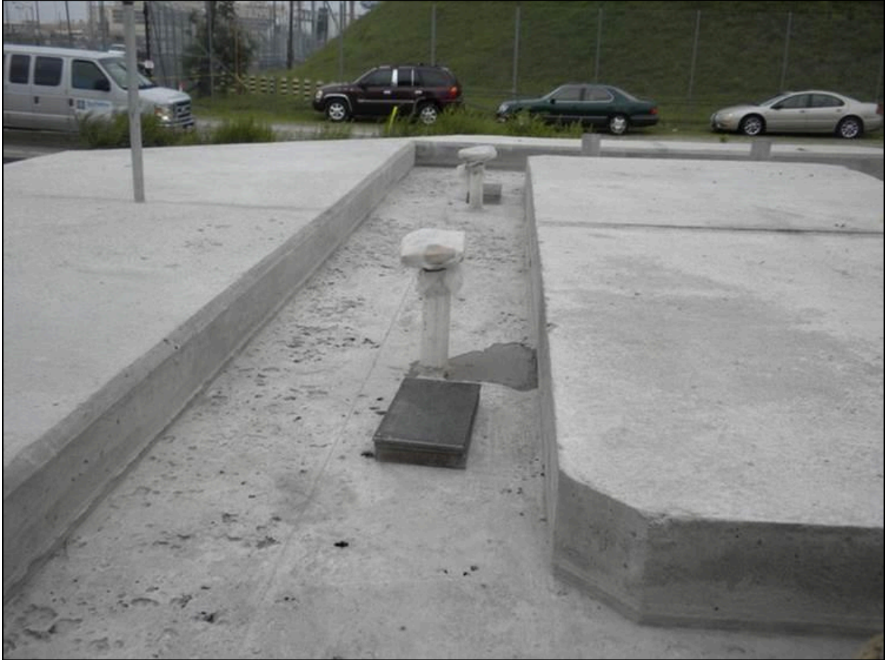
Figure 8.17 – Footing with Keyway (Photo Courtesy of FIGG)
