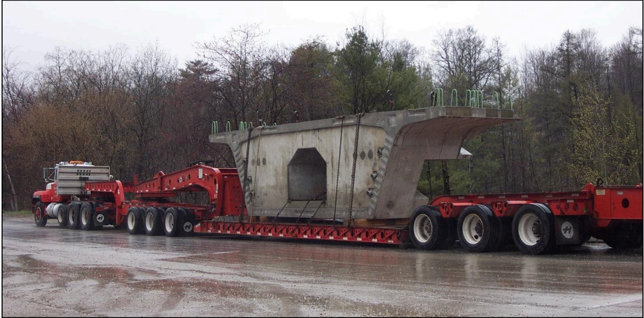
Figure 10.12 – Delivery of an 85-Ton Diaphragm Segment (note barrier wall rebar height), Boston Central Artery Project, MA (Photo Courtesy of Unistress Corporation)
