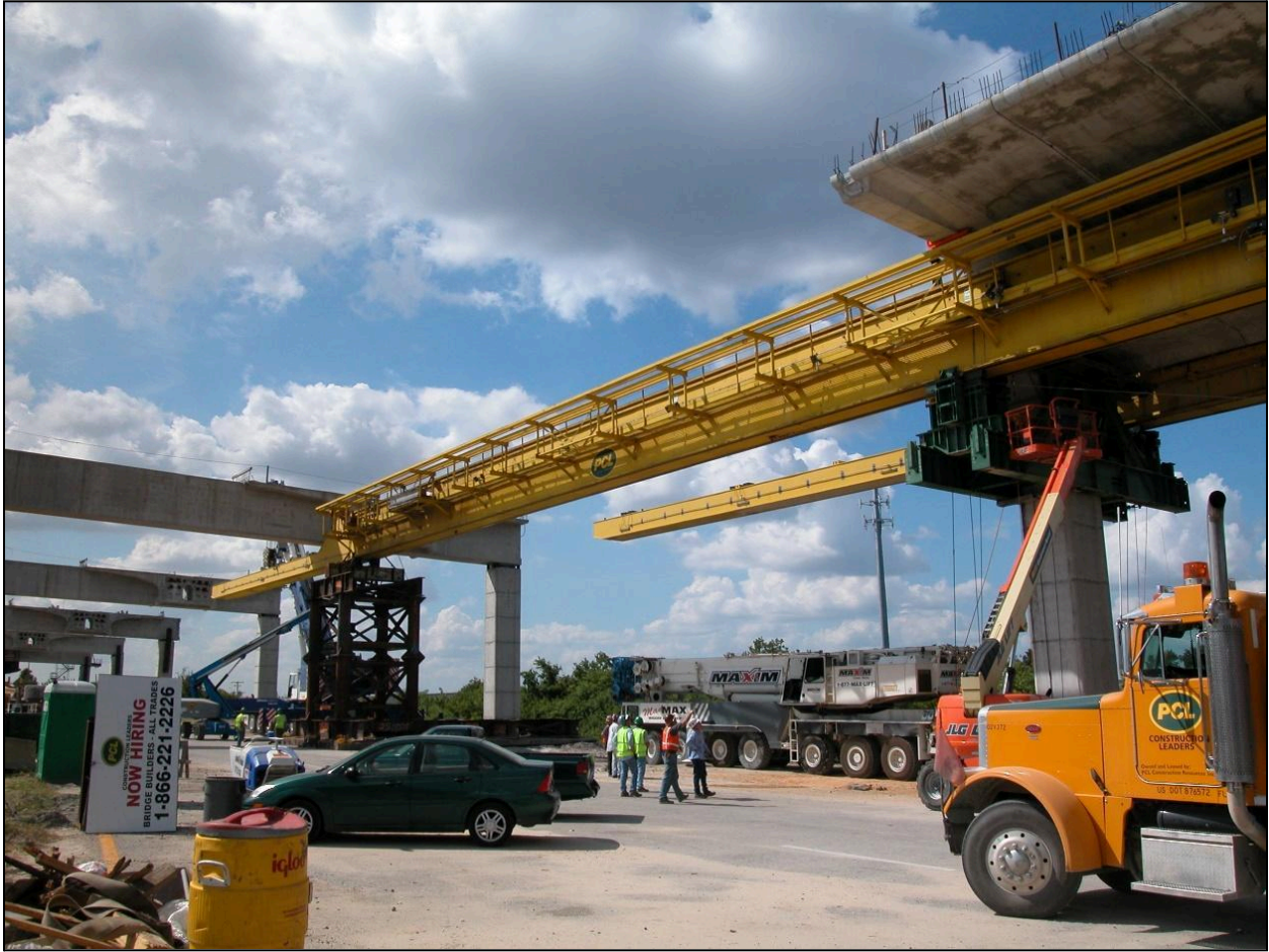
Figure 3.13 – Underslung Truss Advancing into Span to be Erected, Lee Roy Selmon Crosstown Expressway, FL (Photo Courtesy of FIGG)
