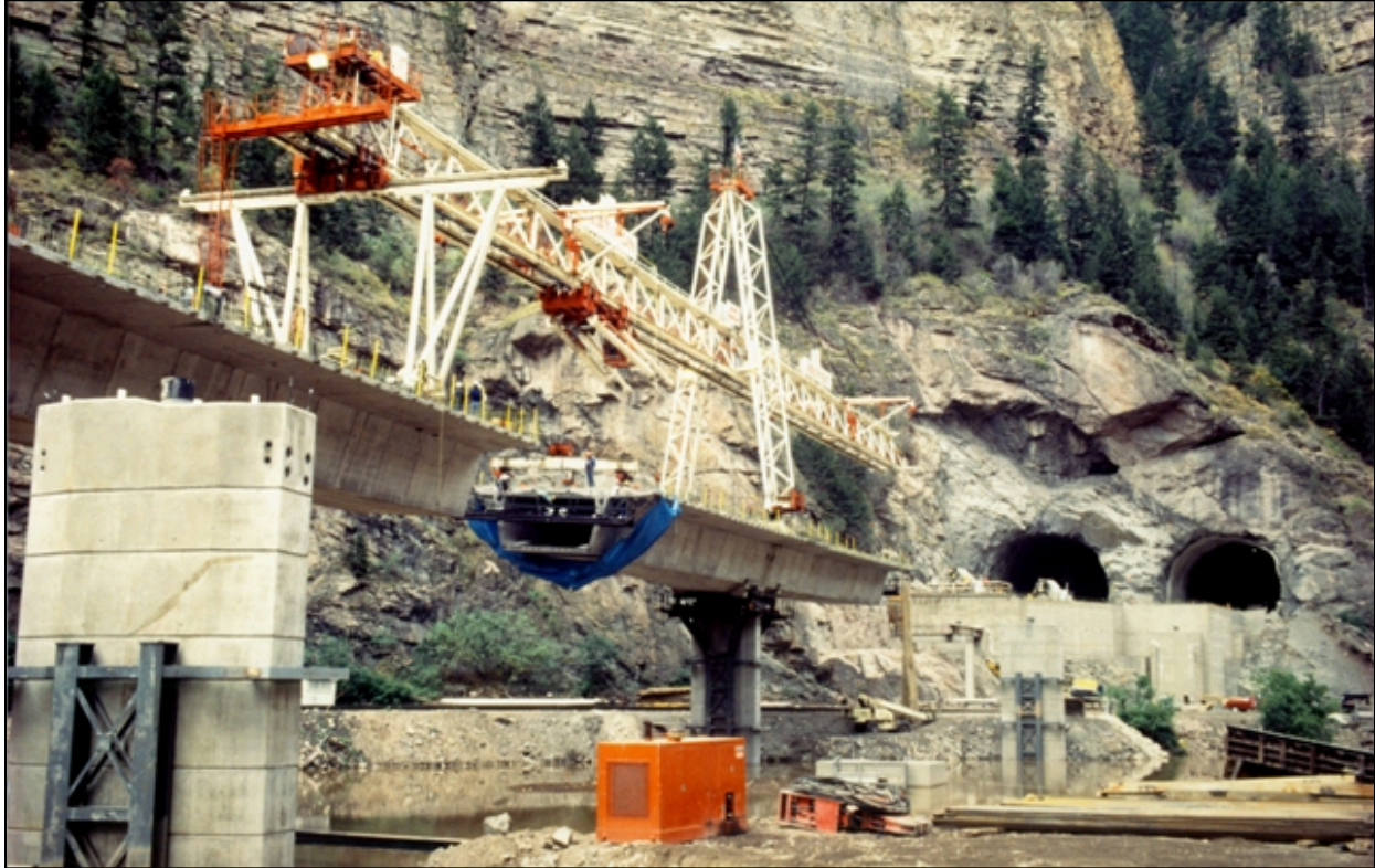
Figure 4.34– Launching Gantry, Hanging Lake Viaduct, Glenwood Canyon, CO (Photo Courtesy of Flatiron Constructors, Inc.)
