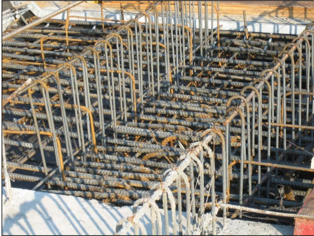
Figure 9.43 - Plinth Steel Added to the Rebar Cage (Photo Courtesy of Fueled Photography/PCL Civil Constructors, Inc.)
