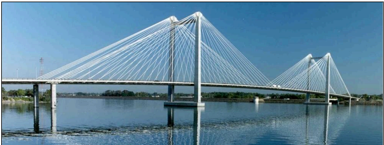
Figure 7.3 – Pasco-Kennewick Bridge, Washington (Photo Courtesy of Washington DOT)
