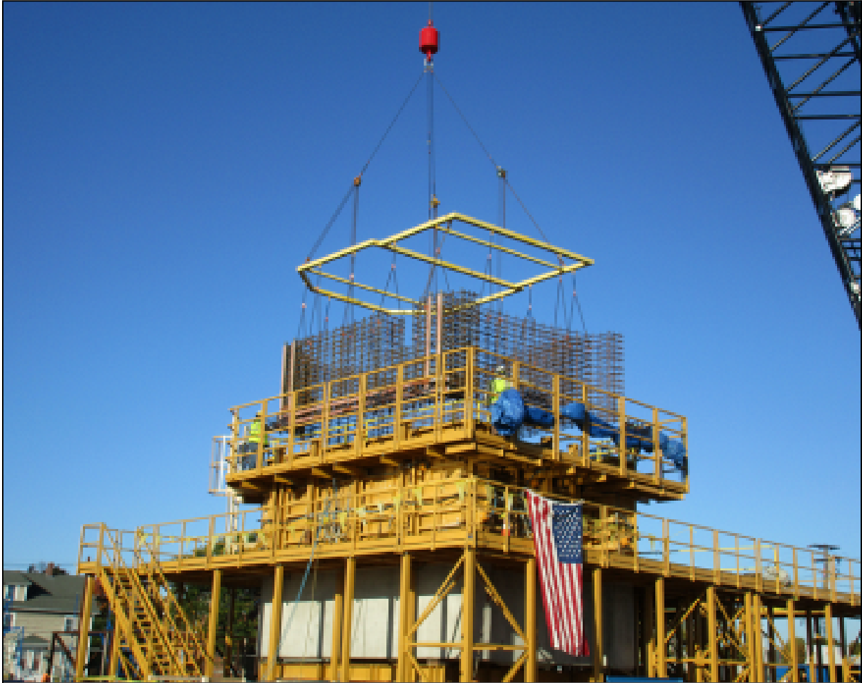
Figure 8.14 – Precast Column Segment Reinforcing Cage (Photo Courtesy of Cianbro)
