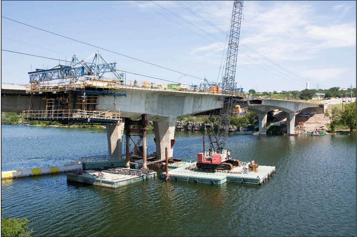
Figure 5.18 – Monolithic Column Superstructure Connection, US-281 Colorado River Bridge, TX (Photo Courtesy of Archer Western)
