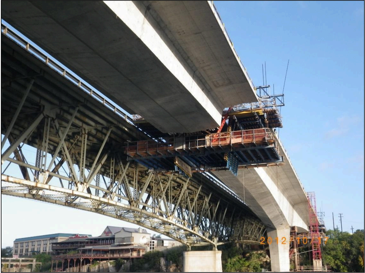
Figure 5.32 – Form Traveler Operation: Nearing Mid-Span Closure (Photo Courtesy of Archer Western)
