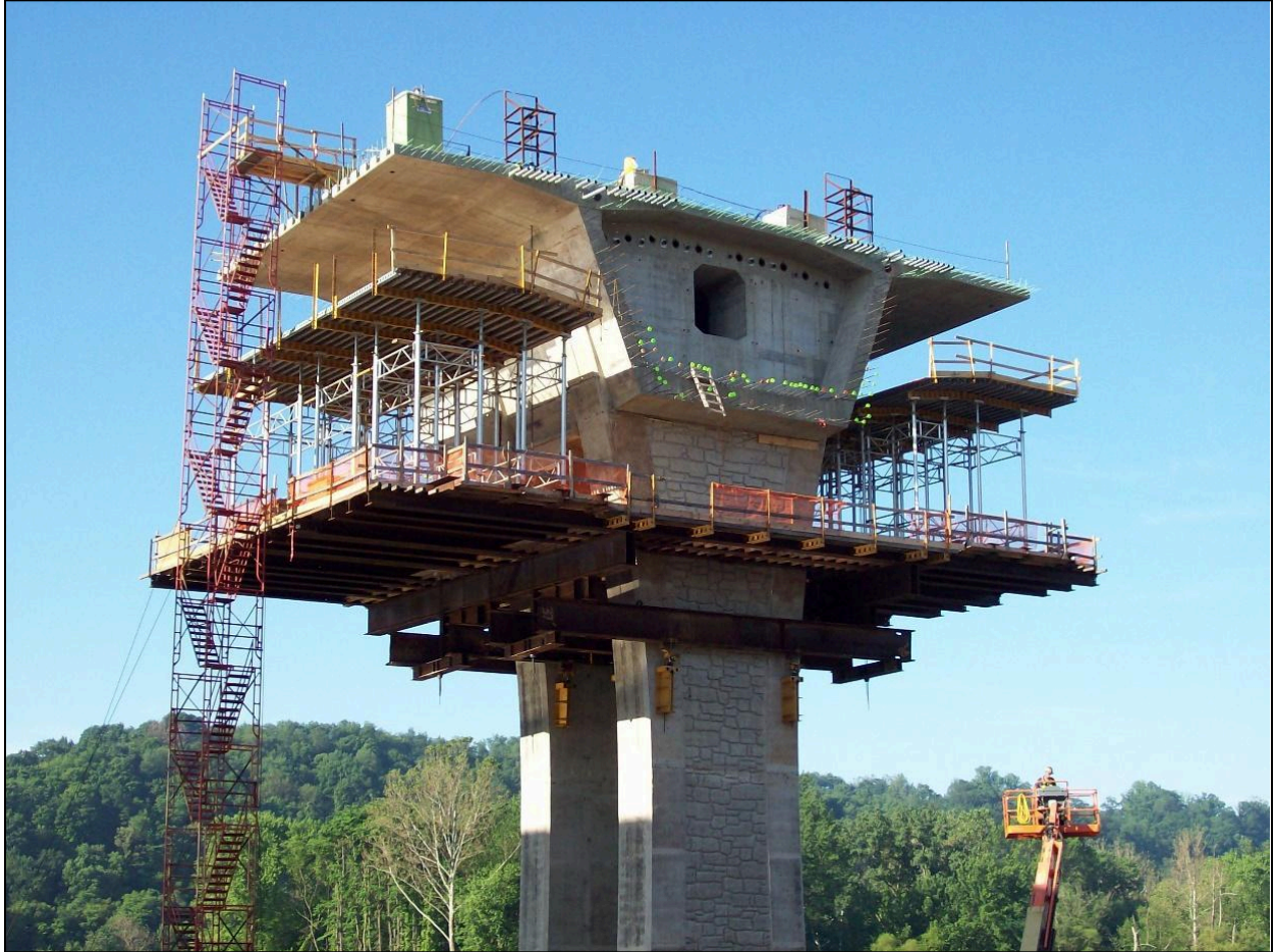
Figure 5.17 – Double-Walled Pier Superstructure Connection, Allegheny River Bridge, PA (Photo Courtesy of FIGG)
