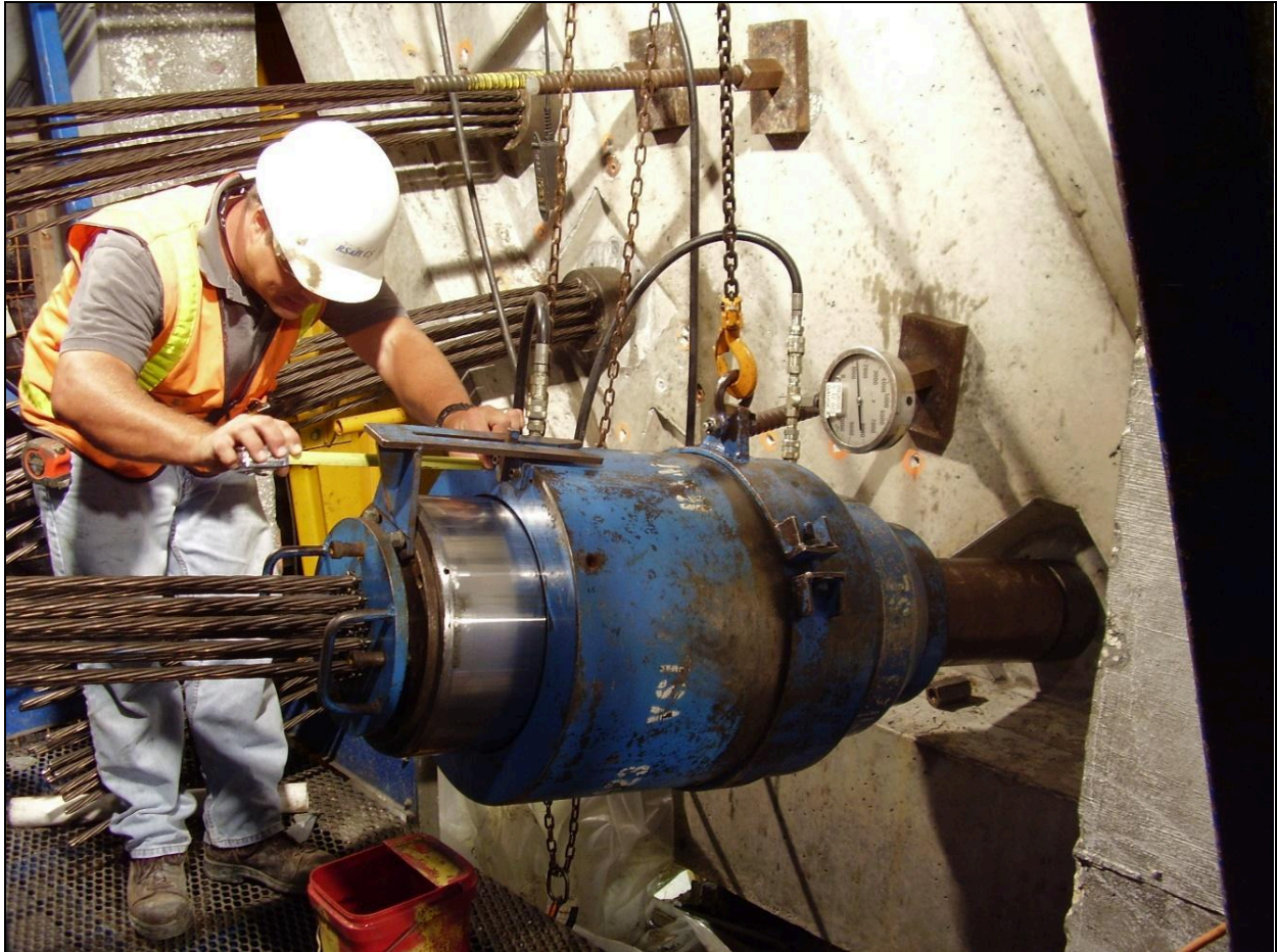
Figure 3.23 – Stressing Permanent Post-Tensioning (Photo Courtesy of PCL Civil Constructors, Inc.)
