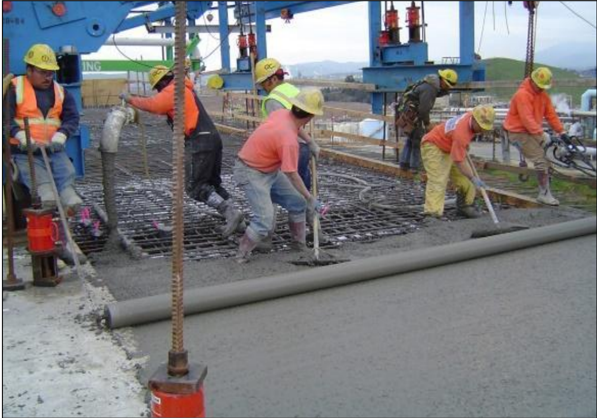
Figure 5.45 – Finishing top deck concrete placement. (Photo Courtesy of Kiewit)
