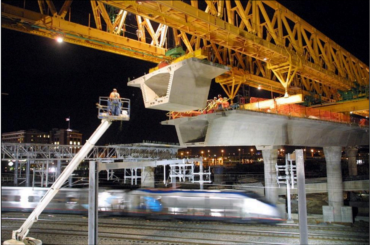
Figure 10.29 – Balanced-Cantilever Erection by Overhead Gantry (Photo Courtesy of Flatiron Constructors, Inc.)
