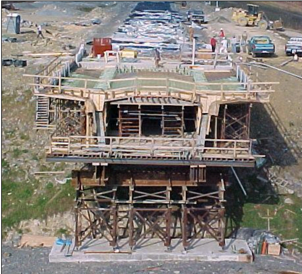
Figure 5.47 - Abutment Segment Under Construction with the Falsework in Place (Photo Courtesy of Archer Western)
