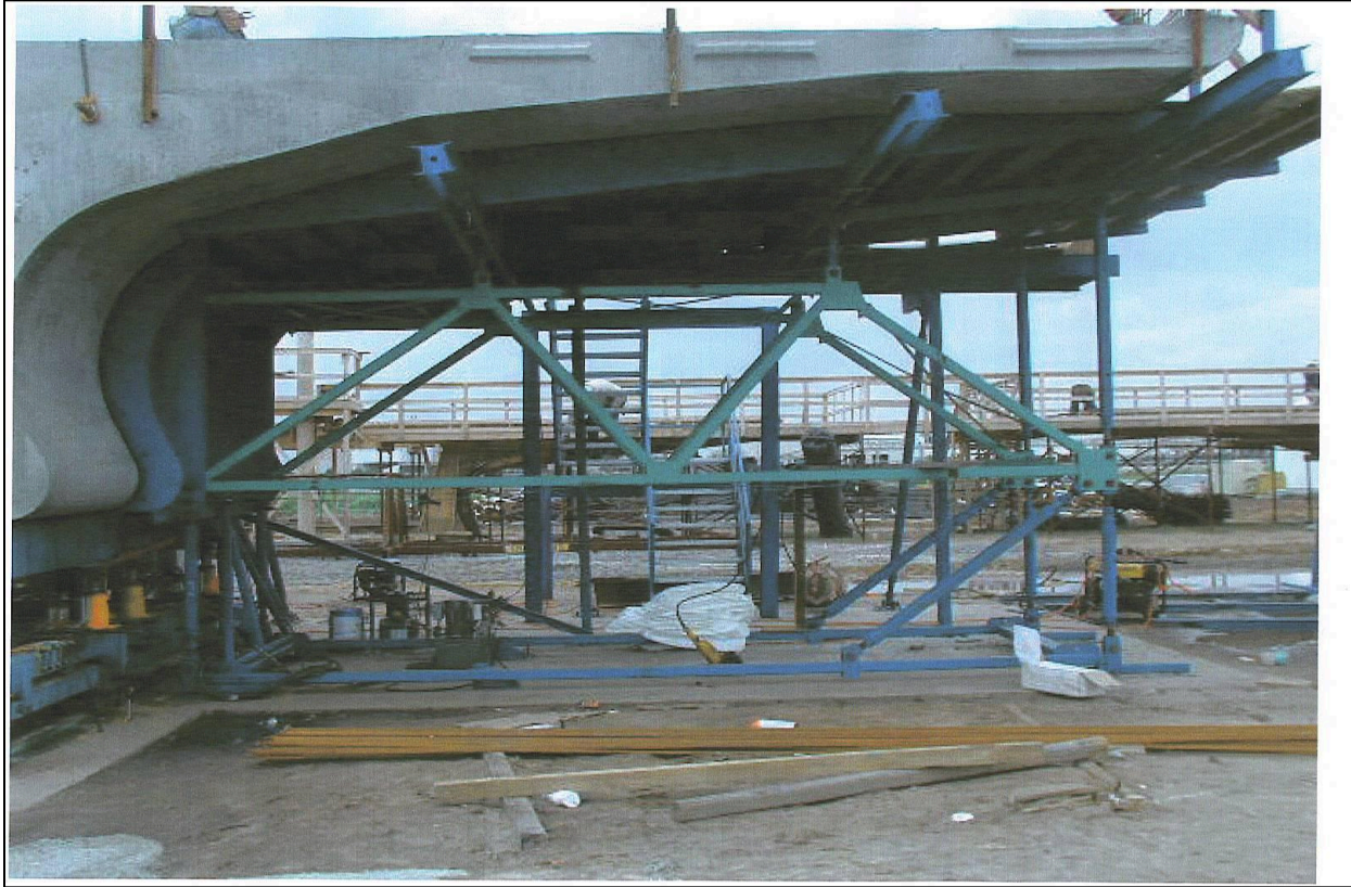
Figure 9.10 - Wing Form Supports, Lee Roy Selmon Crosstown Expressway, FL (Photo Courtesy of FIGG)
