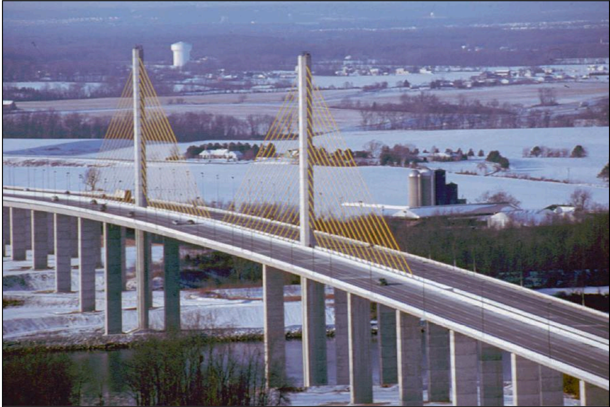
Figure 7.5 – Korean War Veterans Memorial Bridge, Delaware (Photo Courtesy of FIGG)
