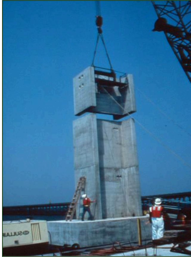
Figure 8.3 – Albemarle Sound Bridge Pier Column Segments, NC (Photo Courtesy of FIGG)
