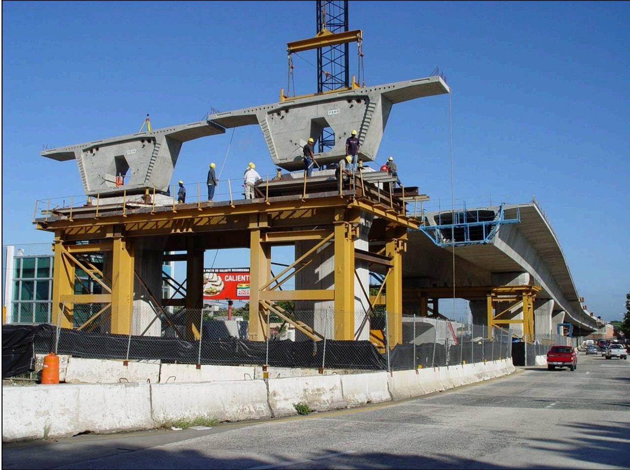
Figure 4.39 – Placing Precast Pier Segments, PR181 (Photo Courtesy of SYSTRA IBT)
