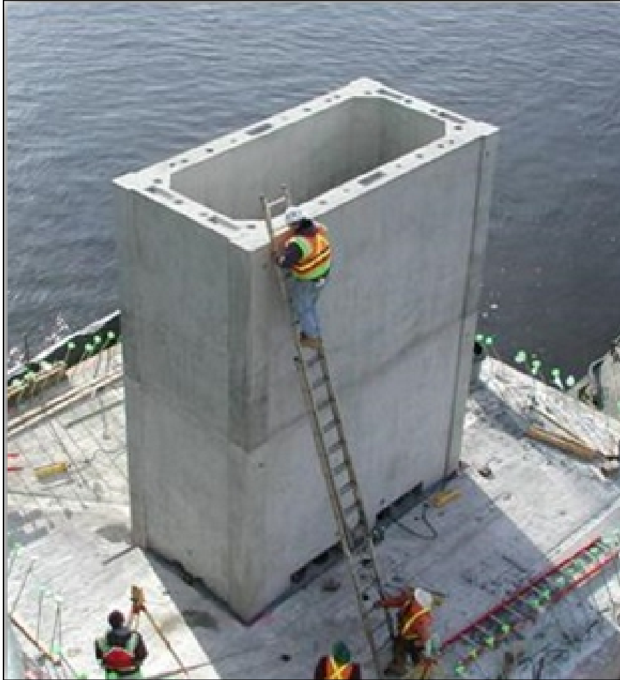
Figure 8.4 - Route 36 Highlands Bridge, NJ (Photo Courtesy of J.H. Reid General Contractors)
