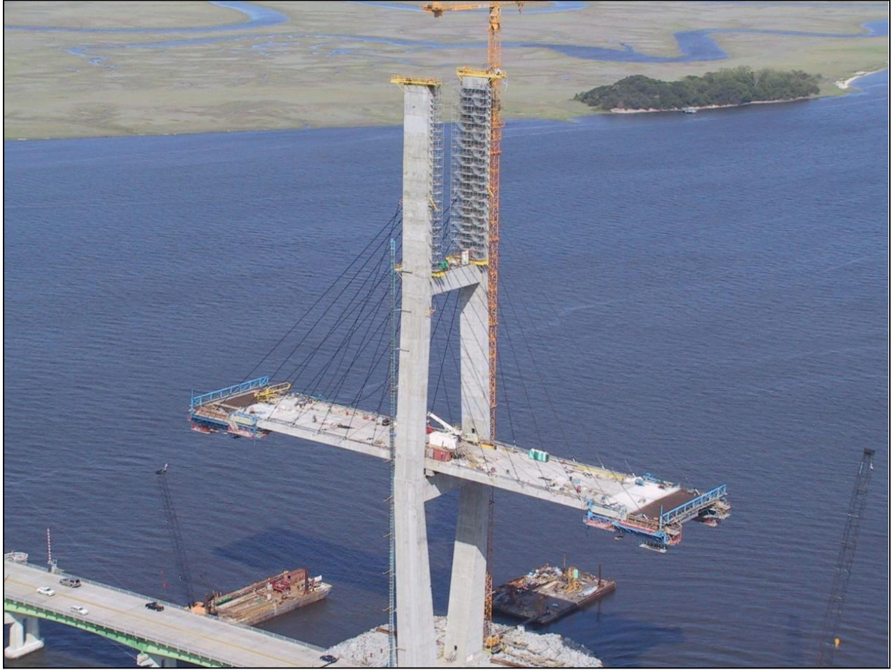
Figure 7.24 – Sidney Lanier Bridge, Georgia (Photo Courtesy of Bob Webster)
