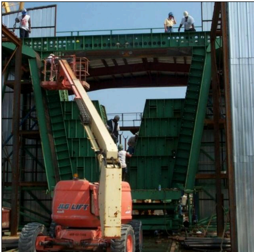
Figure 9.24 – Tall Segment Forms May Require an Aerial Personnel Lift (Photo Courtesy of FIGG)
