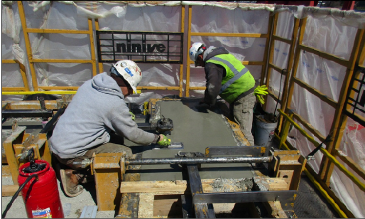
Figure 8.16 – Precast Column Segment Concrete Finishing (Photo Courtesy of Cianbro)
