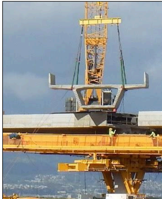
Figure 10.1-3 - Sling-Style Lifting Frame (Photo Courtesy of FIGG)
