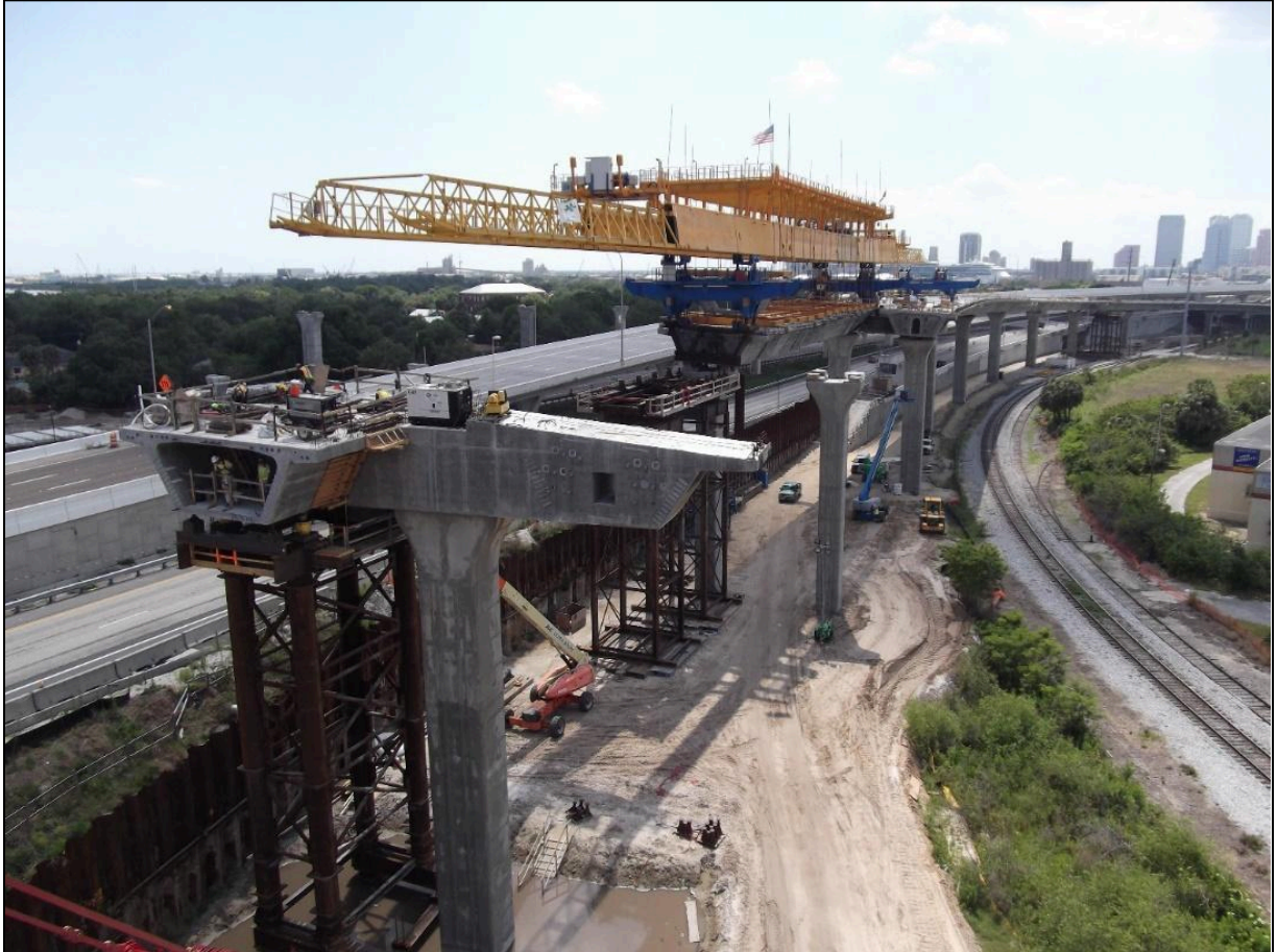
Figure 4.36 – Cast-in-Place Pier Segment, I-4 Connector Project, FL (Photo Courtesy of PCL/Archer-Western JV)
