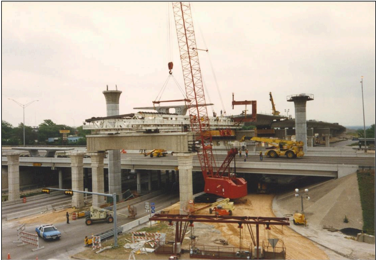
Figure 10.15 – Crane Erection of Span-by-Span Bridge on Underslung Trusses (Photo Courtesy of Flatiron Constructors, Inc.)
