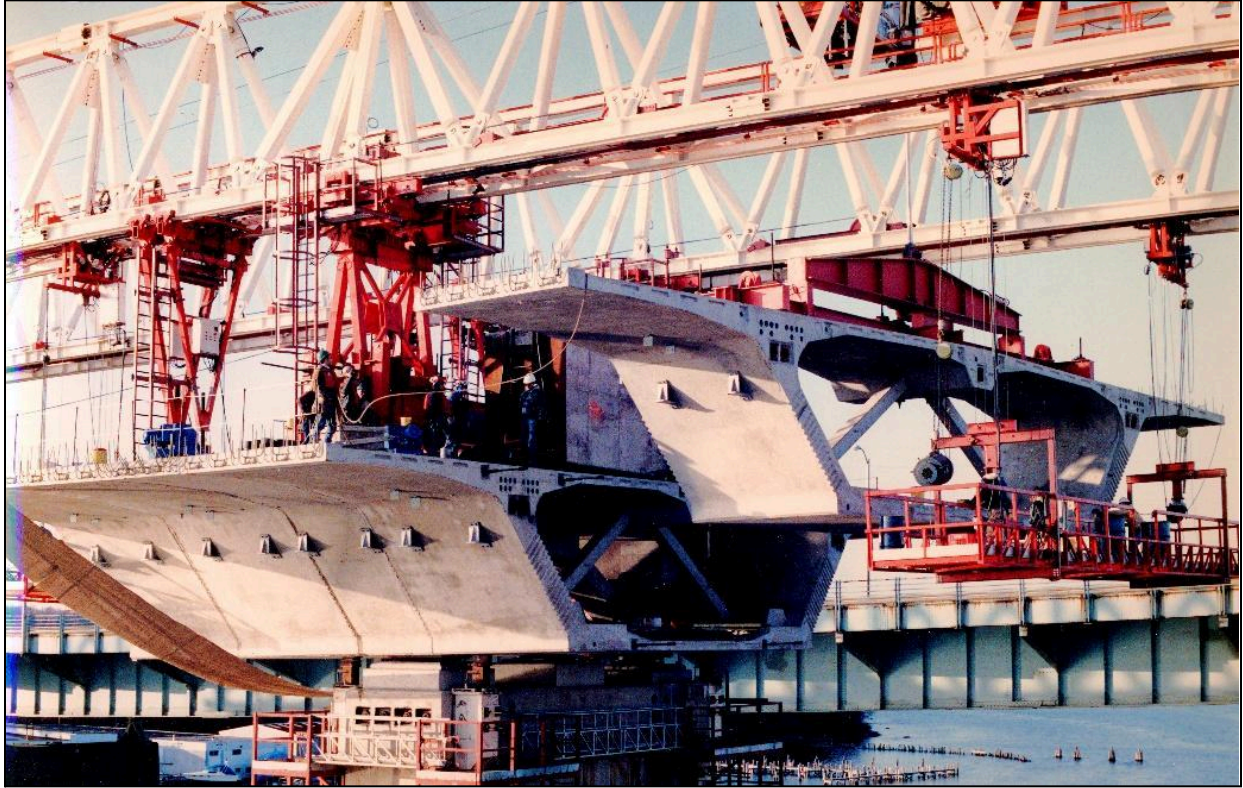
Figure 10.28 – Balanced-Cantilever Erection by Overhead Gantry (Photo Courtesy of Perini/Homsi)
