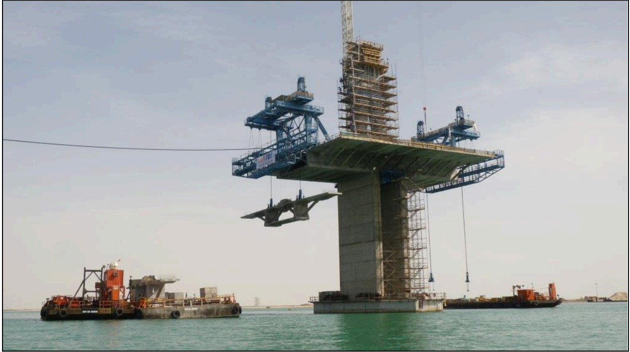
Figure 7.17 – Hodariyat Bridge, Abu Dhabi (Photo Courtesy of SYSTRA IBT)
