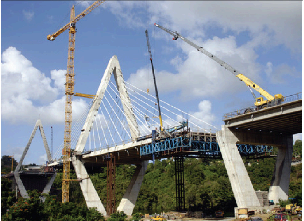
Figure 7.23 – CIP Edge Girder with Traveler, La Plata River Bridge, Puerto Rico (Photo Courtesy of Las Piedras Construction)
