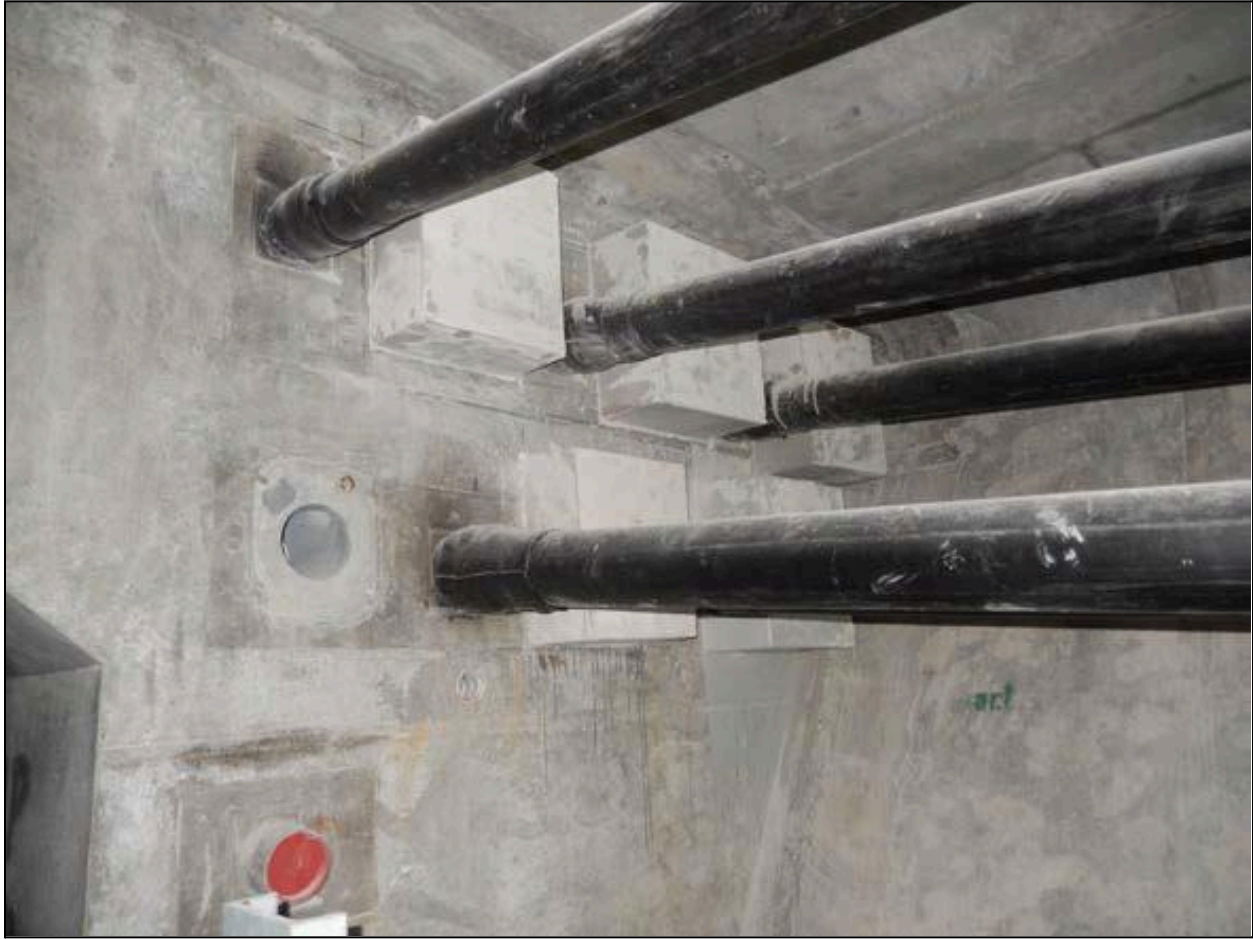
Figure 12.10 - Epoxy Grout Pourbacks for Anchorage Protection (Photo Courtesy of FIGG)
