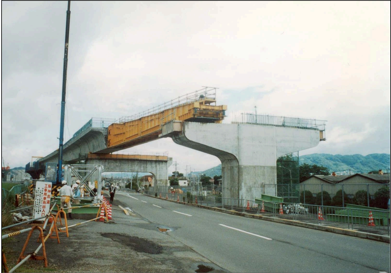
Figure 6.3 – Incremental Launching Over a Road – Japan (Photo Courtesy of PSM Construction USA, Inc.)
