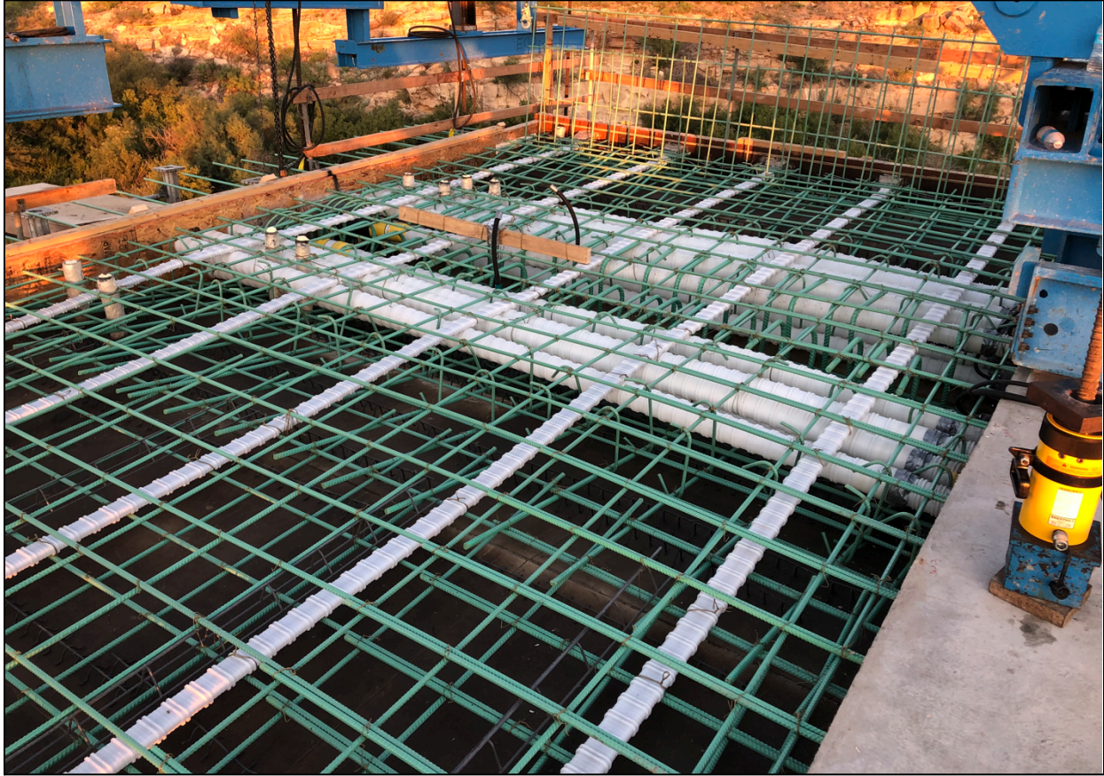
Figure 5.43 – Installing reinforcing for the top deck. (Photo Courtesy of NMDOT)
