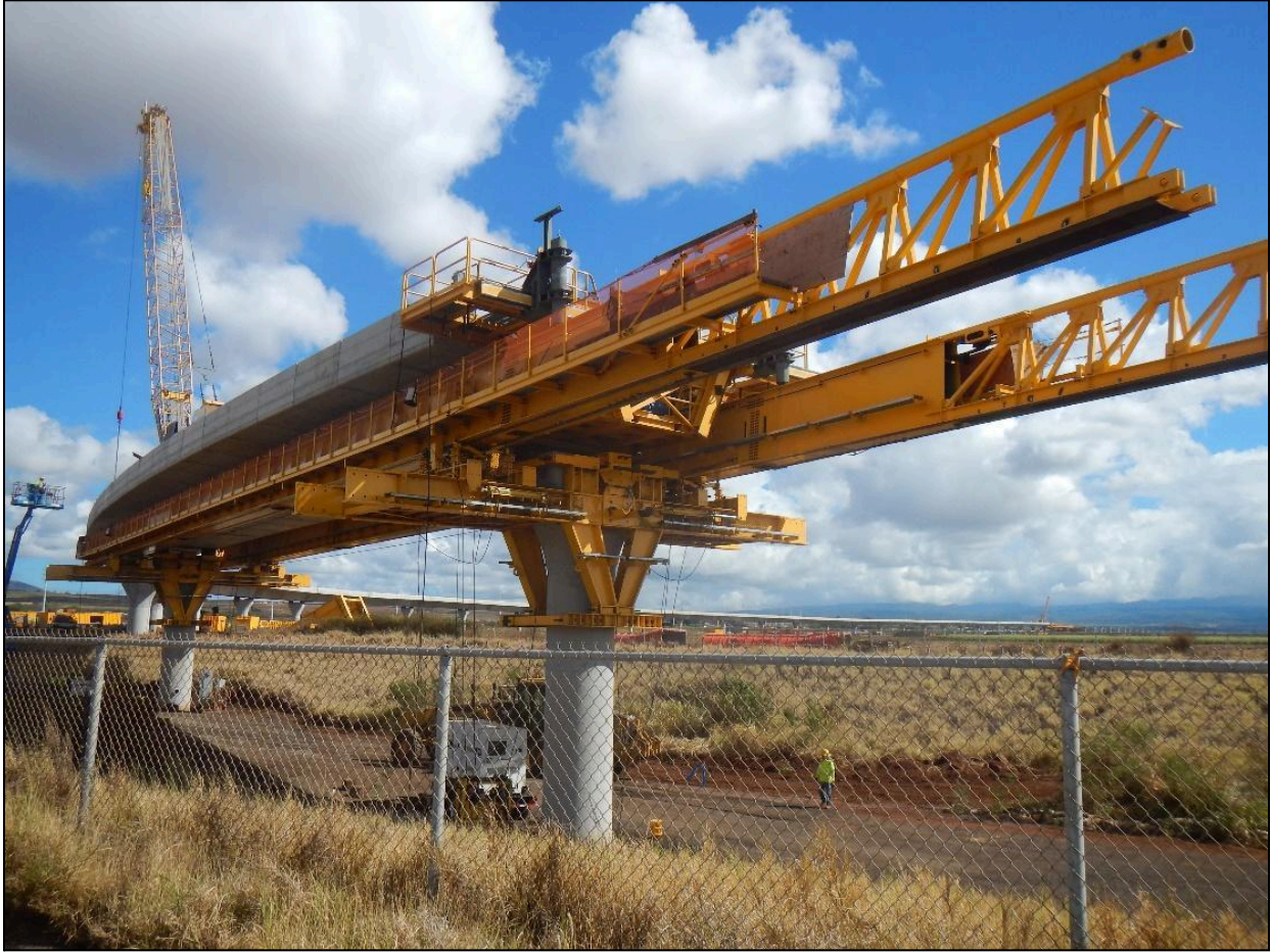
Figure 3.1 – Underslung Erection Truss, Honolulu Light Rail, HI (Photo Courtesy of FIGG)
