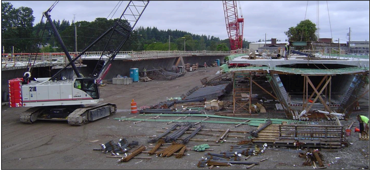
Figure 9.3 – Simple Long-Line Casting Yard in Operation, SW Line Bridge, WA (Photo Courtesy of Atkinson Construction)
