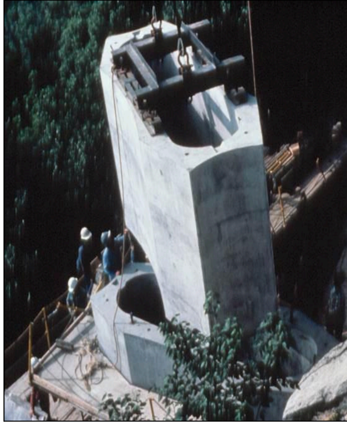
Figure 8.9 – Pier Column Segment Erection, Linn Cove Viaduct, NC (Photo Courtesy of FIGG)
