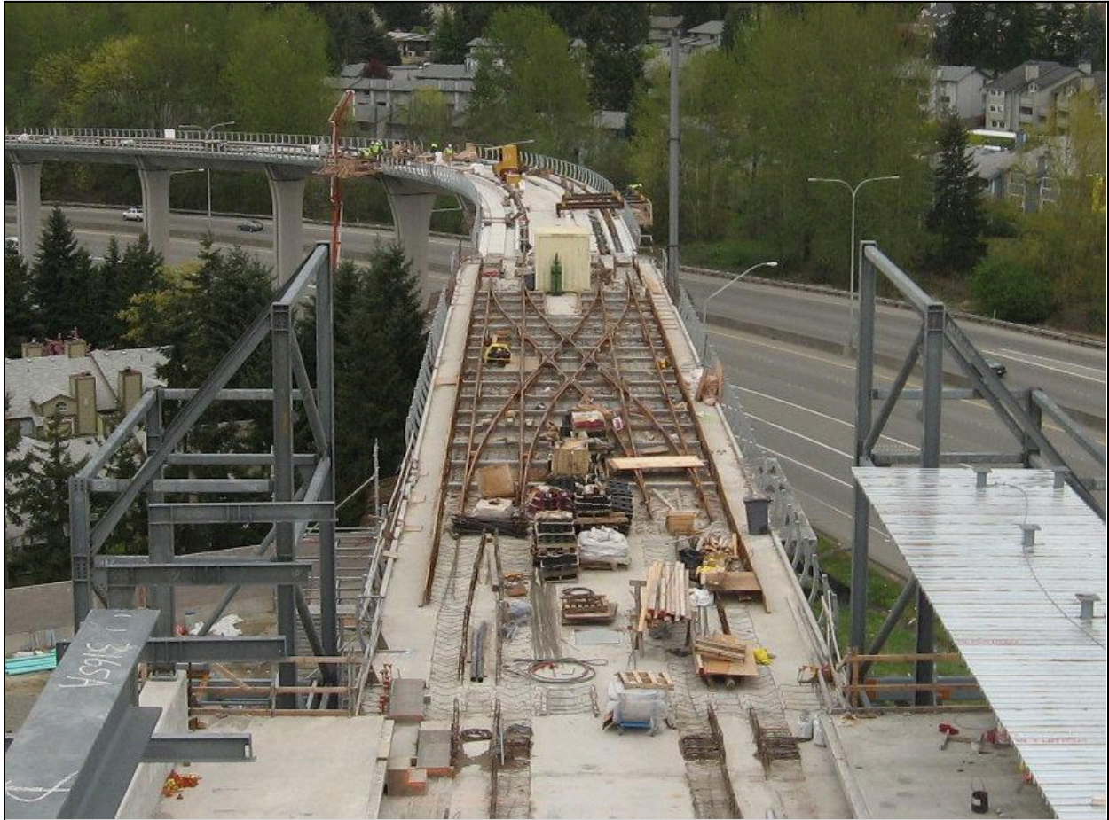
Figure 9.46 – Crossover Rail Layout Prior to Secondary Concrete Pour (Photo Courtesy of Fueled Photography/PCL Civil Constructors, Inc.)
