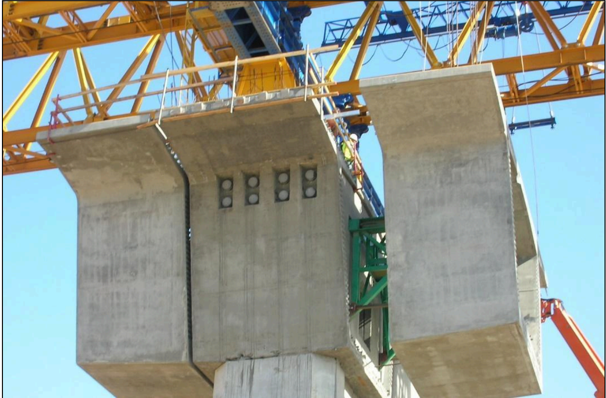
Figure 4.37 – First Precast Segment Supported Prior to Casting Closure Joint, Otay River Bridge, CA (Photo Courtesy of SYSTRA IBT)
