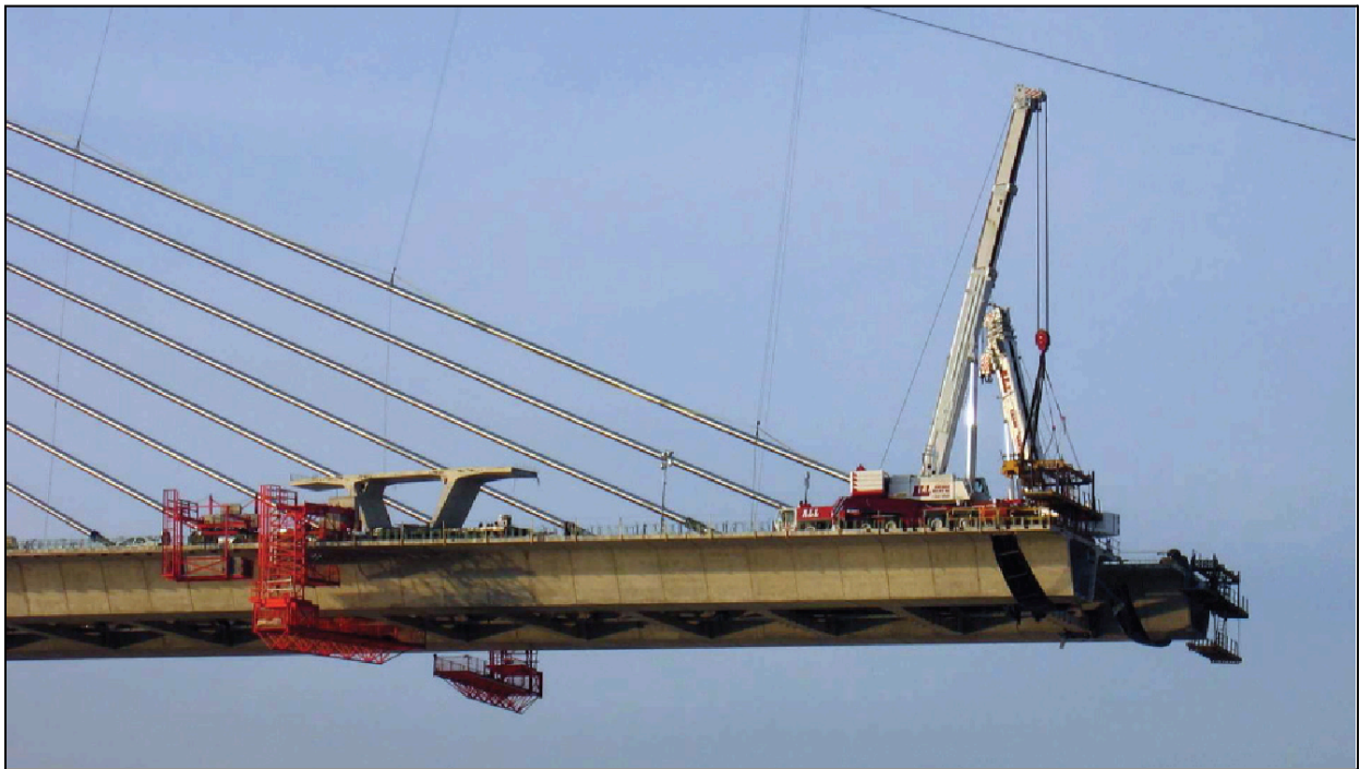
Figure 7.20 – Segments Delivered Over Deck, Veterans' Glass City Skyway, OH (Photo Courtesy of Bilfinger & Berger)
