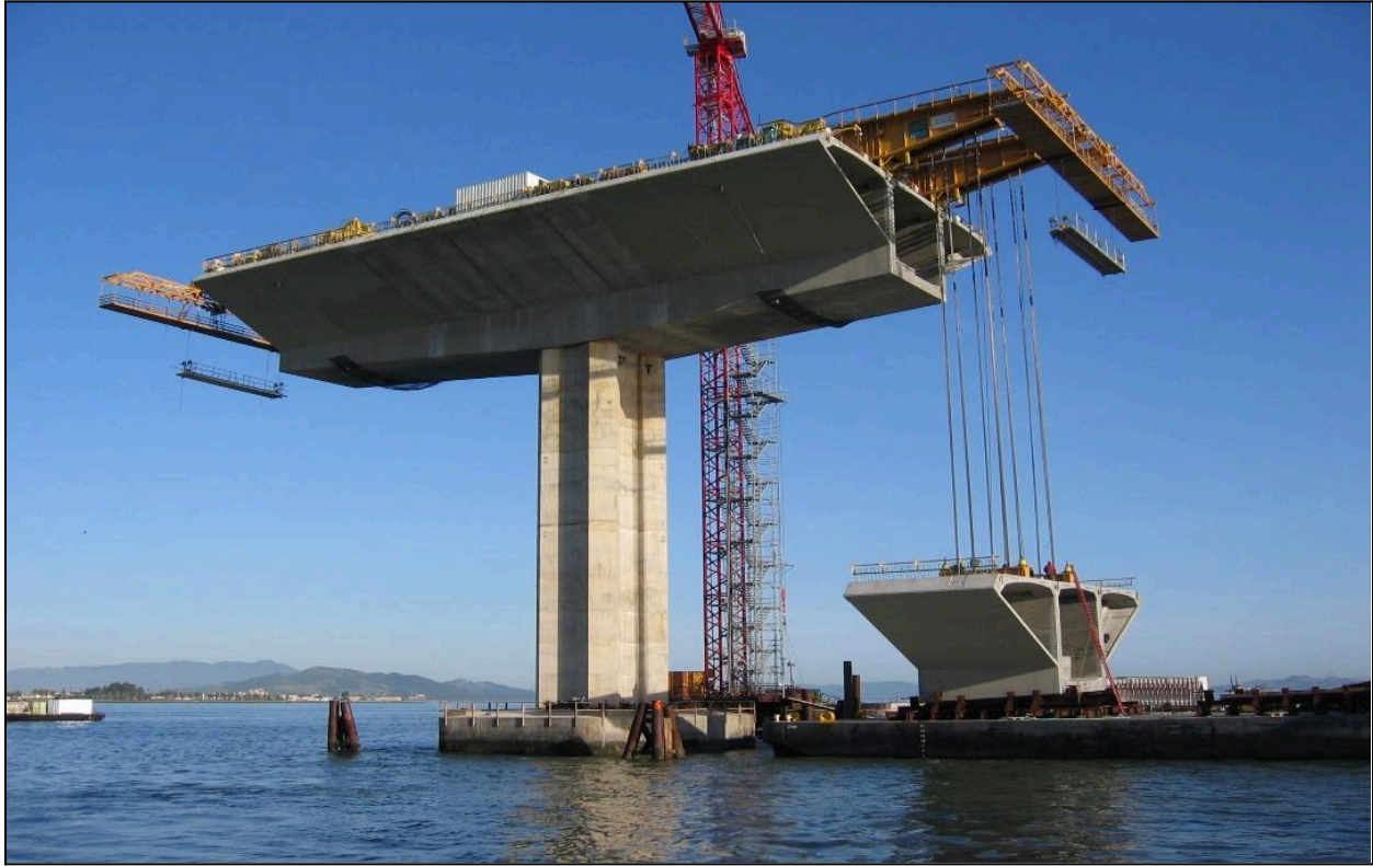
Figure 4.27 – Beam and Winch System, San Francisco-Oakland Bay Bridge, CA (Photo Courtesy of Flatiron Constructors, Inc.)
