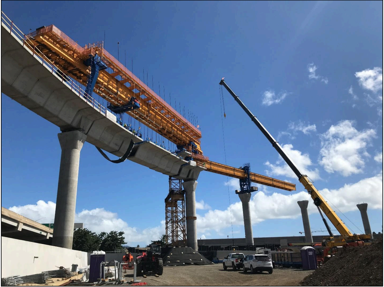
Figure 10.19 – Span-by-Span Articulating Gantry, Honolulu Light Rail, HI (Photo Courtesy of Traylor Bros., Inc.)
