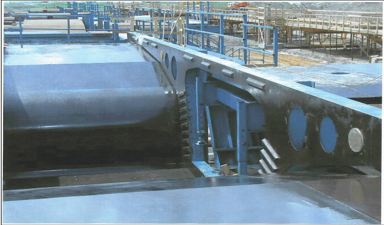
Figure 9.9 – Bulkhead and Wing Forms, Lee Roy Selmon Crosstown Expressway, FL (Photo Courtesy of FIGG)
