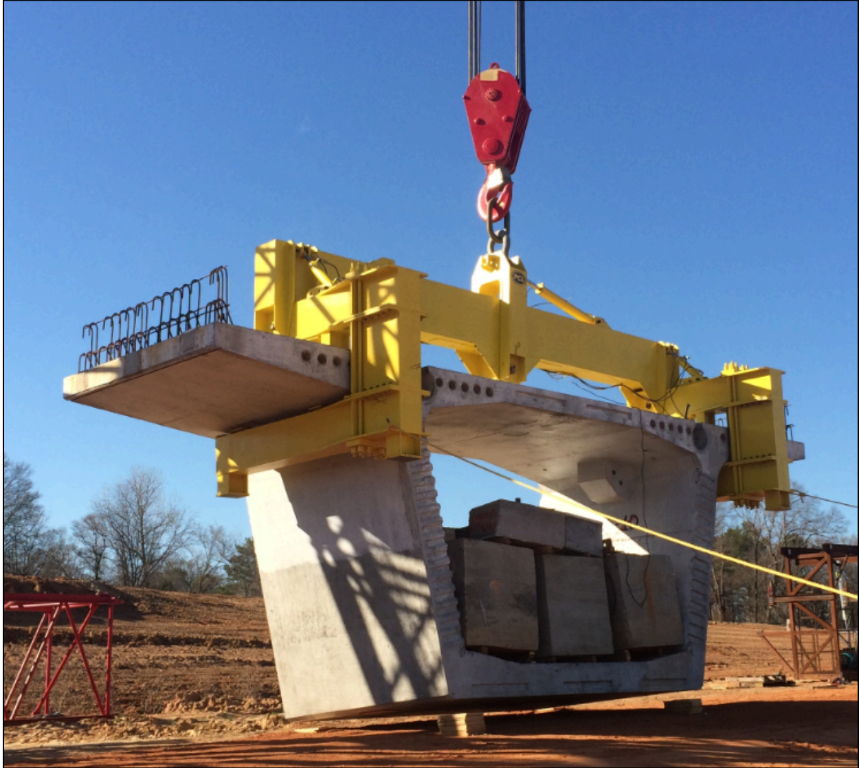
Figure 4.18 – C-Frame Lifting I-49 Bridge Segment K, LA (Photo Courtesy of PCL Civil Constructors, Inc.)
