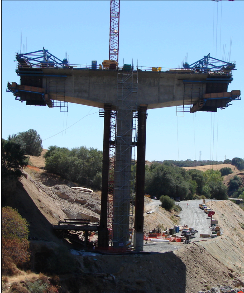
Figure 5.16 Temporary supports during construction, Folsom Dam Bridge, CA (Photo Courtesy of Kiewit)
