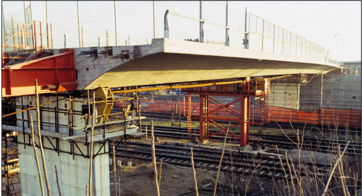
Figure 6.20 – Lateral Guide at the Permanent Pier (Photo Courtesy of Marco Rosignoli)
