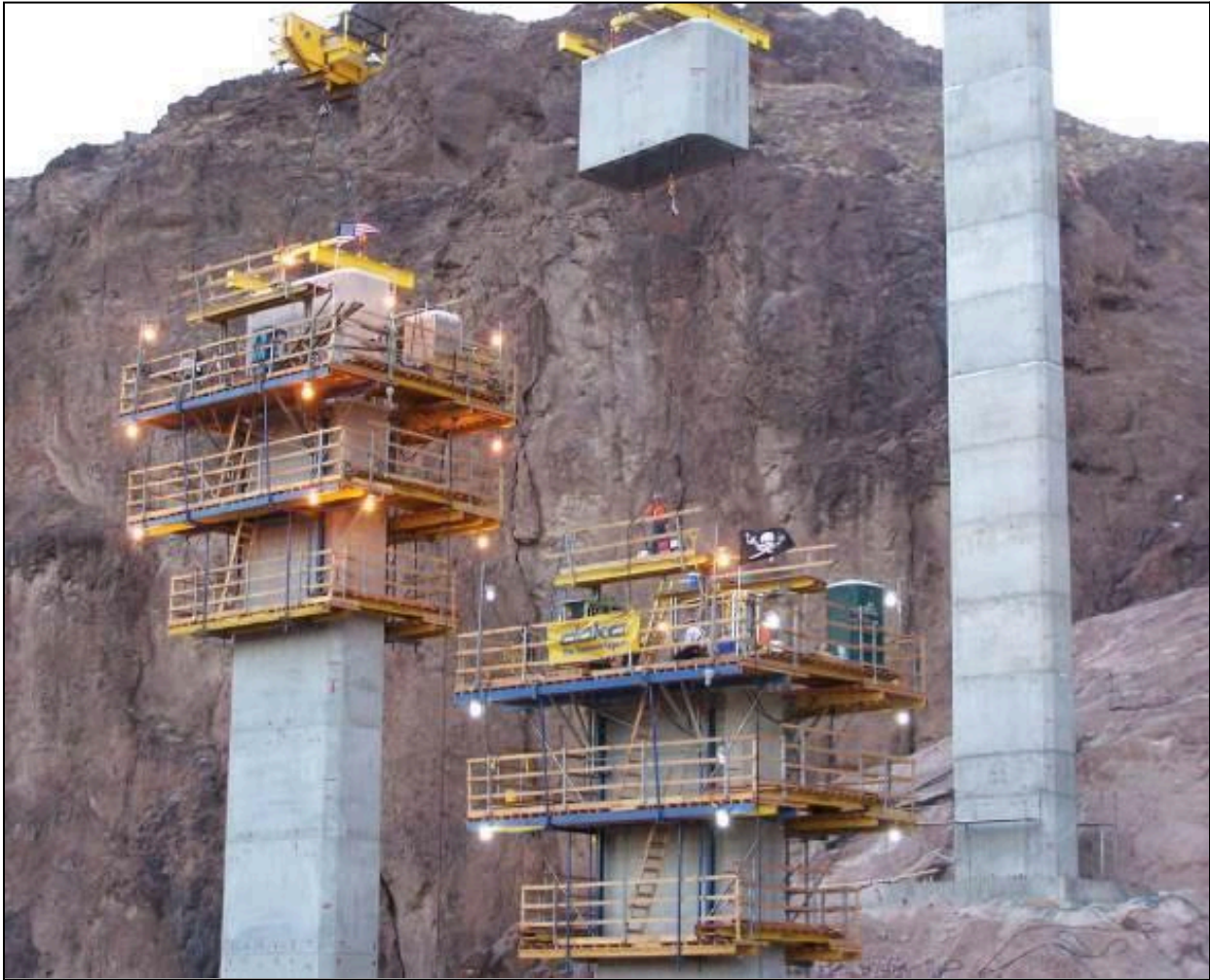
Figure 8.12 – Precast Column Erection, O’Callaghan-Tillman Memorial Bridge, AZ-NV (Photo Courtesy of Obayashi)
