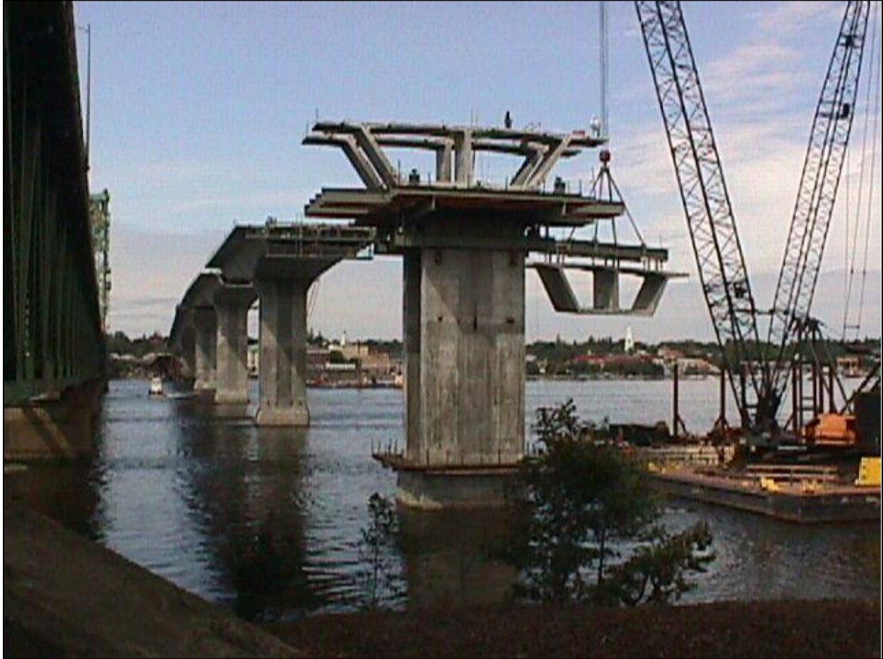
Figure 10.26 - Balanced-Cantilever Erection by Barge-Mounted Crane (Photo Courtesy of Flatiron Constructors, Inc.)
