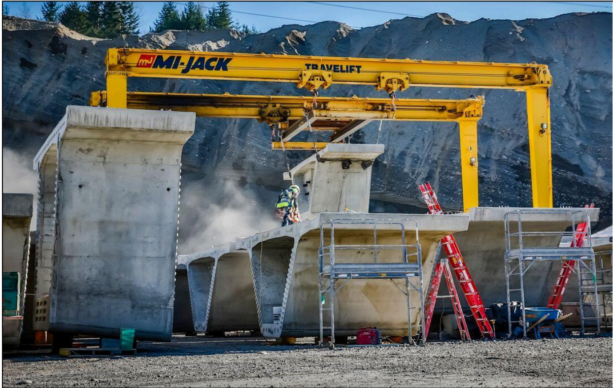
Figure 9.41 – Work Access for Finishing Segments (Photo Courtesy of Fueled Photography/PCL Civil Constructors, Inc.)
