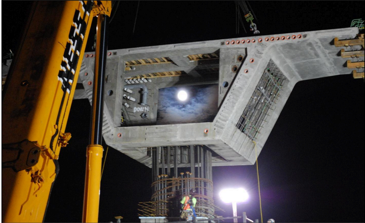
Figure 9.12 – Precast Pier Segment Shell Over Seismic Reinforcing [Note Voids for Placing Reinforcing and Concrete] (Photo Courtesy of Atkinson Construction)
