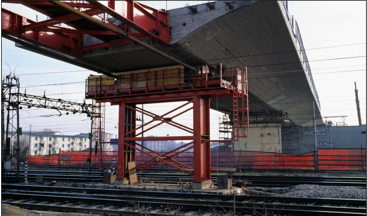
Figure 6.4 – Incremental Launching with Temporary Pier over Railway – Italy (Photo Courtesy of Marco Rosignoli)
