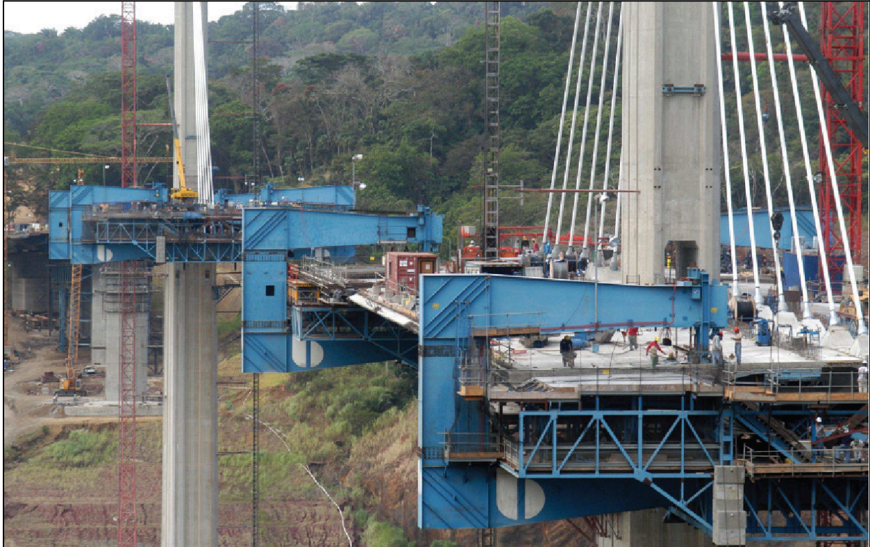
Figure 7.21 – CIP Box Girder with Traveler, Centennial Bridge, Panama (Photo Courtesy of Bilfinger & Berger)
