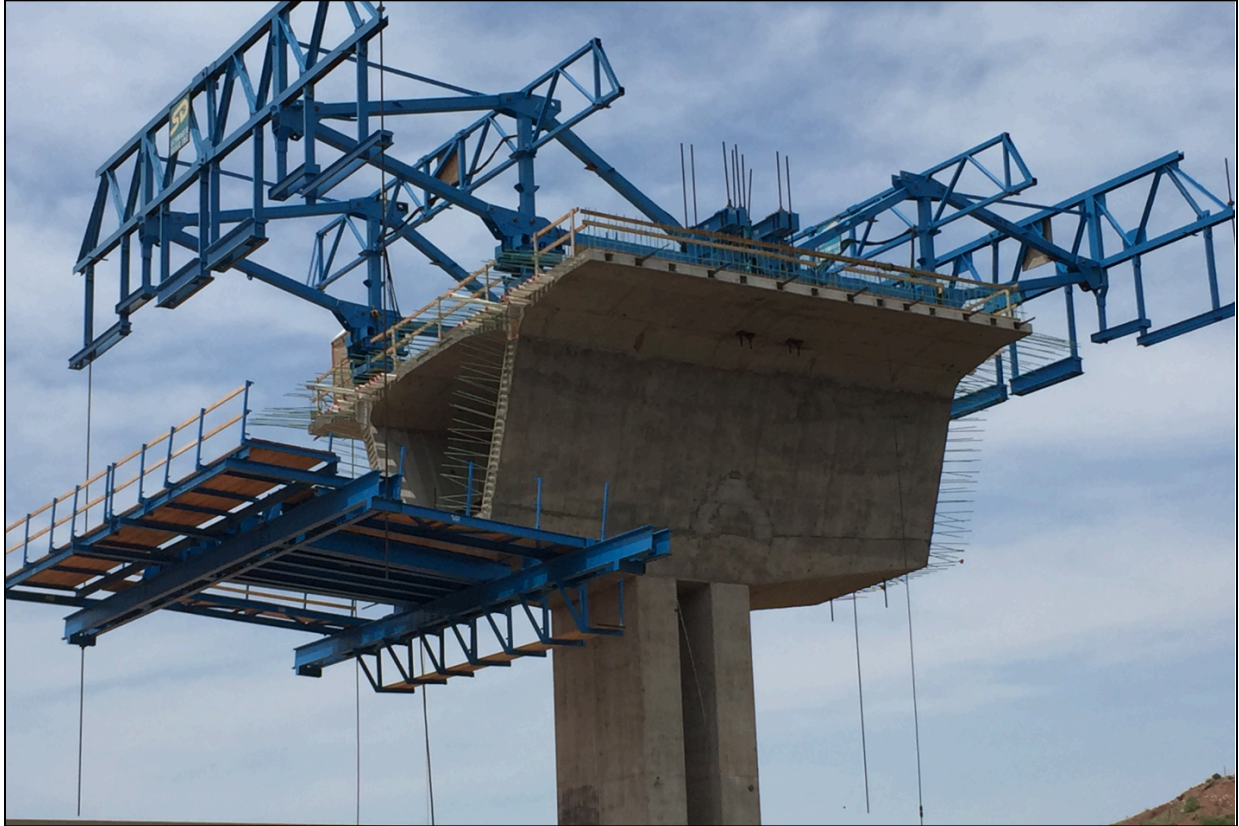
Figure 5.19 - Cast-in-Place Balanced Cantilever Bridge Design and Construction: Asymmetrical Pier Table, US 54 Canadian River Bridge, NM (Photo Courtesy of Krew Heavy Civil)
