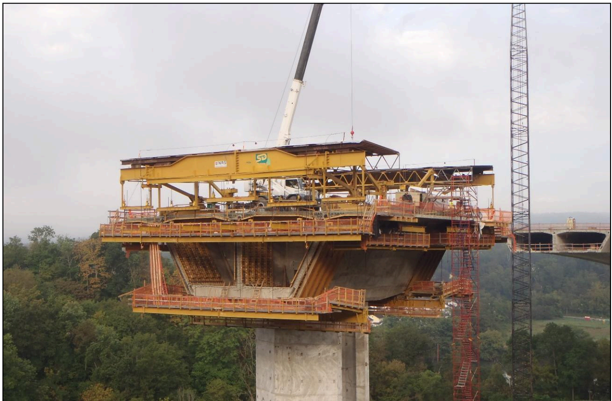
Figure 5.37 – End View of Form Traveler Work Platforms, Mon River Bridge, PA (Photo Courtesy of Walsh Construction)
