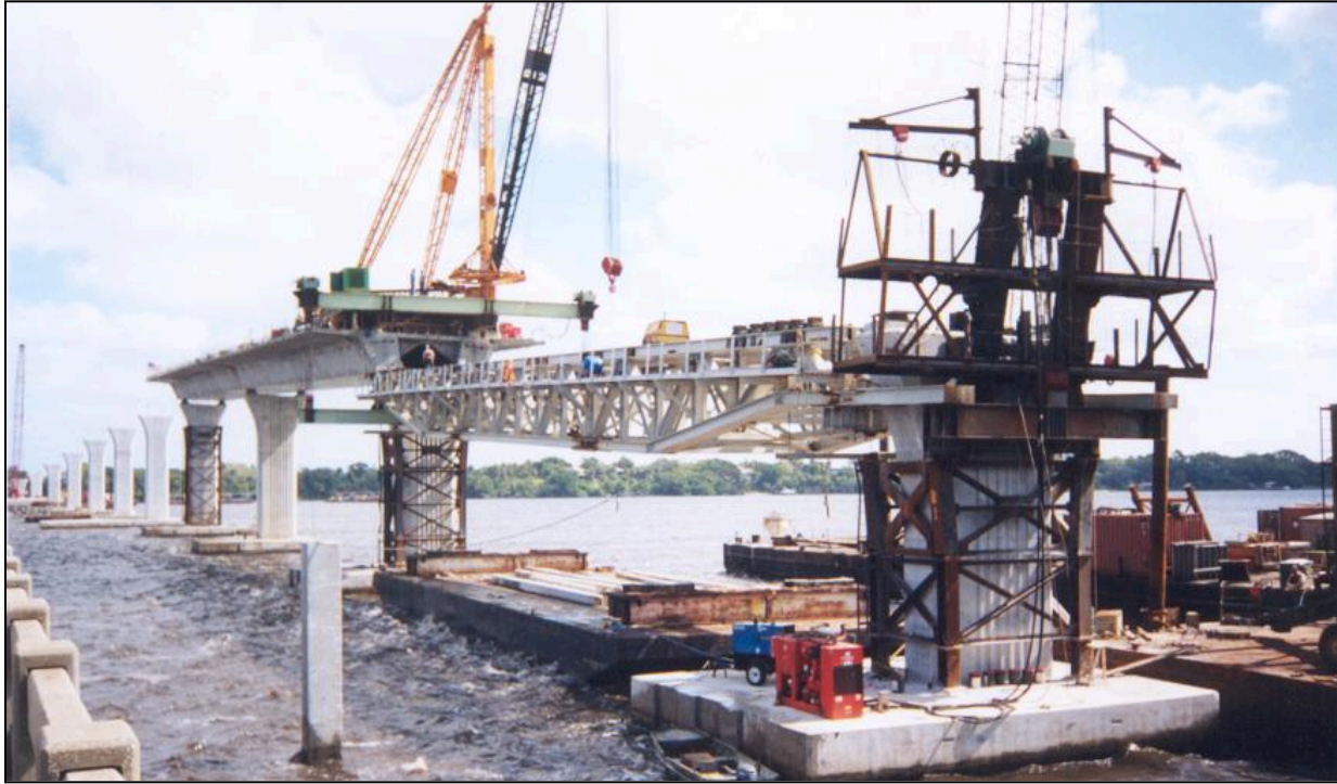
Figure 3.16 – Erecting Segments onto Trusses, Evans Crary Sr. Bridge, FL (Photo Courtesy of FIGG)
