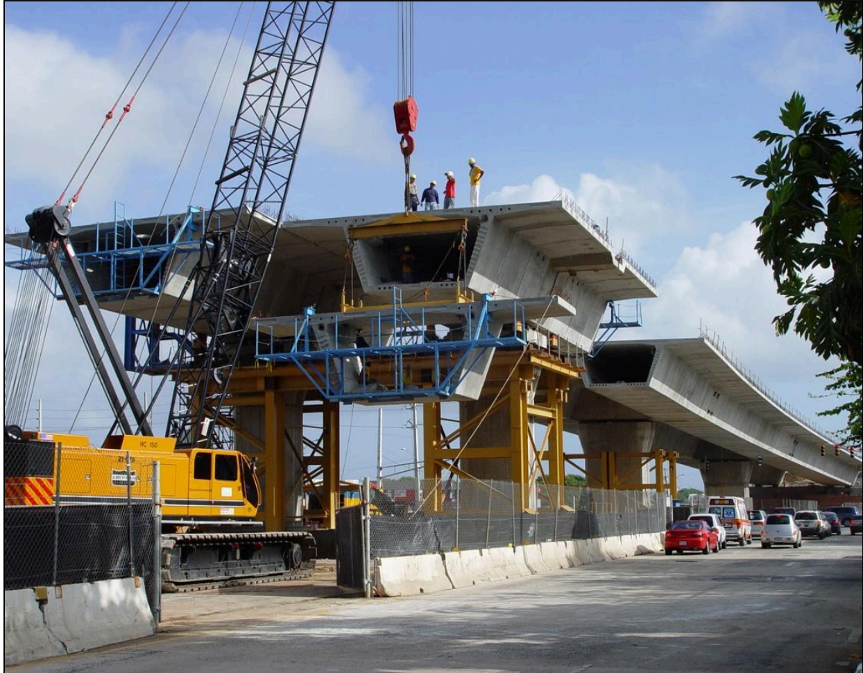
Figure 4.25 – Segment Erection by Crane on PR18 (Photo Courtesy of SYSTRA IBT)
