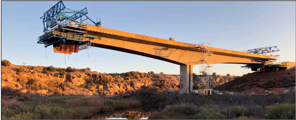
Figure 5.5 – Balanced Cantilever with End Spans on Falsework: US 54 Canadian River Bridge, NM (Photo Courtesy of Krew Heavy Civil)
