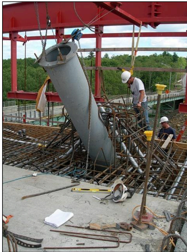
Figure 7.67 – Guide Pipe Being Positioned in Deck Formwork (Photo Courtesy of FIGG)
