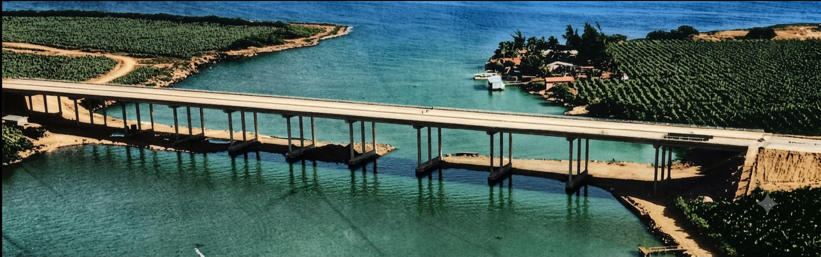
Mosquito River Bridge, Cuba – predecessor to Zaza Bridge
